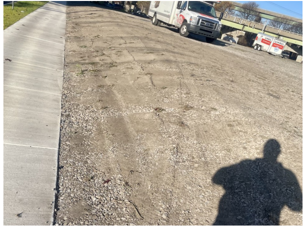
Photo of repairs to site cover and demarcation layer.
