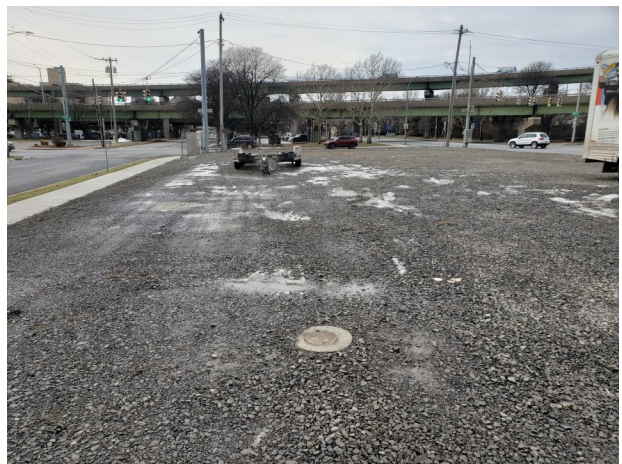
Photo of site cover system.
