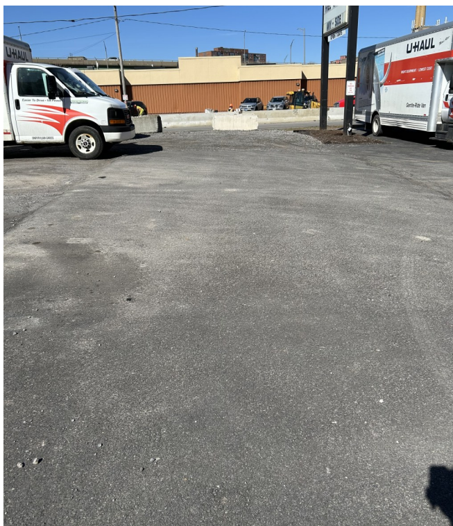
Photo of portion of gravel cover system that had been paved over to prevent gravel from tracking into other parking lot.
