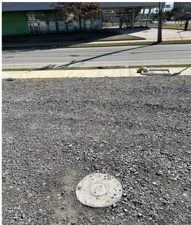
Photo of gravel cover system and monitoring well.
