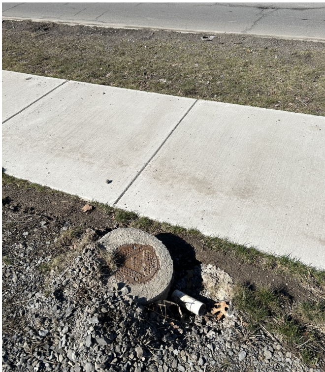
Photo of damaged monitoring well, MW-6.
