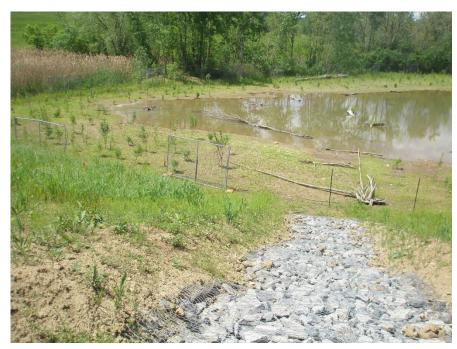
Constructed swale, with a gabion mattress, along the berm conveys surface flow to mitigation area.
