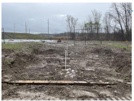
Spillway construction along the northern edge of the mitigation area.
