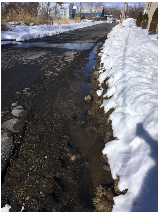
Photo 1 - View of isolated soil cover system damage near southwestern corner of building.
