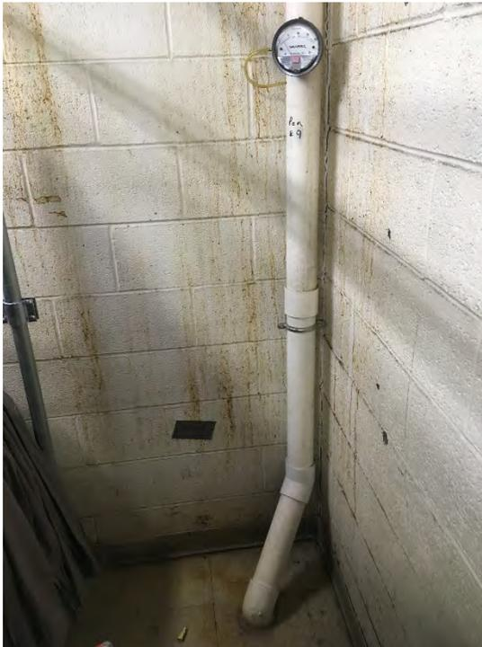
Photo 16 - View of typical SSDS suction point riser and magnehelic gauge.
