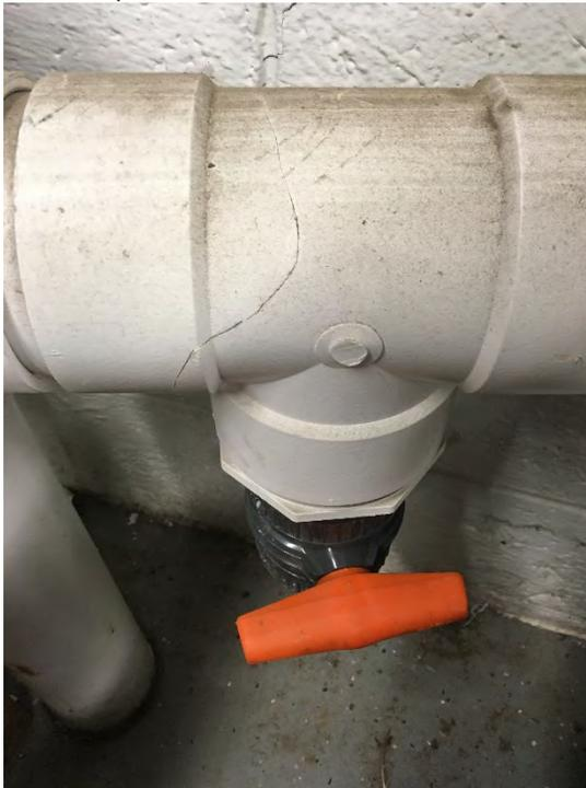
Photo 10 - The dislodged ball valve was able to be temporarily re-inserted until repairs can be arranged outside of this PRR's certification period.
