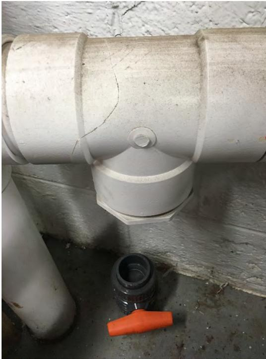
Photo 9 - View of broken "T" fitting and dislodged ball valve on SSDS suction riser S-14 leading to Fan 2. Repairs will be arranged outside of this PRR's certification period.
