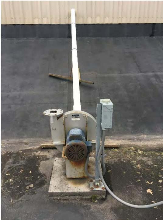
Photo 7 - View of Fan 1 pipe supports that need to be repaired. Temporary repairs were made by Box Capital on March 20, 2020 (outside of this PRR's certification period) until parts for permanent repair are available.
