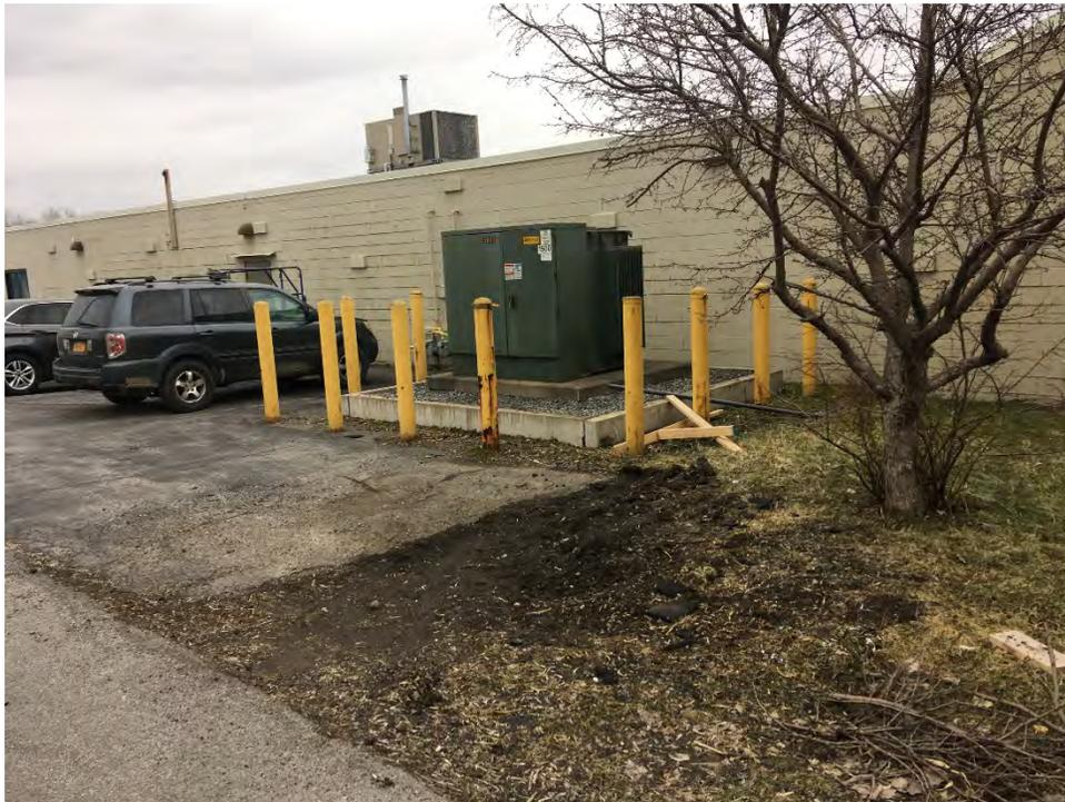
Photo 2 - View of minor soil cover system damage near northwestern portion of Site. Reportedly repaired by Box Capital by regrading on March 20, 2020
