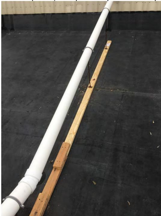
Photo 8 - View of Fan 1 pipe supports temporary repairs made by Box Capital on March 20, 2020 (outside of this PRR's certification period).
