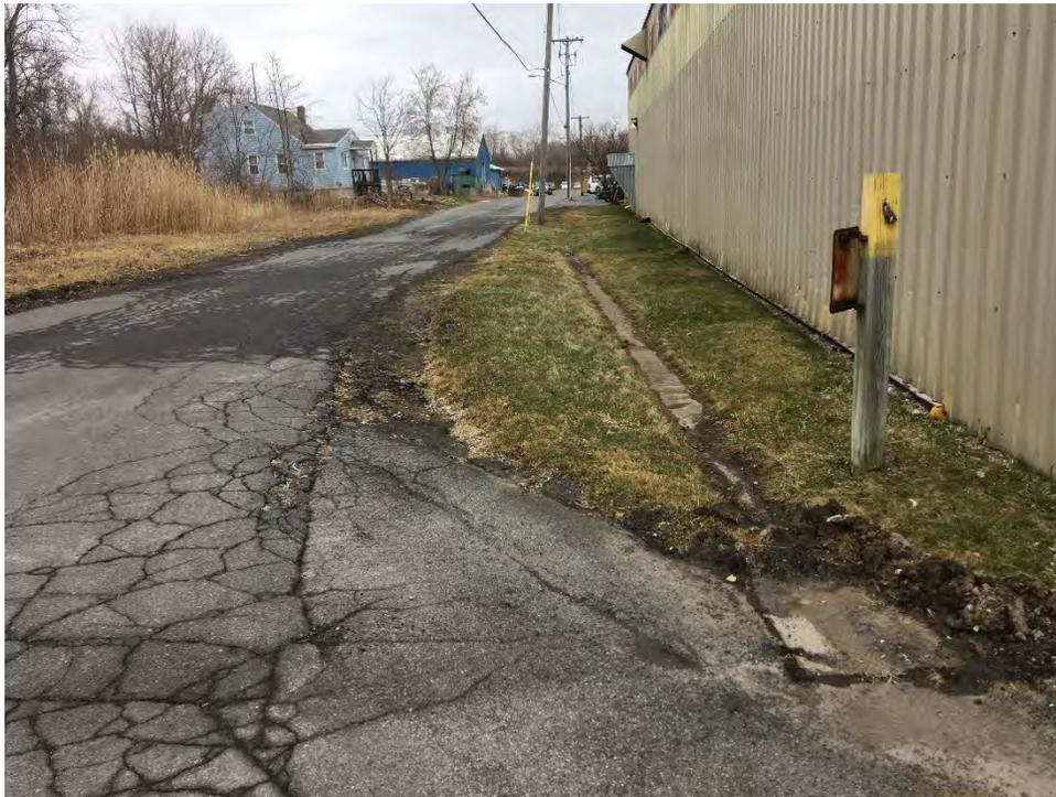
Photo 1 - View of minor soil cover system damage near southwestern corner of building. Reportedly repaired by Box Capital by regrading on March 20, 2020.
