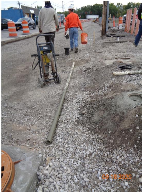
Photo 1 - The PVC well screen and riser was removed from exterior monitoring well location (MW-19) and the void was grouted.
