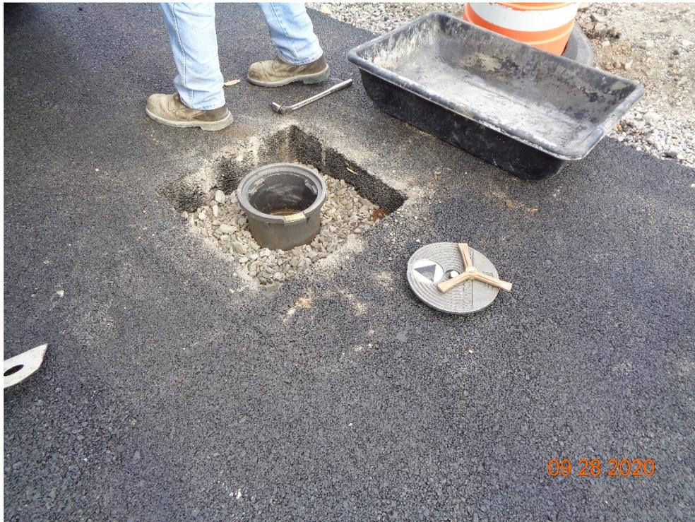
Photo 4 - New flush mount surface casing installed to bring monitoring well (MW-18) up to the newly developed asphalt grade.
