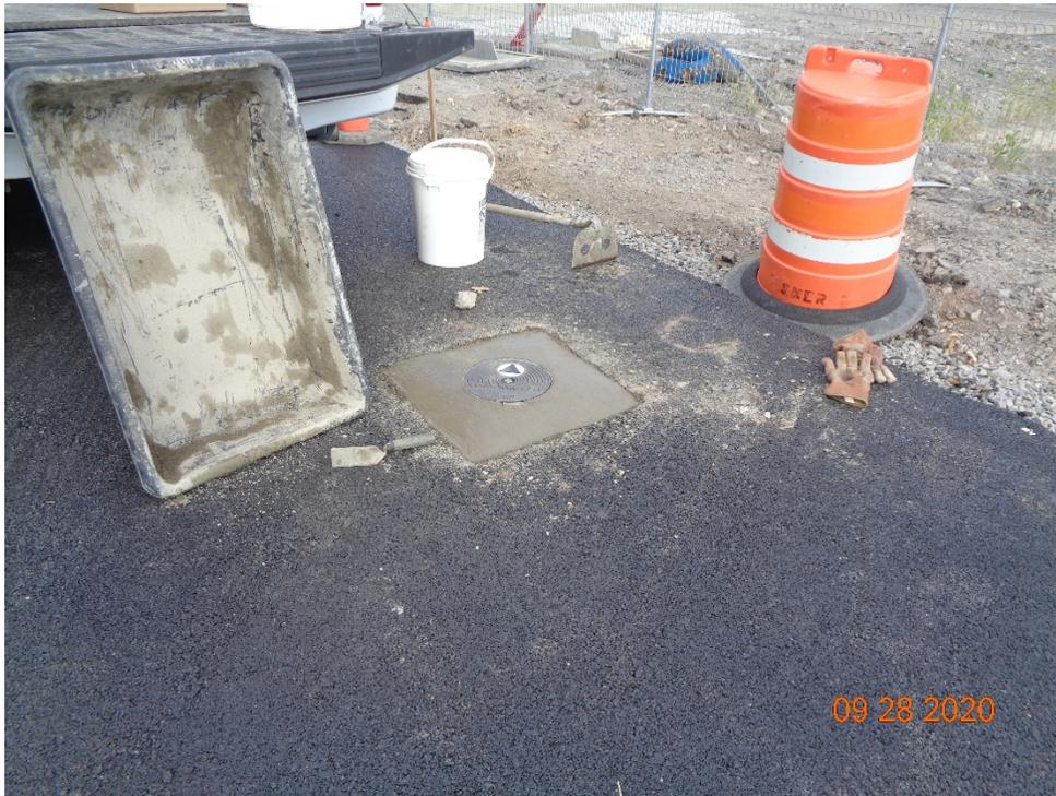
Photo 5 - Finished concrete pad and cover at MW-18 flush with surrounding grade.
