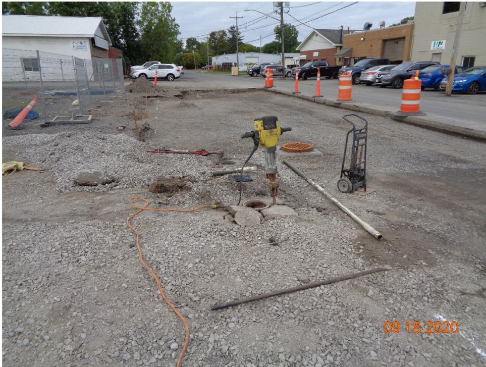
Photo 3 - The flush mount covers and associated concrete pads were removed.
