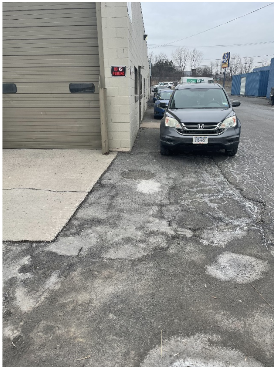
Photo 8 - View of northern portion of Site along Knapp Street.
