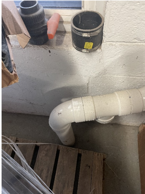
Photo 10 - View of repaired "T" fitting on SSDS suction riser S-14, leading to Fan 2. Recommended repairs were completed by Box Capital in April 2020.
