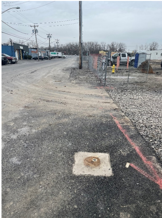
Photo 15 - View of repaired MW-18, off-site in the Luther Avenue right-of-way.
