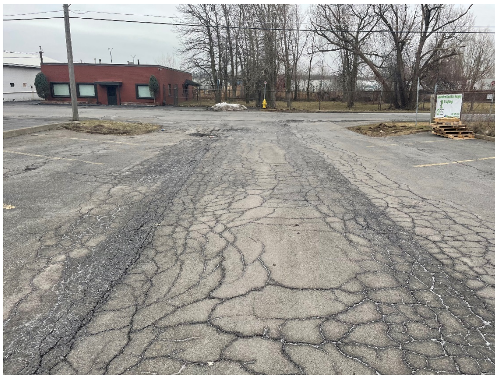
Photo 5 - View of southern portion of Site.
