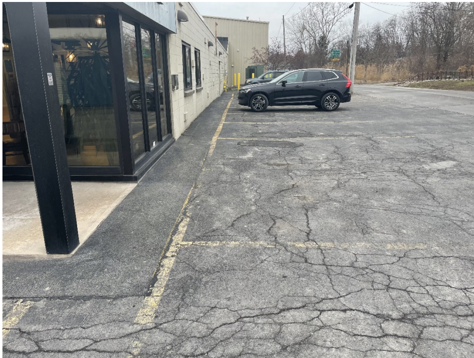
Photo 3 - View of northern portion of Site from Knapp Street and Albion Avenue intersection.
