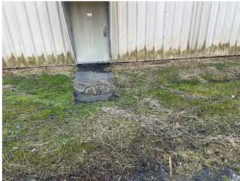
Photo 2 View looking at access door to facility along northwestern wall.
