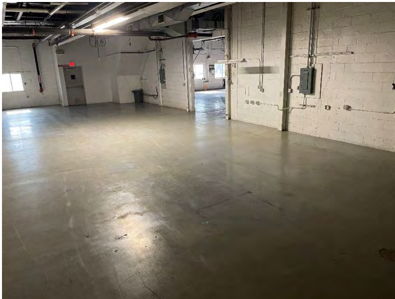
Photo 8 Interior portion of building formerly occupied by UniFirst (currently vacant).
