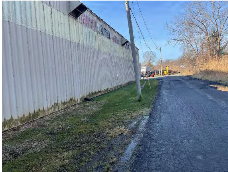
Photo 1 View looking southwest of grass and pavement areas located at northwest side of building.
