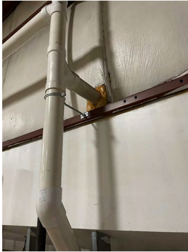
Photo 5 Typical view of riser wall penetration to exterior roof mounted fan.
