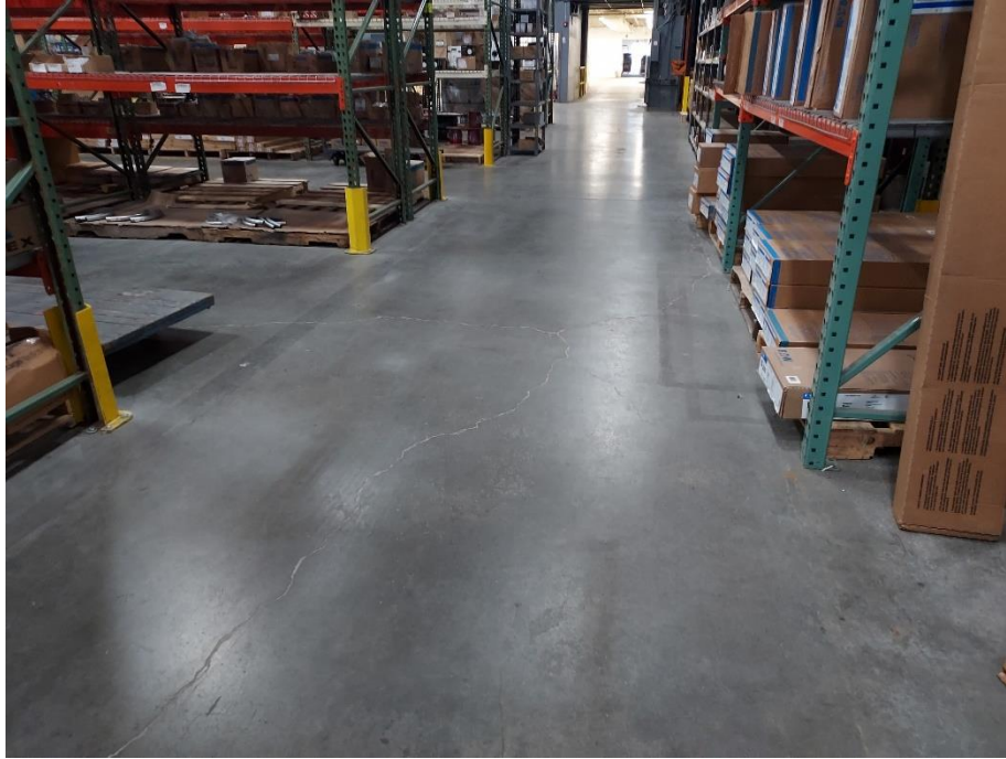
Photo 5 View of warehouse space showing previously sealed cracks still in good condition.
