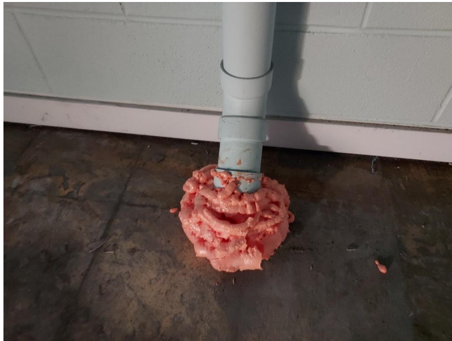
Photo 2 View of spray foam around floor penetration of suction riser S-6, no air leak noted.
