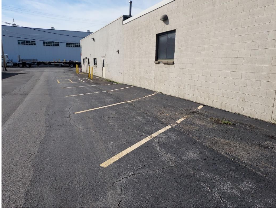
Photo 13 View of eastern asphalt pavement area in generally good condition.
