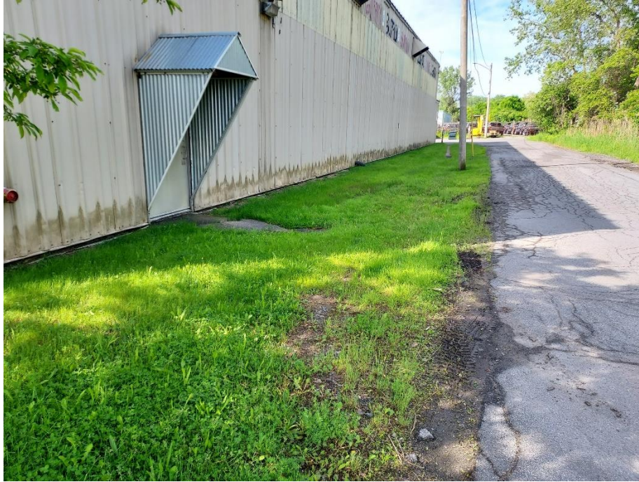
Photo 11 View of stabilized vegetation area along northern side of Site.
