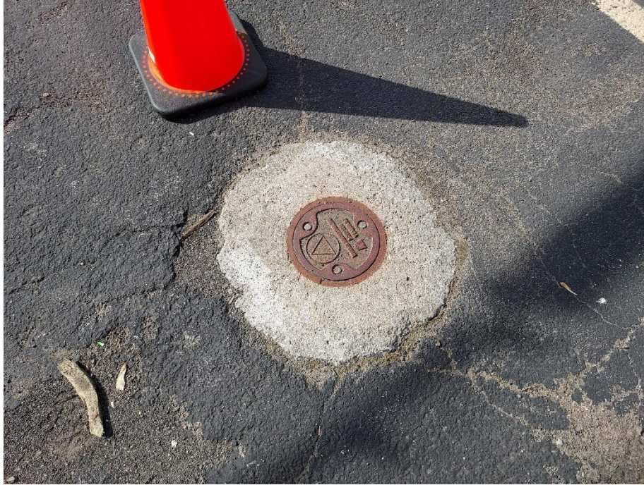
Photo 15 View of typical flush mount groundwater monitoring well along Luther Avenue side of Site.
