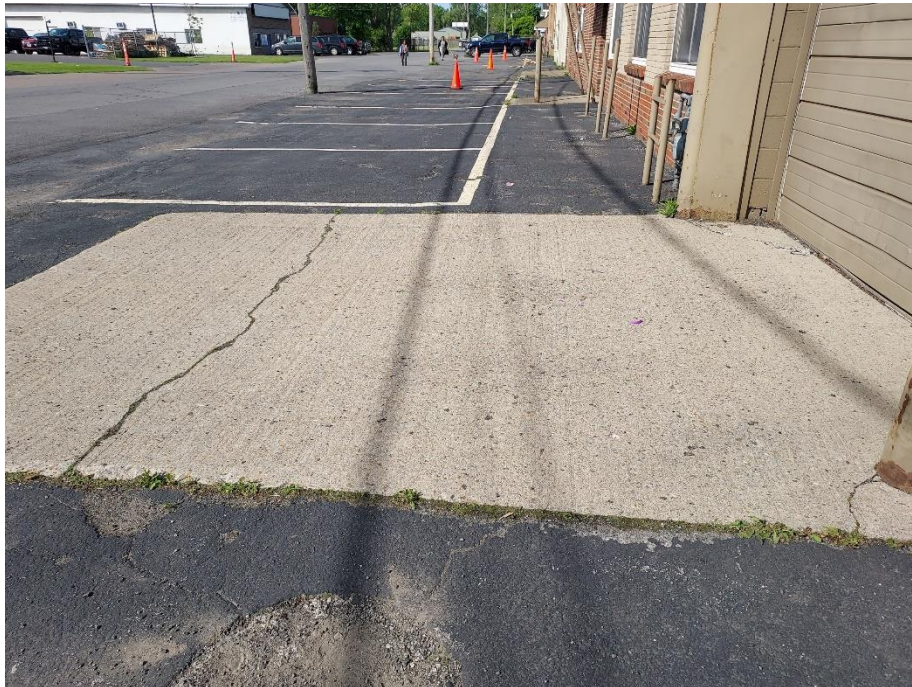
Photo 14 View of southern asphalt pavement area in generally good condition.
