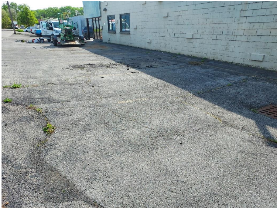
Photo 12 View of northern asphalt pavement area in generally good condition.
