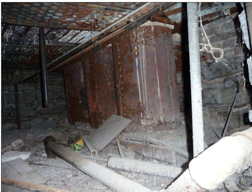
Crawl space with suspected UST fill pipe.
