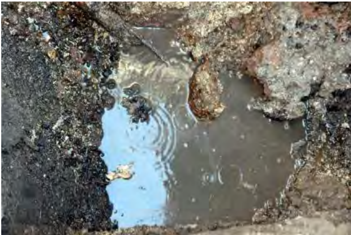
Buried fill, discolored water in excavation behind former mfg. area, northeast side of building.
