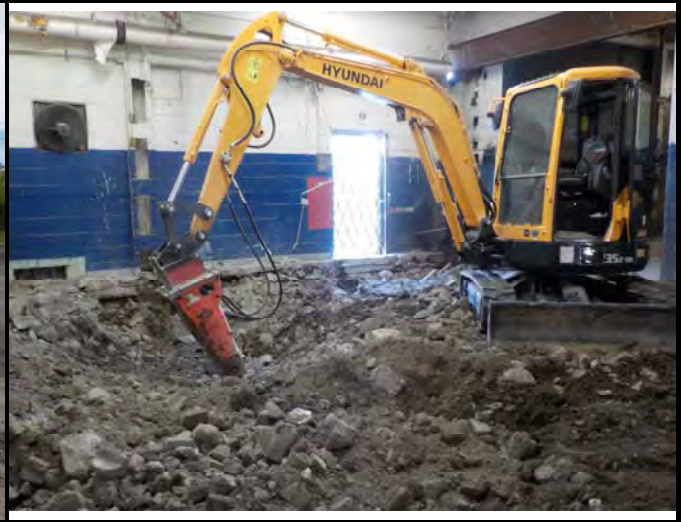
Photograph 4. Contractors utilizing a jackhammer attachment to break up concrete within the excavation.
