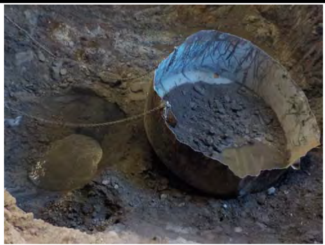
Photograph 26. Removing the second tank.
