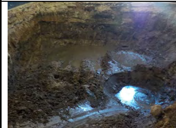
Photograph 27. The excavation area, post tank removal.
