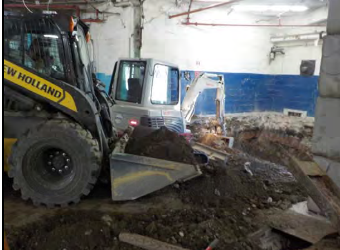
Photograph 10. Contractors using a mini excavator to load the bucket of a skid steer.
