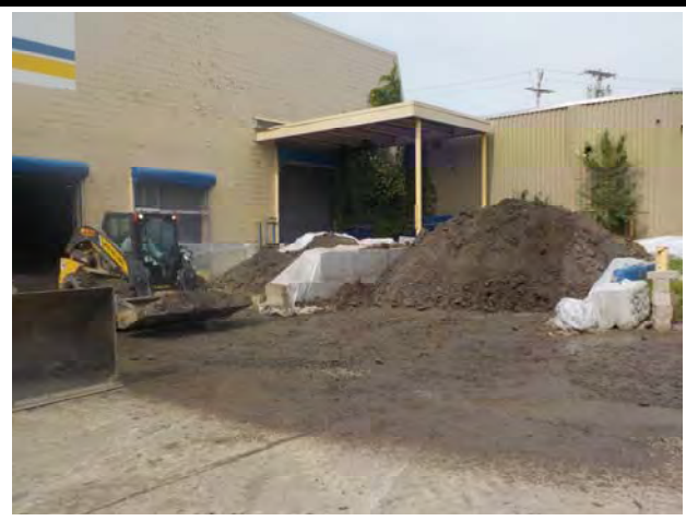
Photograph 20. Skid steer transporting material from the excavation area to stockpiles.
