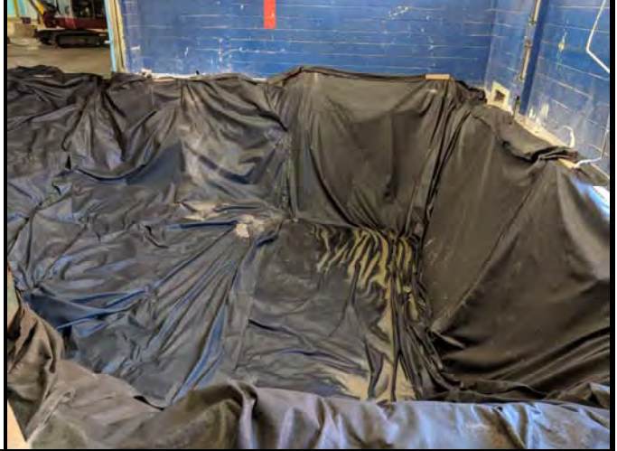
Photograph 32. Contractor lined the excavation with 8 ounce nonwoven geotextile material.
