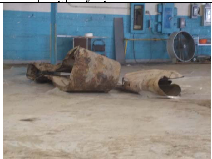
Photograph 15. Contractors cut the tank into sections to facilitate removal.
