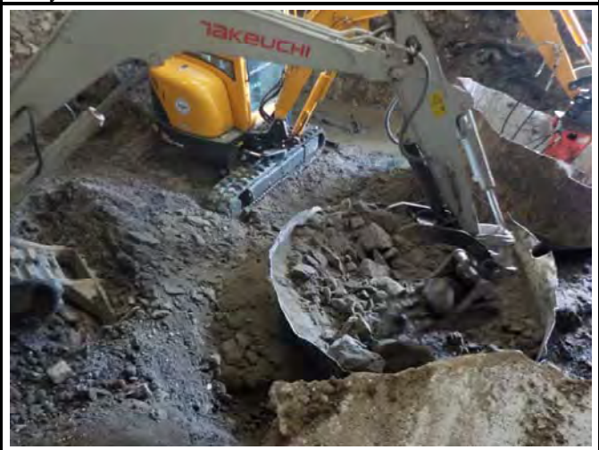
Photograph 24. Contractors using an excavator to remove cementitious material from the tanks.
