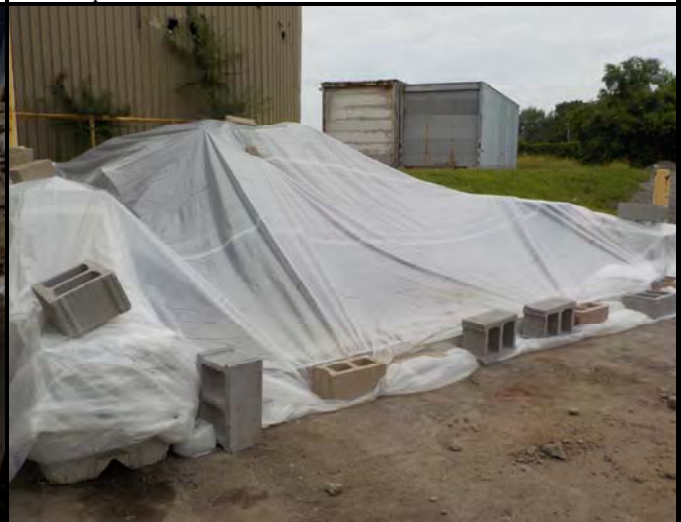
Photograph 6. Stockpiled material was covered with polyethylene sheeting at the end of each day.
