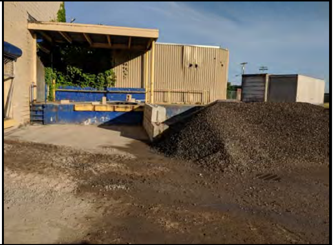
Photograph 34. Stockpile of #2 run of crush stone used to backfill the excavation.
