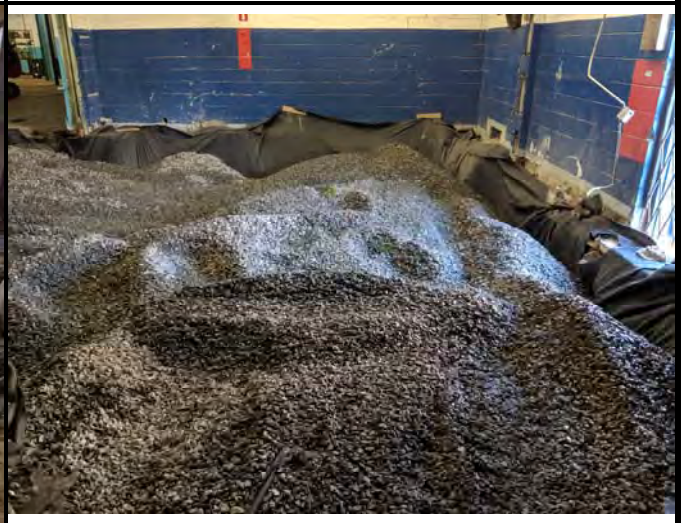
Photograph 36. Excavation backfilled with #2 run of crush stone.
