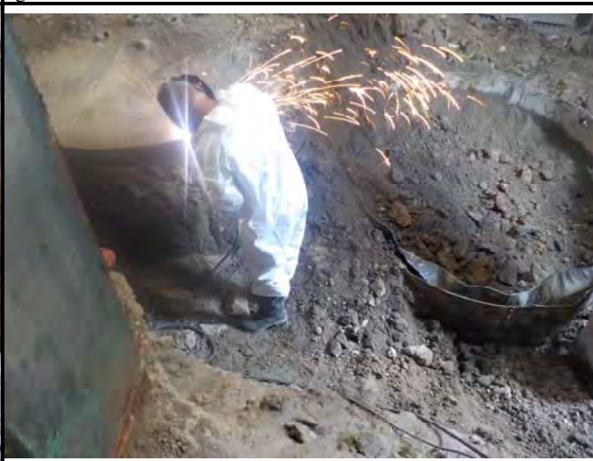
Photograph 18. Contractor utilizing an acetylene torch to cut the top off the tank.
