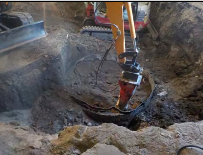
Photograph 17. Contractors using a jackhammer attachment to break up cementitious material within the tanks.
