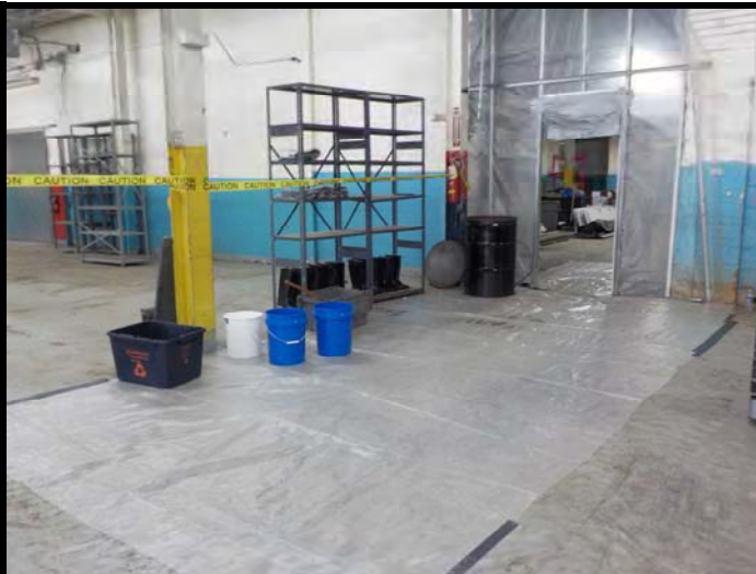
Photograph 1. Decontamination area and additional supplies for the contractors working within the Exclusion Zone.
