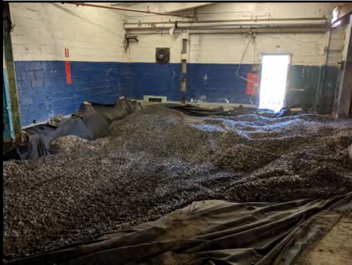
Photograph 35. Excavation backfilled with #2 run of crush stone.
