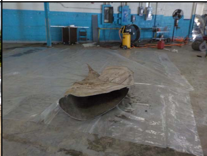
Photograph 12. Contractors cut off the top of a tank to remove the contents of the tank separately.
