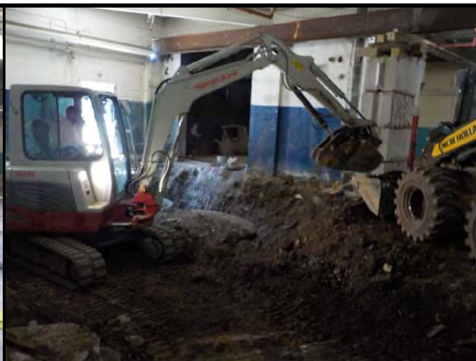
Photograph 8. Contractors using a mini excavator to load the bucket of a skid steer.
