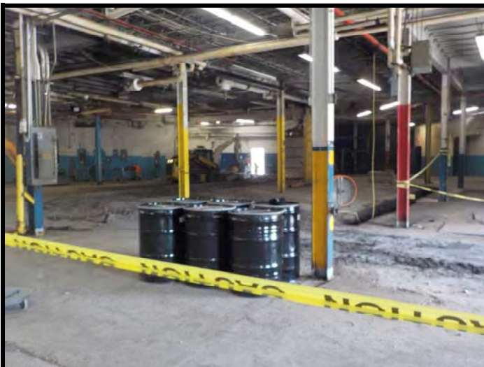
Photograph 7. Overall image of the warehouse.
