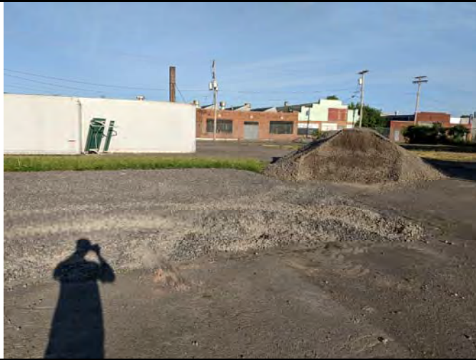
Photograph 33. Stockpile of #2 run of crush stone used to backfill the excavation.
