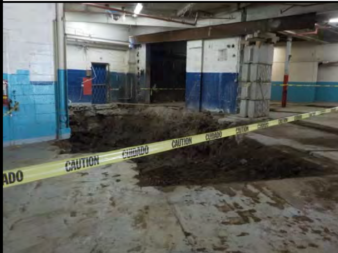
Photograph 29. Excavation taped off at the the end of UST and contaminated soil removal.
