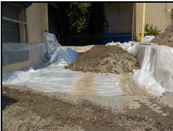
Photograph 13. Stockpiled the cementitious material from within the tanks separately, pending analytical results.
