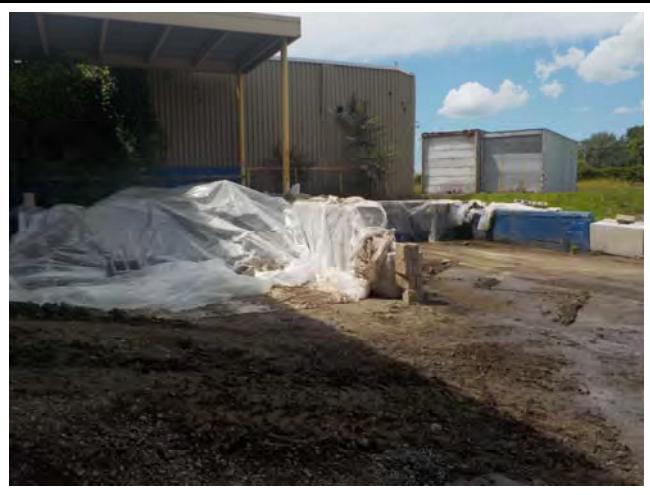
Photograph 22. Cementitious material covered, pending analytical results.
