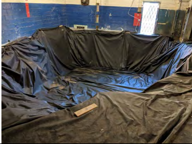
Photograph 31. Contractor lined the excavation with 8 ounce nonwoven geotextile material.
