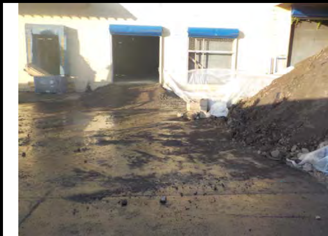
Photograph 19. Contractors wet the haul roads to minimize dust.
