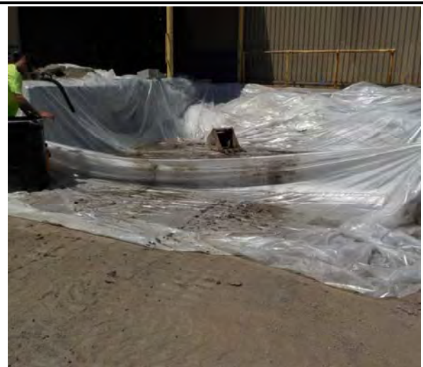
Photograph 30. Contractor decontaminating equipment.
