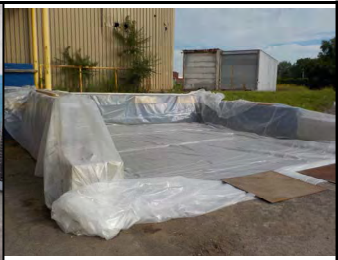
Photograph 2. Polyethylene lined stockpiling area adjacent to the loading docks and to the north of the building.
