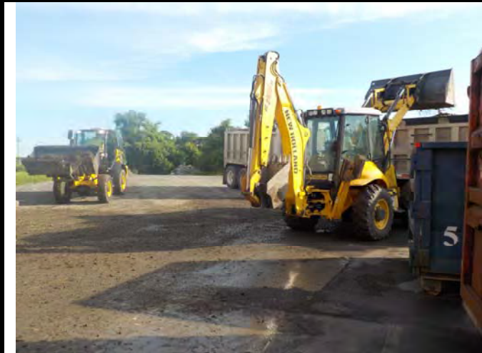
Photograph 21. Contractors loading the trucks with soil for off-site disposal.
