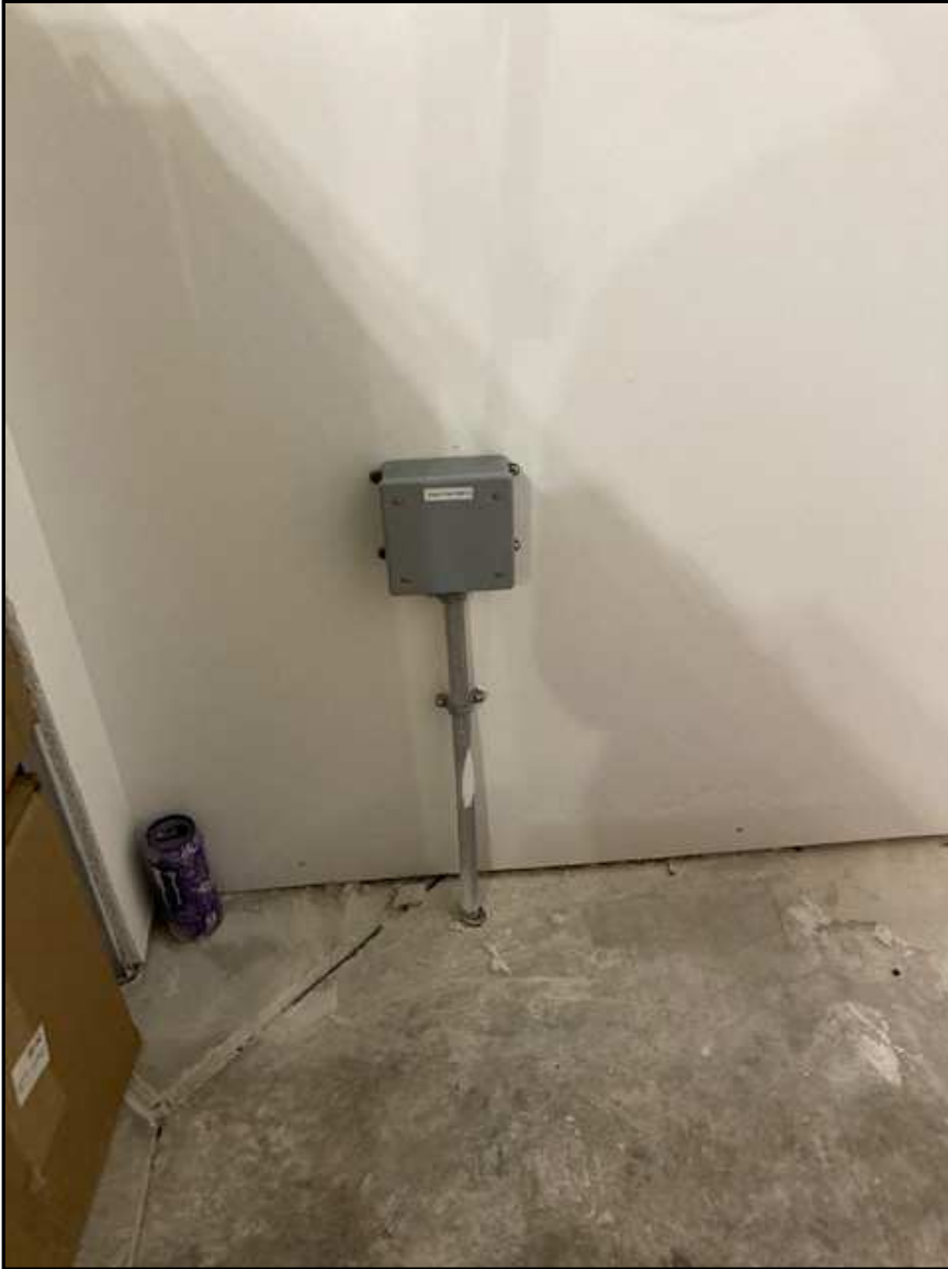
Pressure monitoring port in enclosure (typical).
