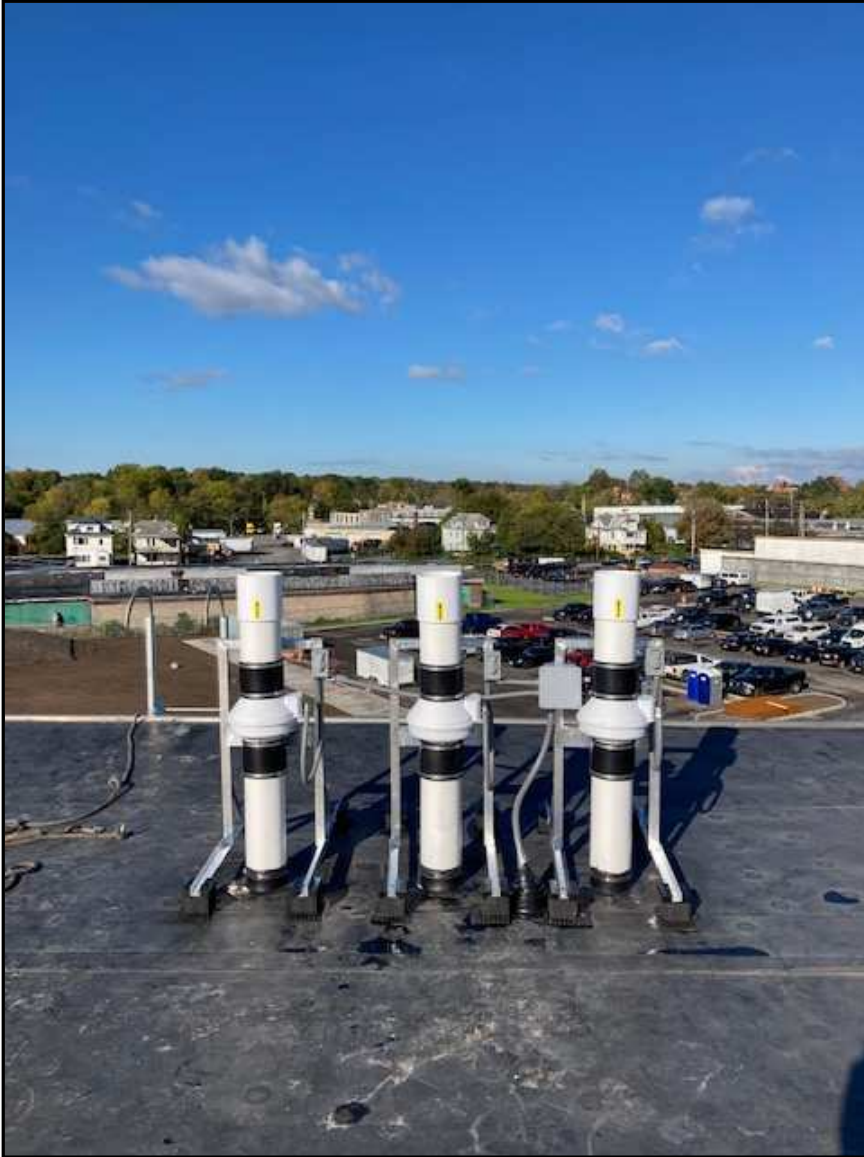
Fans F-3, F-4, and F-5 located on the roof. Electrical disconnect located adjacent to each fan.
