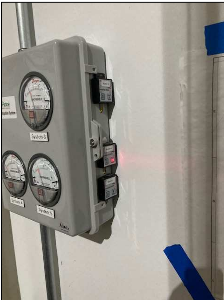
Low pressure alarms located on the side of the monitoring panel.
