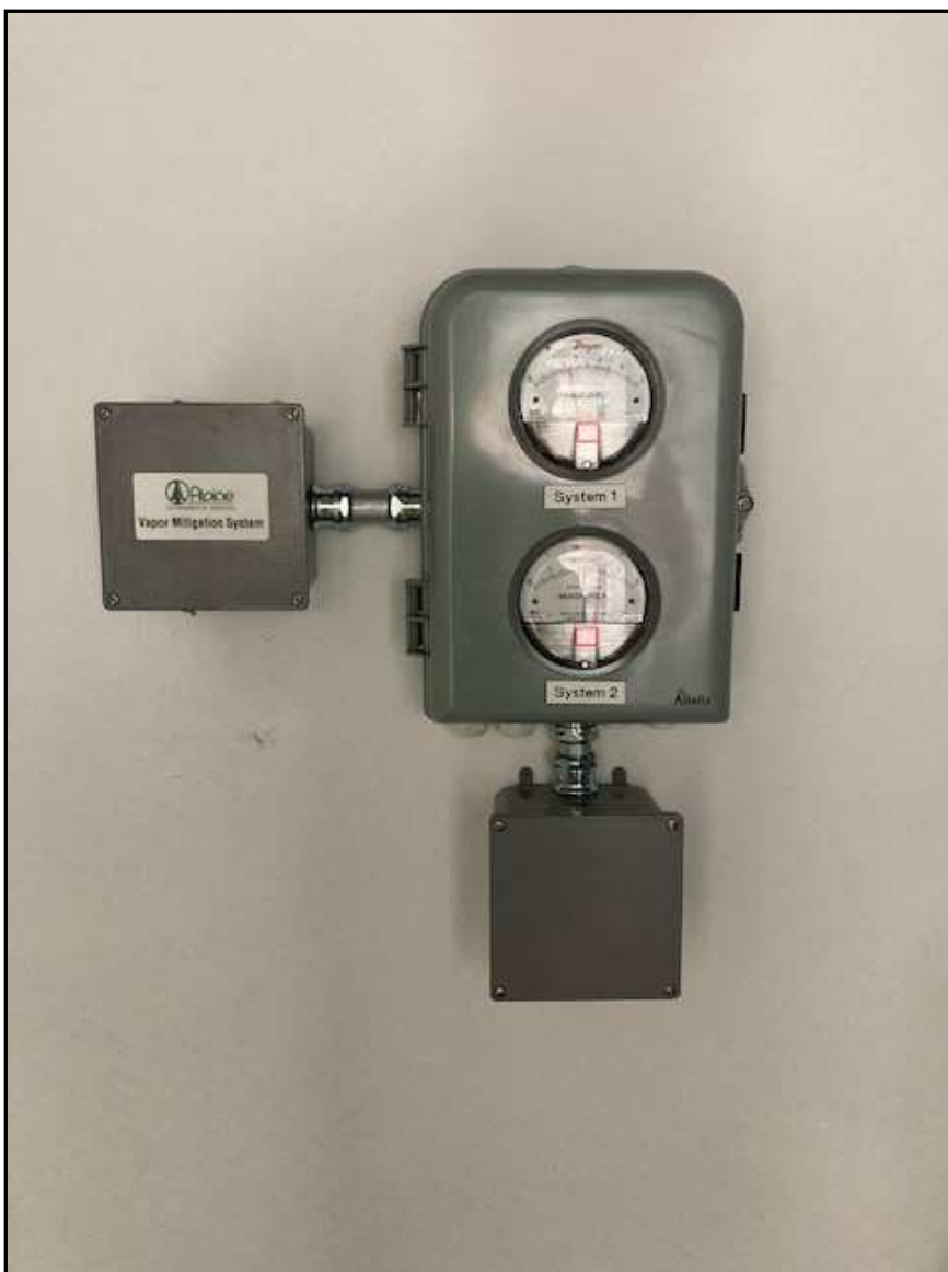
Monitoring panel for systems 1 and 2. Pressure gauges visible, low pressure alarms located on the side of the monitoring panel.
