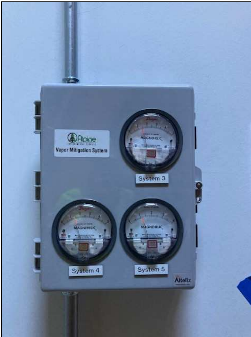
Monitoring panel for systems 3, 4, and 5. Pressure gauges visible, low pressure alarms located on the side of the monitoring panel.
