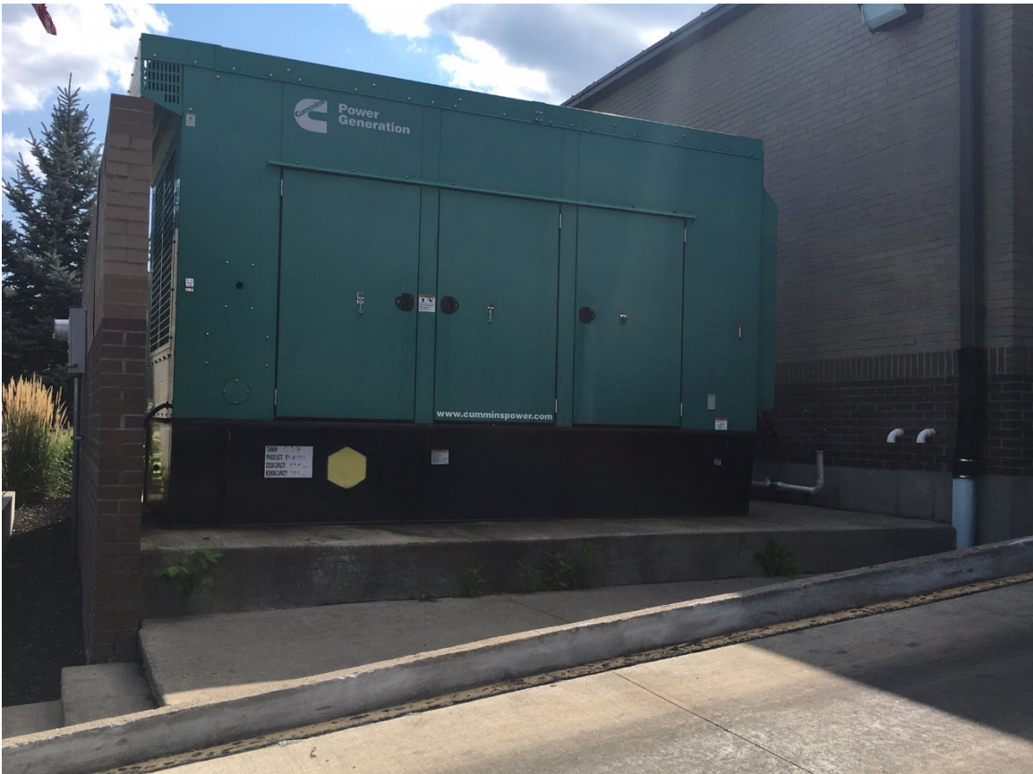
Backup diesel generator
