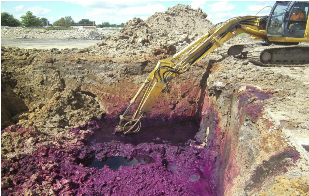
Figure 2. Shallow soil Blending
