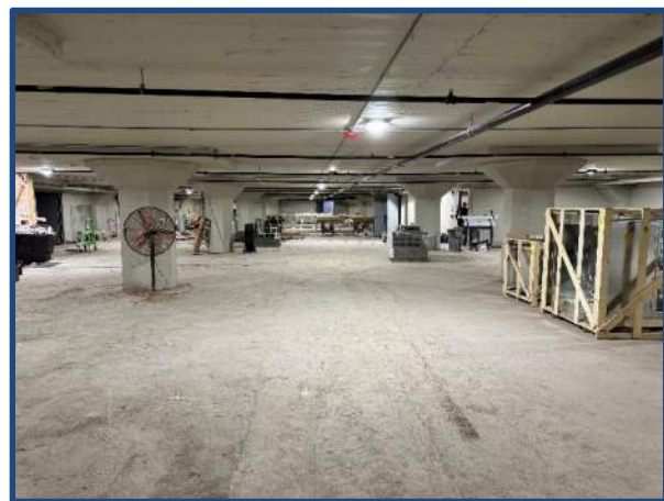
Basement Level (View from South, Looking North)
