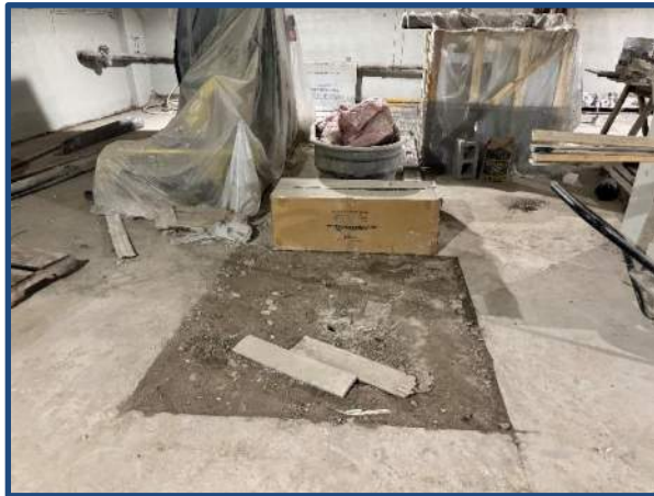
Basement Level, Section of Exposed Soil, Located in the South Portion.
