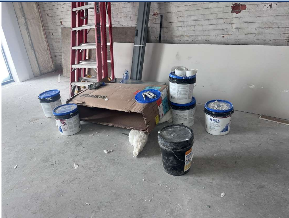
View of USG Plus 3 Joint Compound and Master Seal 610 stored in the Annex.
