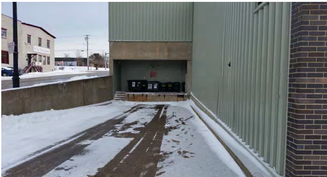
Photograph 2: Rear loading dock (north side) of the building along East Cayuga Street.
