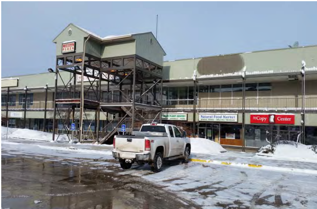
Photograph 1: Front (south side) of building.
