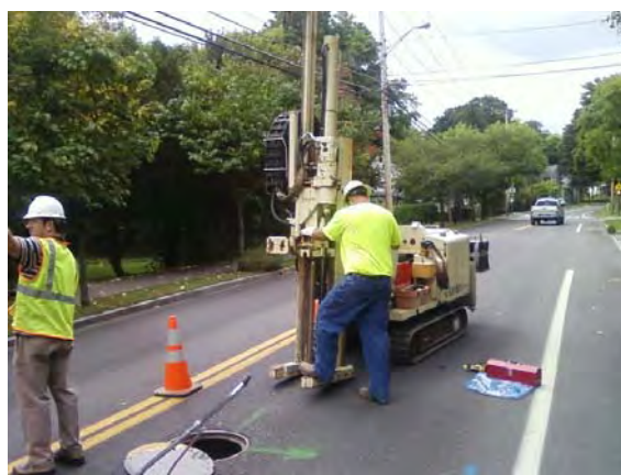
Geoprobe Utilized to Install Soil Vapor Point SV-18.
