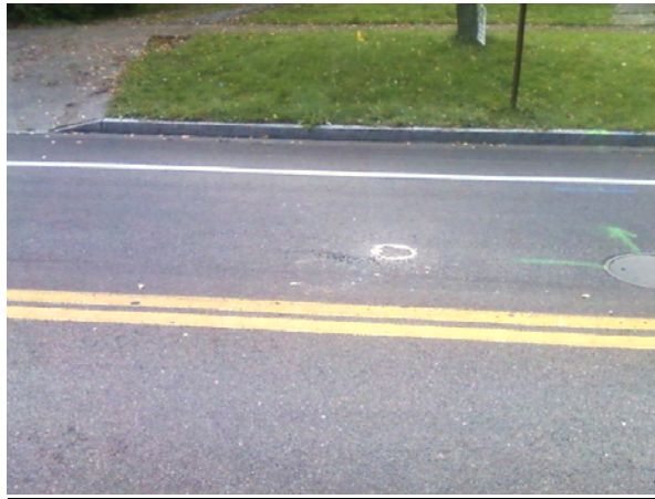
Cold Patch over removed curb box
