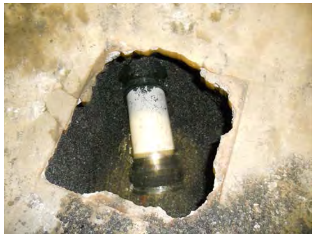
Connection of clay drain tile with PVC/Ferncos
