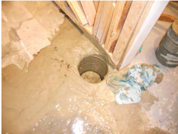
Concrete/Bedrock cored for EP-2
