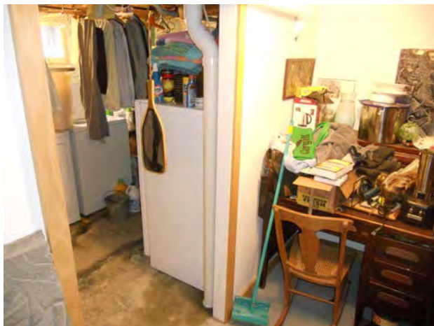
EP-2 in utility area.
