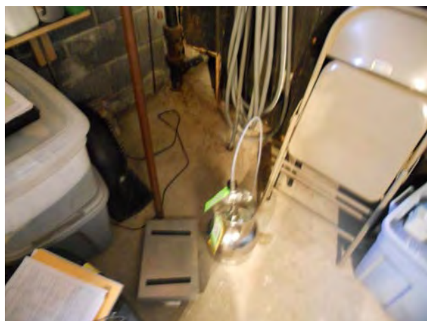
Structure 38 – Sub-Slab Vapor
