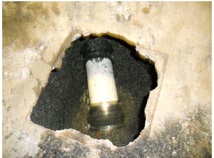
Floor drain reconnected –Structure 35
