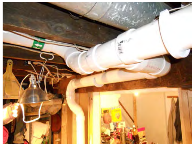
Tie-in between EP-2 and main line.
