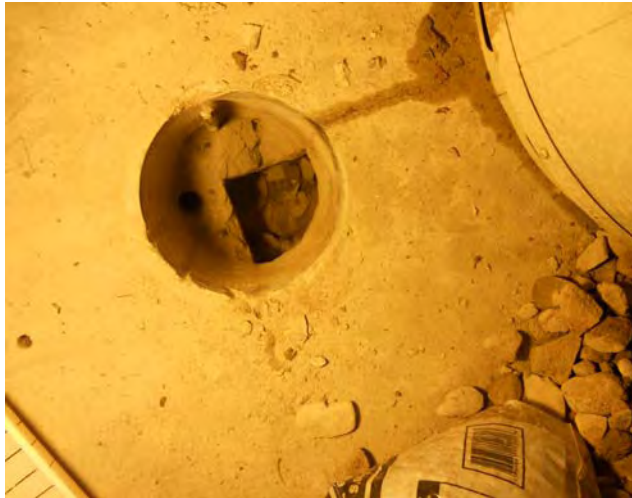
Concrete cored for EP-2
