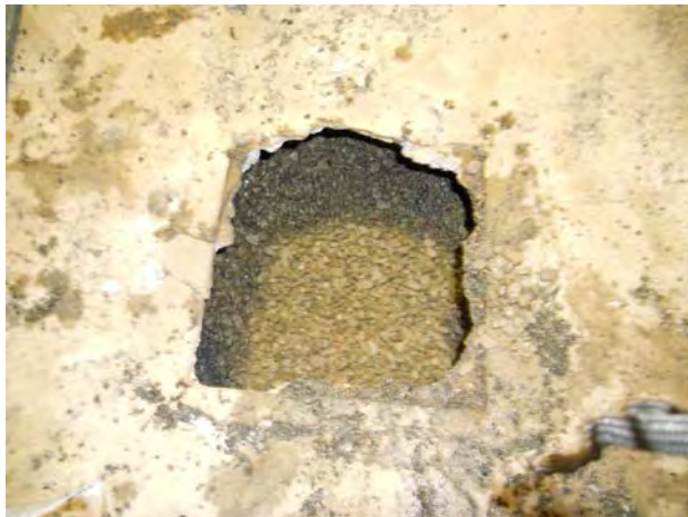
Gravel placed to fill void area where drain was previously located.
