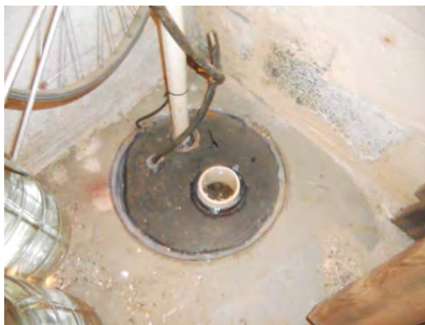
Resealed sump pit in Structure 39.
