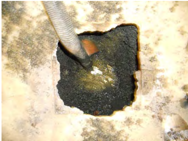
Cleaning out of floor drain/drain tile area
