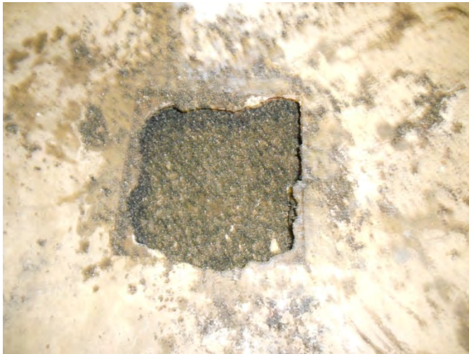
Peastone fill in former floor drain –Structure 35
