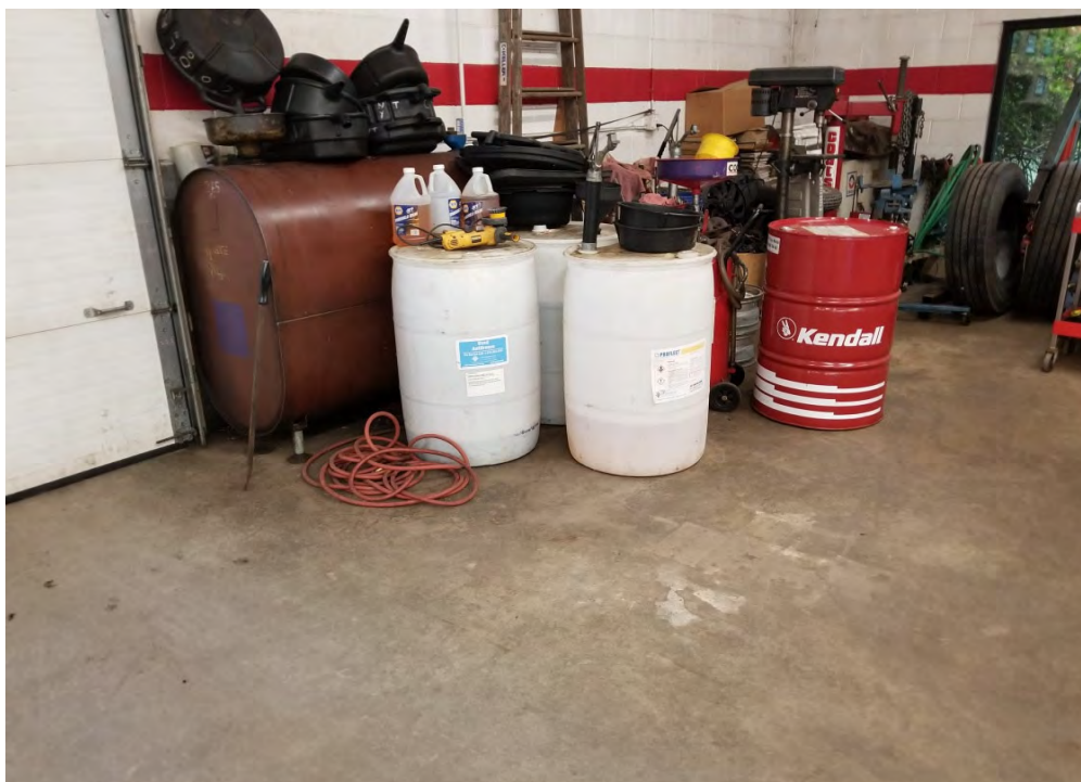
4. Southwest view - View of the 55-gallon drums for used antifreeze, a 265-gallon waste-oil AST, and a 55-gallon drum of new oil located on the southwest interior of the on-Site structure.
