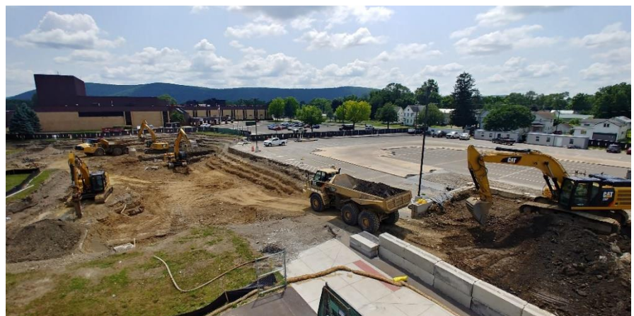
Cleanup activities on EHS property during summer 2019
