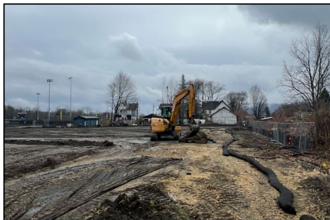
Figure 2: April 2024 – Restoration Activities in NAF
