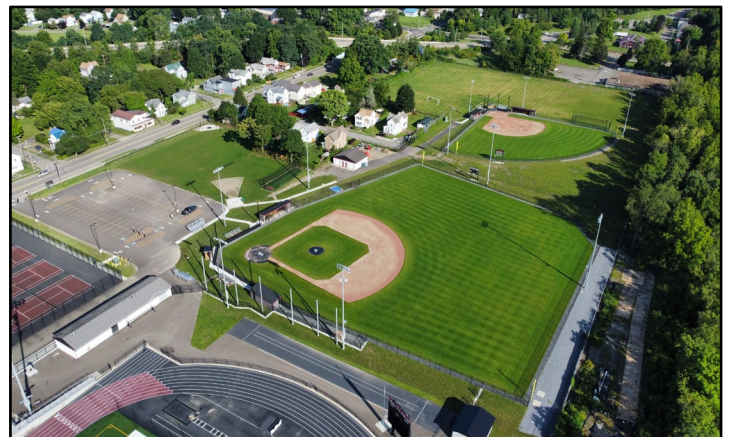
Figure 4: NAF (IRM 5A2) Completed Restoration August 2024 (looking northwest)
