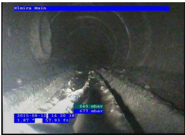
cb1 to tp9_c13cbdee-9df2-43af-9046-c2f05aa83cf0_20191227_1726 49_644.jpg, 00:07:53, 57.93ft Survey Abandoned / DSF
