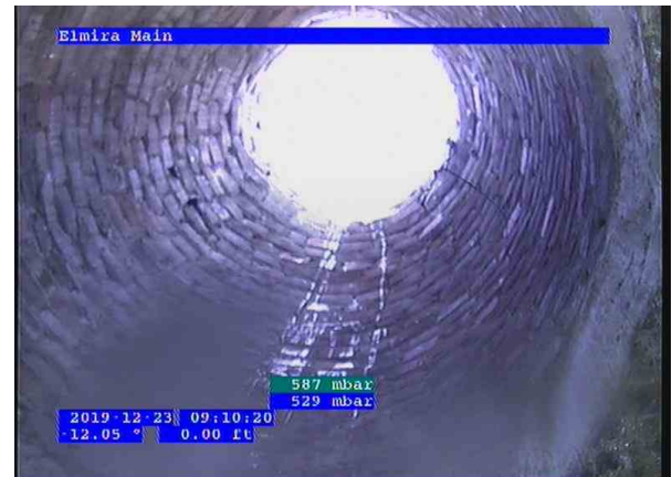
CB-15 to Unkonwn_3cf30b0b-8d8b-452e-a24c-83e6d7f293b5_2019122 3_092006_603.jpg, 00:00:00, 0.00ft Manhole / CB-15
