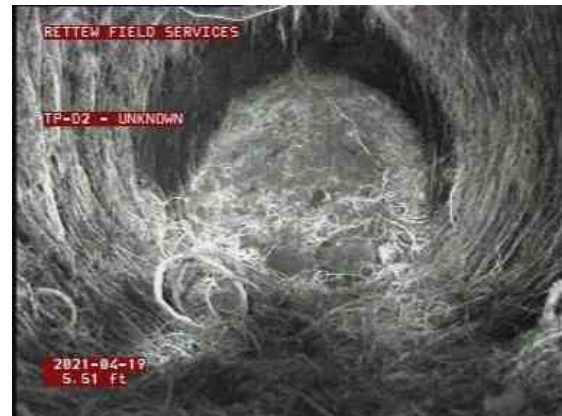
4, 00:00:30, 5.50ft Roots Ball Barrell from 12 o'clock to 12 o'clock, 100% lost
