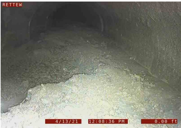
3, 00:00:12, 0.00ft Deposits Settled Fine, 50% of cross sectional area from 3 o'clock to 9 o'clock, Start
