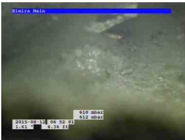
Test Pit 8 to CB-01_7d301137-cea9-4fa1-915d-9399ddef5823_20200116_ 204617_618.jpg, 00:05:12, 4.36ft Deposits Settled Compacted, 100% of cross sectional area from 12 o'clock to 12 o'clock
