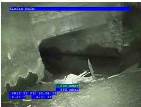
CB-15 to Unkonwn_8b18f192-5f82-4cb8-abec-494fe7f9c17e_20200116 _202616_483.jpg, 00:00:59, 0.00ft General Observation / Pipe to the west from CB15 main line in the large vault like manhole
