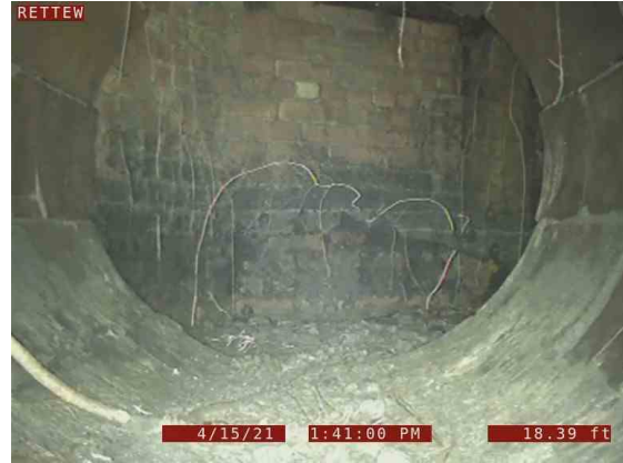
6, 00:01:35, 24.93ft Junction Box / Vault
