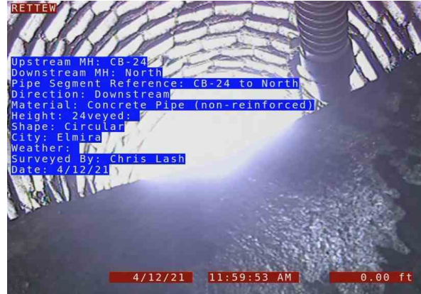
2, 00:00:00, 0.00ft Manhole / CB-24
