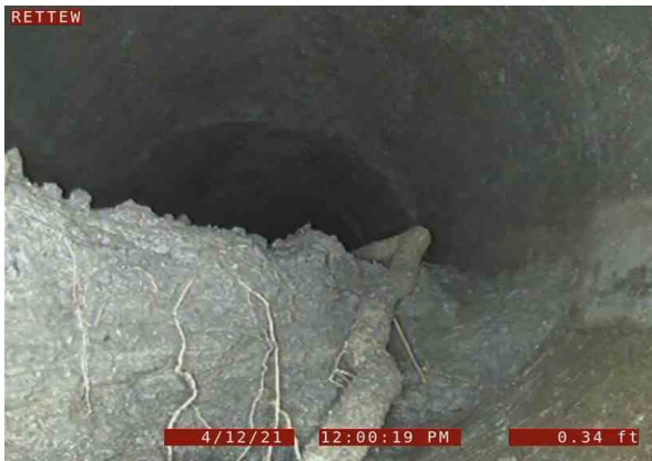
3, 00:00:30, 0.30ft Roots Tap Barrell at 6 o'clock, 15% of cross sectional area, Start
