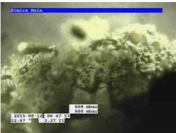
Test Pit 8 to the West_8c26fefb-8314-4832-b1af-1d2df3c1615e_20200130_19 2036_857.jpg, 00:01:04, 2.27ft Obstacles Other, 50% of cross sectional area from 3 o'clock to 9 o'clock / Mud
