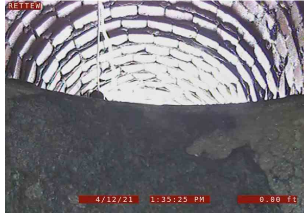
2, 00:00:00, 0.00ft Manhole / CB-24
