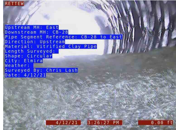
2, 00:00:00, 0.00ft Manhole / CB-28
