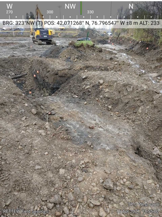
Test Pit D West Vault Structure
