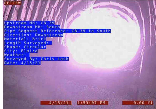
2, 00:00:00, 0.00ft Manhole / CB-39
