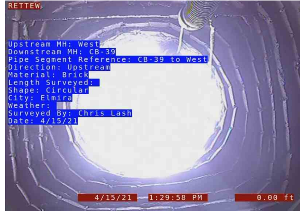
2, 00:00:00, 0.00ft Manhole / CB-39
