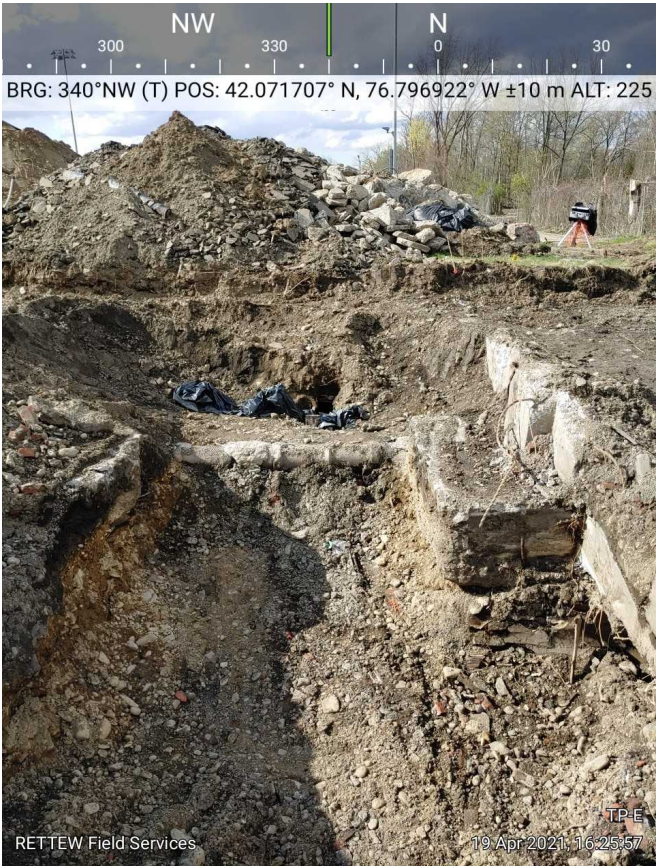
Test Pit E (TP-E)
