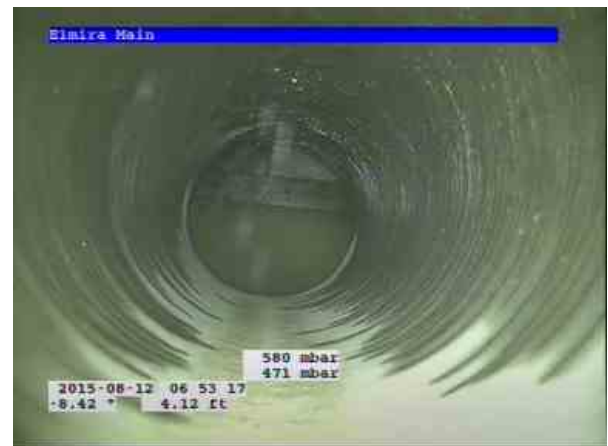
CB-08 to CB-05_82122a3b-94c4-4f3d-9f4d-24c45f0c4c50_20200116_2 05336_185.jpg, 00:07:22, 9.03ft Tee Connection at 12 o'clock, 12"inch vertical
