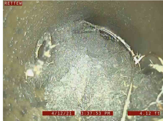
6, 00:03:32, 4.12ft Obstacles Other, 100% of cross sectional area from 12 o'clock to 12 o'clock / Roots and Soil
