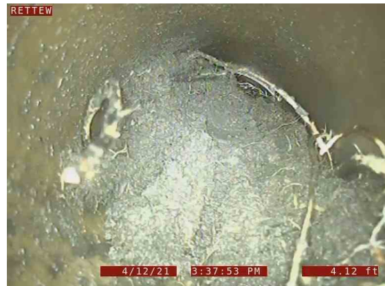
4, 00:03:32, 4.12ft Deposits Ingress Fine, 100% of cross sectional area from 12 o'clock to 12 o'clock
