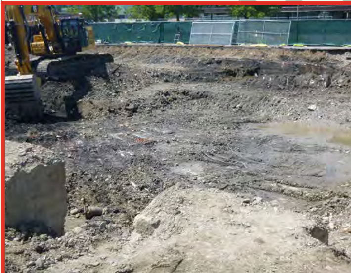
Concrete slab exposed at a depth of ~8.5 ft bgs
