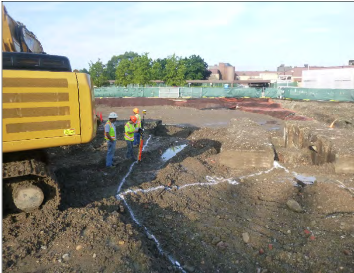
Layout of excavation extents
