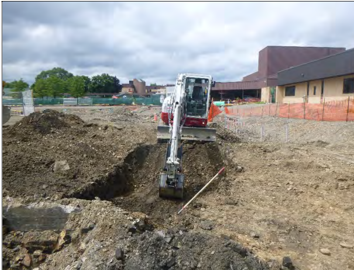
Miniexcavator to dig around electric and Gas lines
