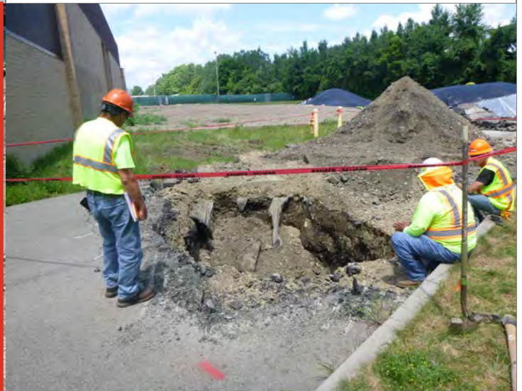
Scott Williams from the DEC and Recon at the water line excavation in the afternoon. Water line found at ~8 ft bgs.
