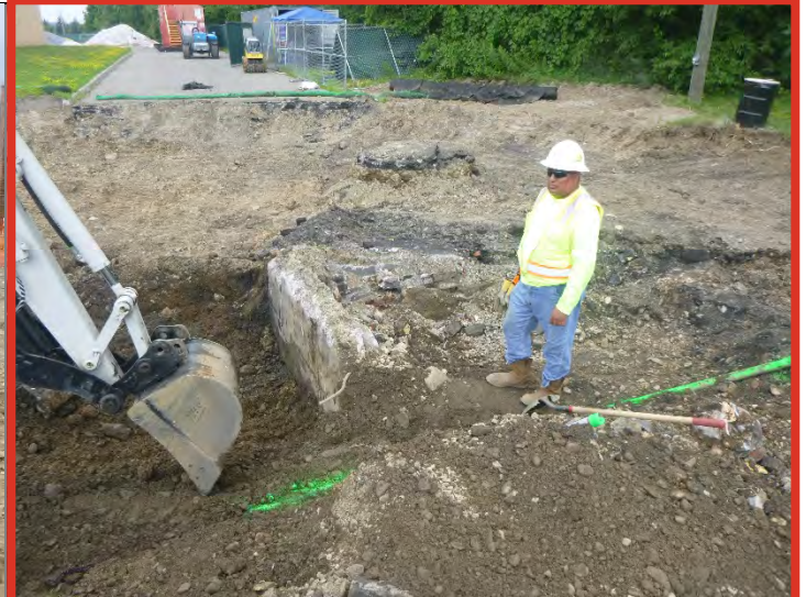
Concrete structure found adjacent to gas line
