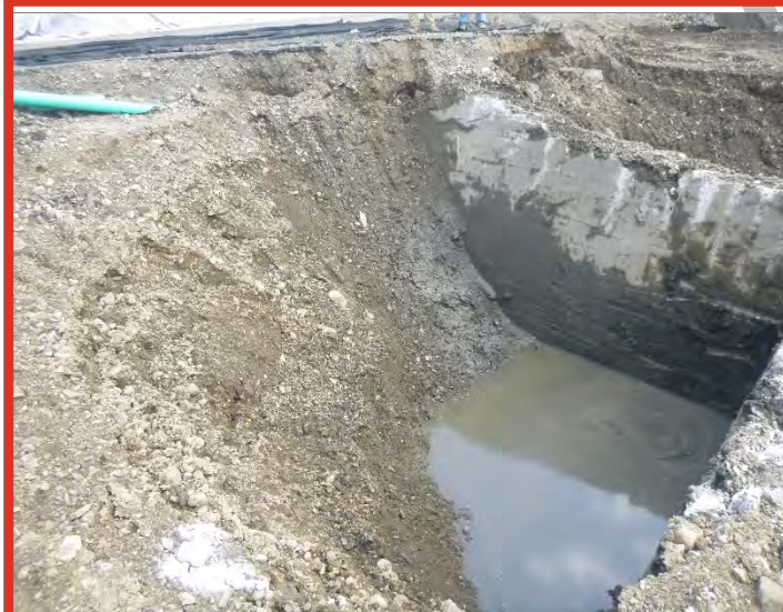
Bottom slab of concrete structure~13.5' + below BGS
