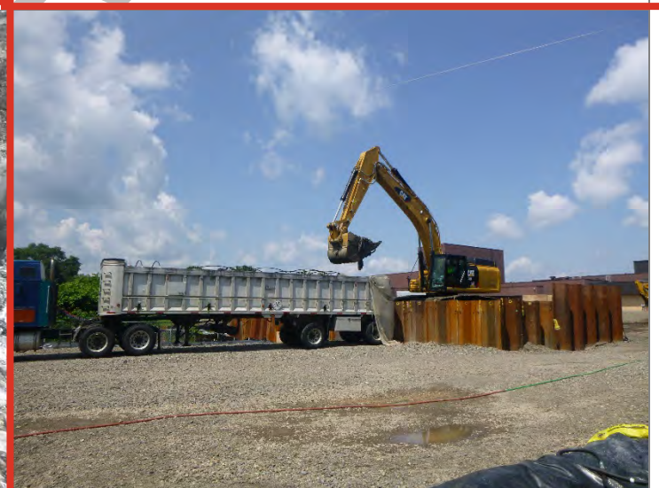
Loading of TSCA trucks
