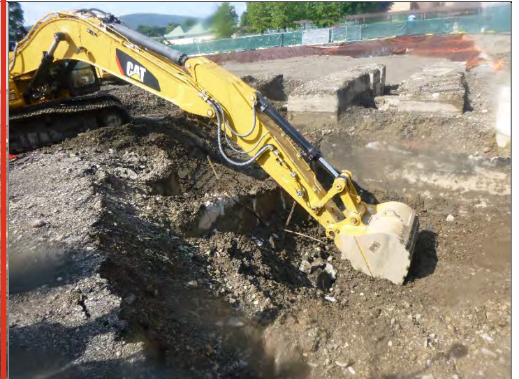
Exposed concrete structure
