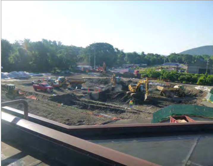
Morning view of site, with excavation continuing in Phase 2 and Phase 3
