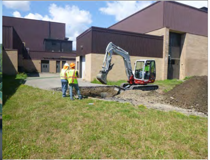
Recon beginning excavation of water line area in rear area of school.
