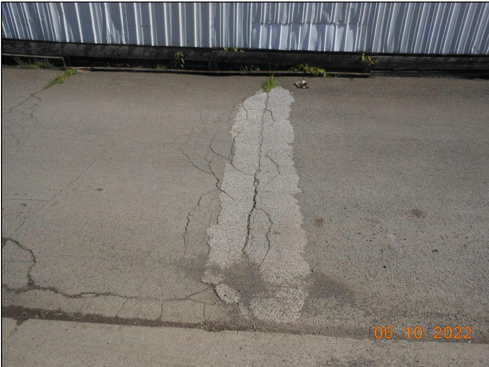
19.) PAOC 17 Bituminous Concrete Crack
