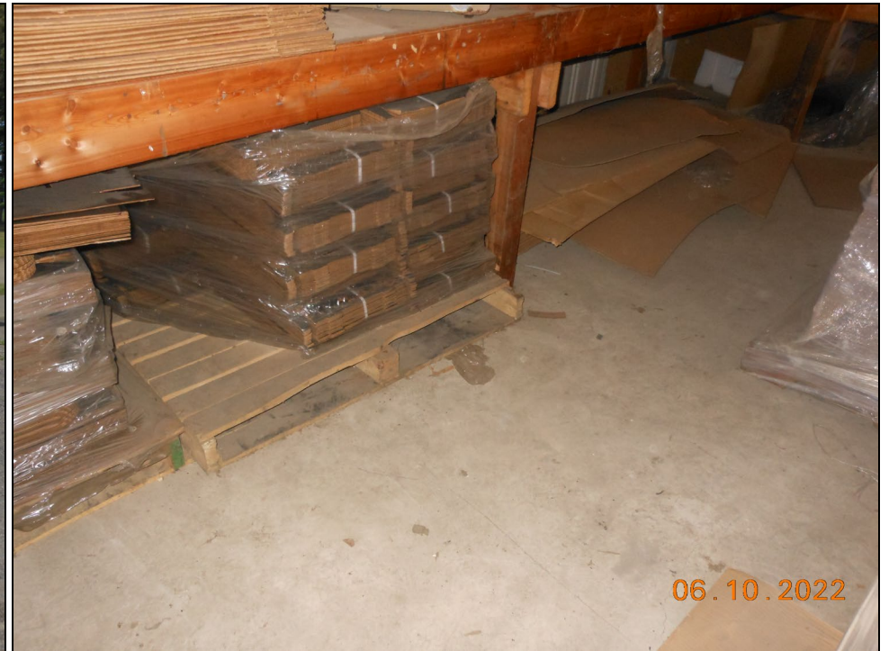
16.) PAOC 17 Concrete Floor Slab (Warehouse #3 SE Corner)
