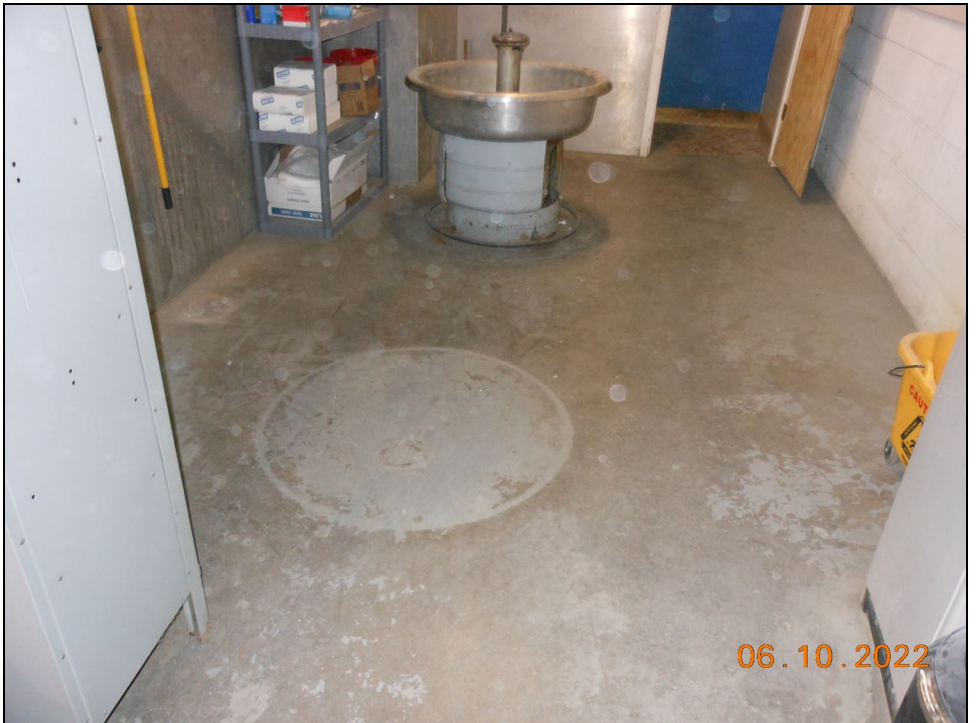
26.) PAOC 24 Concrete Floor Slab Cover – North Area
