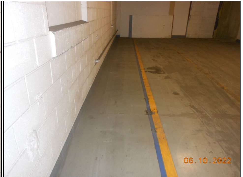
24.) PAOC 18 Concrete Floor Slab Cover – North – West Side
