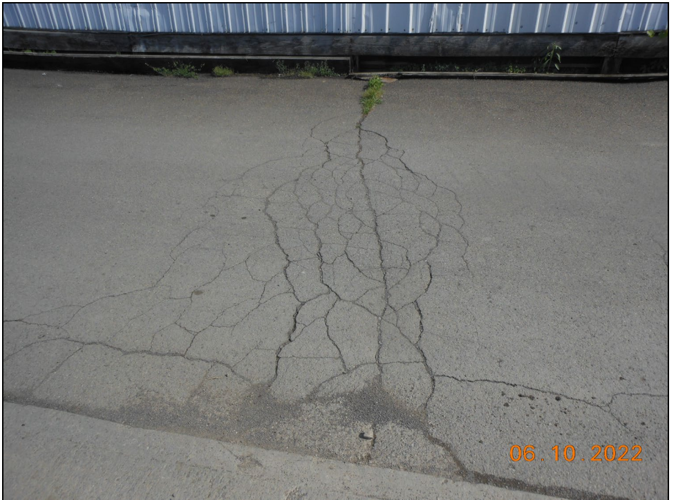
20.) PAOC 17 Bituminous Concrete Crack
