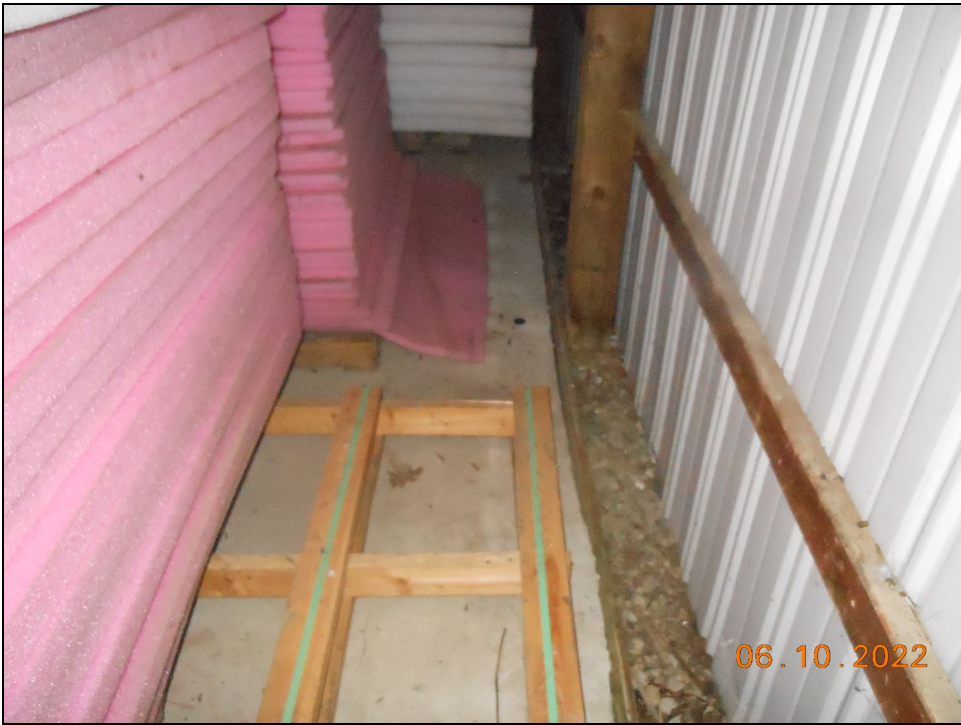
1.) PAOC 4 Concrete Floor Slab
