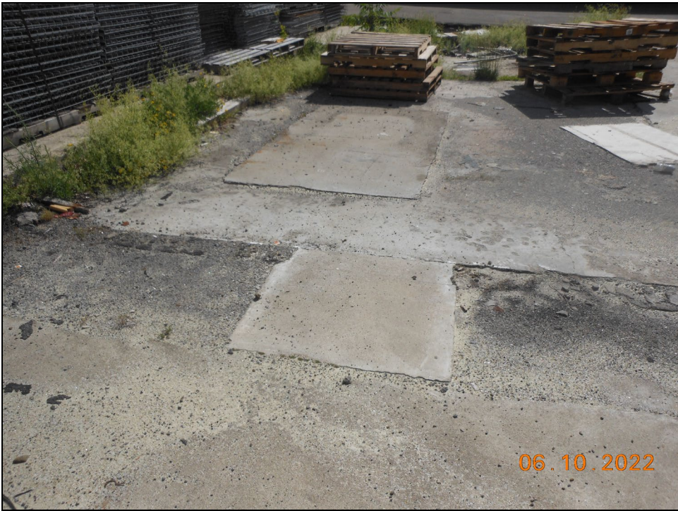
9.) PAOC 10/11 Concrete Floor Slab (North)
