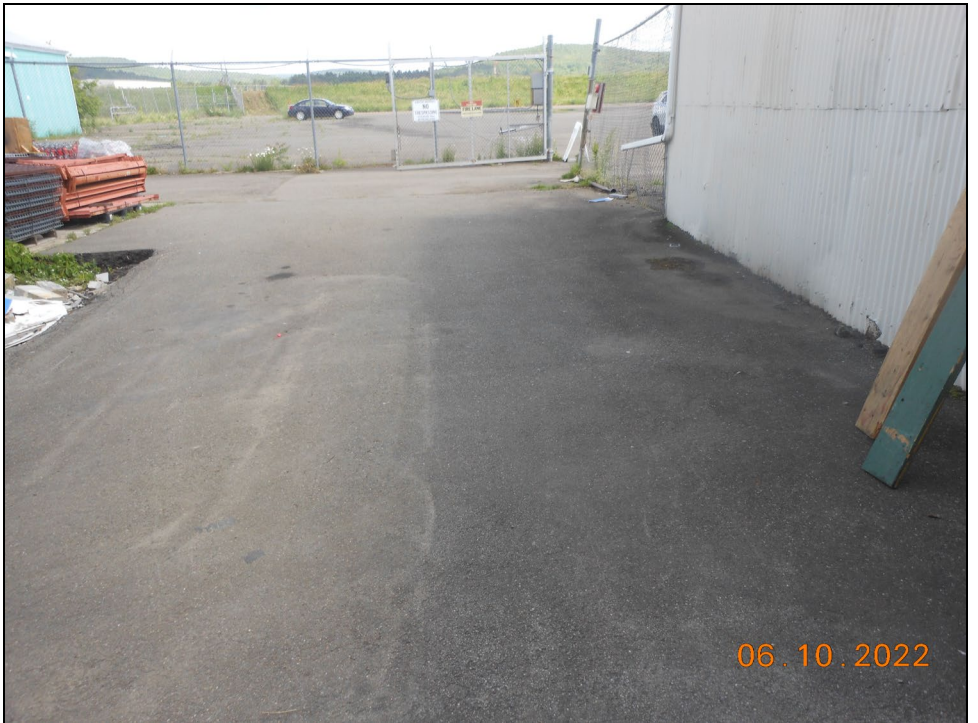
12.) PAOC 10/11 Bituminous Concrete Cover
