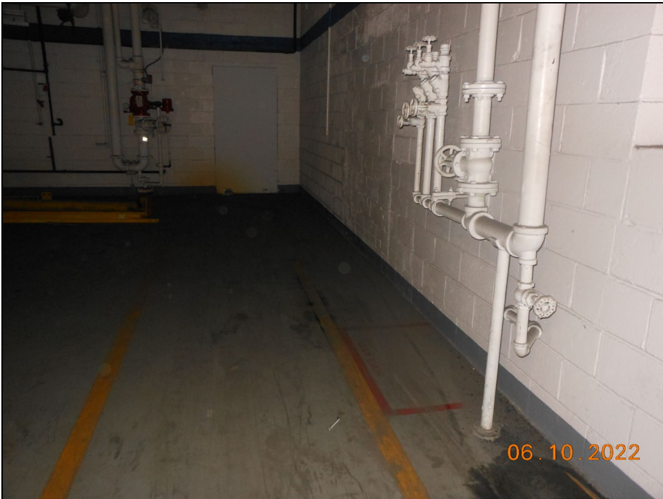
23.) PAOC 18 Concrete Floor Slab Cover – North – East Side
