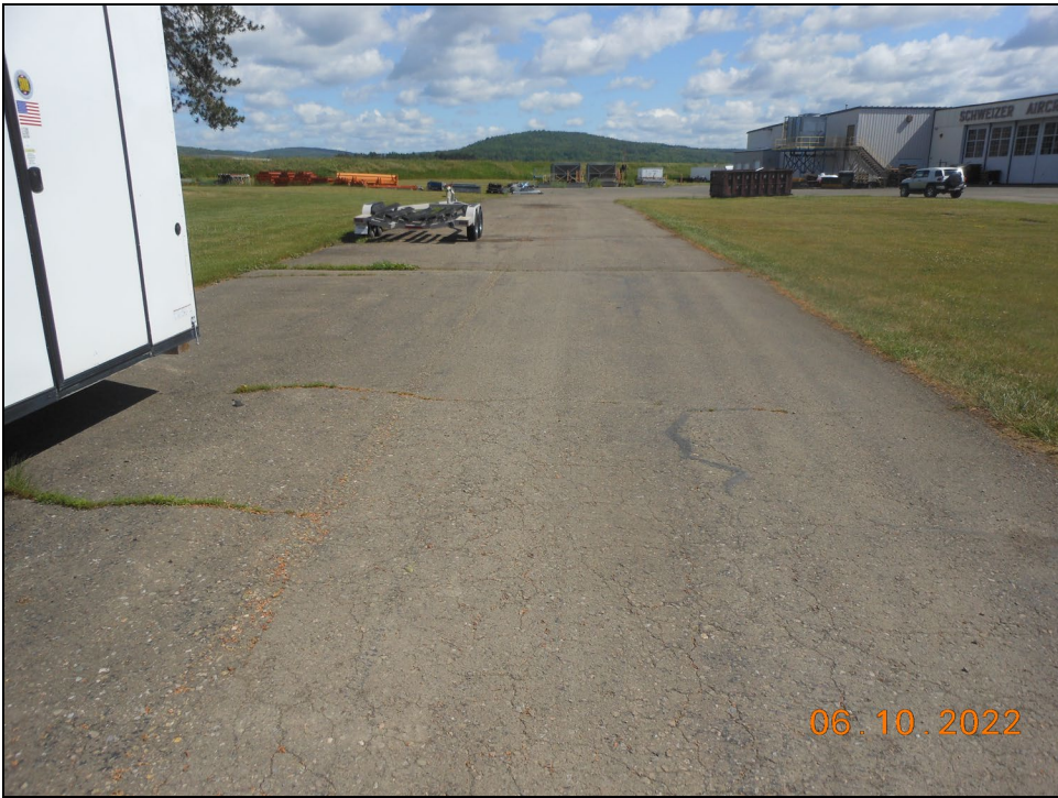
13.) PAOC 15 Bituminous Concrete Cover
