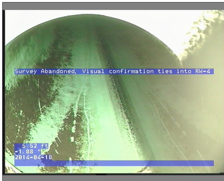
Photo: 6_1_3_18042014_112913_A.JPG, VCR No.: X 5.52FT, Survey Abandoned / Visual confirmation ties into RW-4
