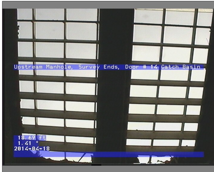
Photo: 3_1_2_18042014_100254_A.JPG, VCR No.: X 18.69FT, Upstream Manhole, Survey Ends / Door # 14 Catch Basin
