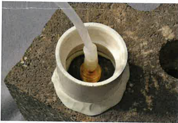
Figure 8. Water dam used for leak detection
