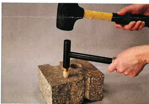
Figure 2. Installing the FLX-VP
