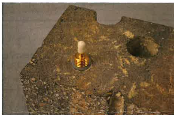
Figure 3. Installed VAPOR PIN®
