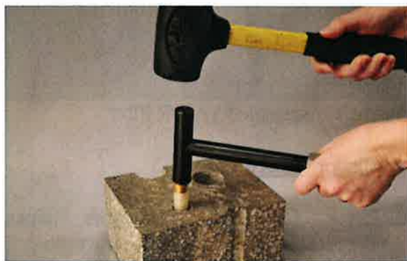
Figure 2. Installing the VAPOR PIN®
