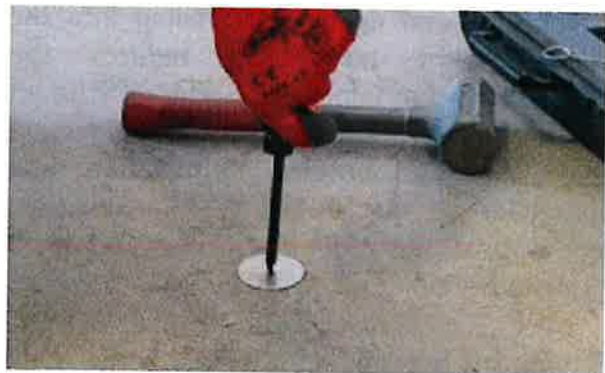
Figure 5. Tightening the Secured Cover
