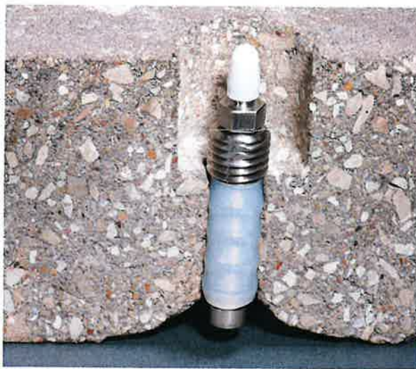
Figure 3. Installed FLX-VP
