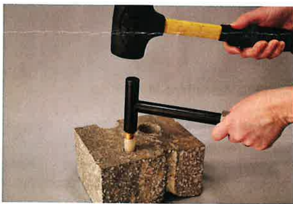
Figure 2. Installing the FLX-VP
