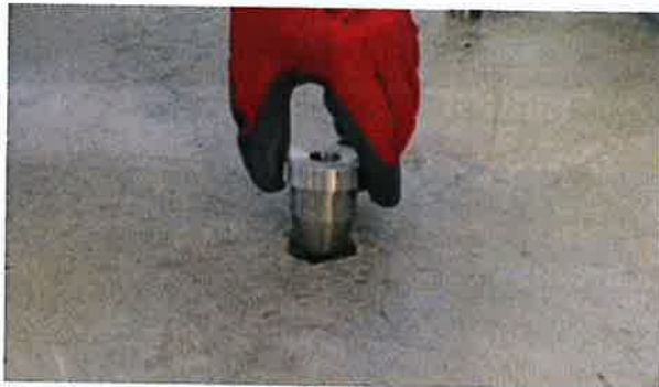
Figure 3. Testing Depth with the Drilling Guide
