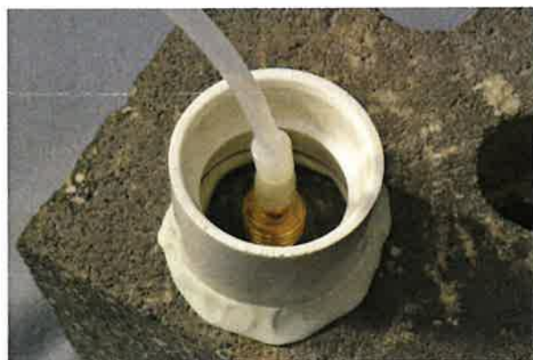
Figure 6. Water dam used for leak detection
