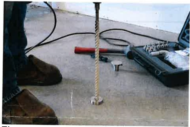
Figure 4. Using the Drilling Guide
