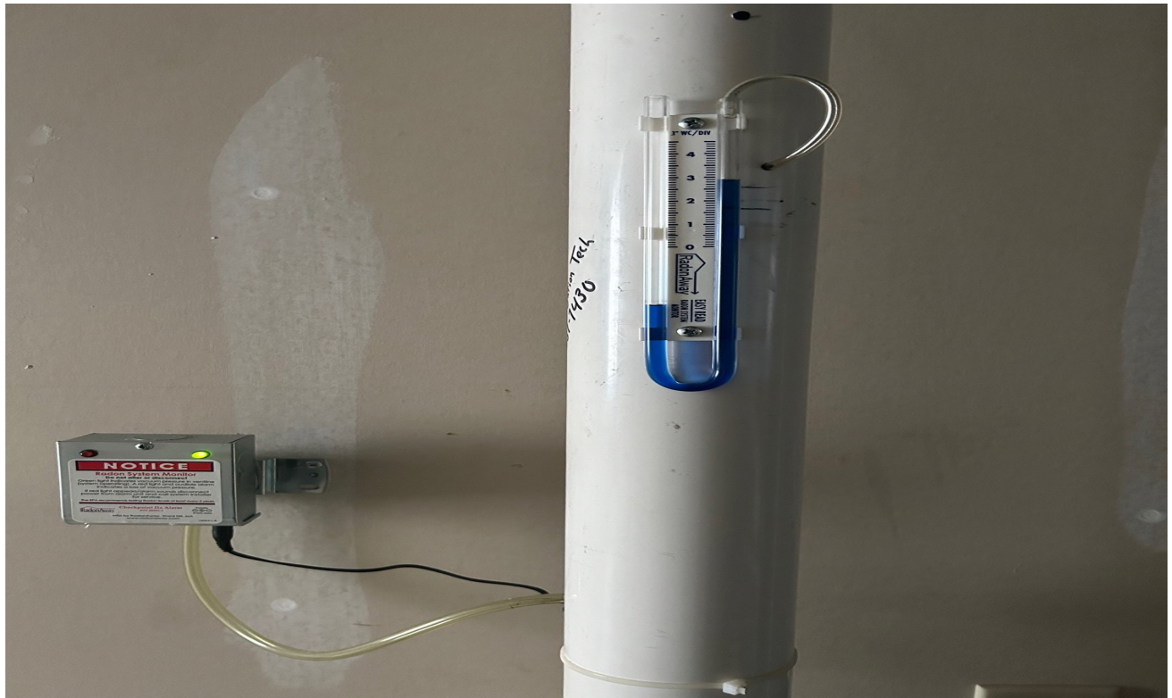
SSDS Alarm and Manometer
