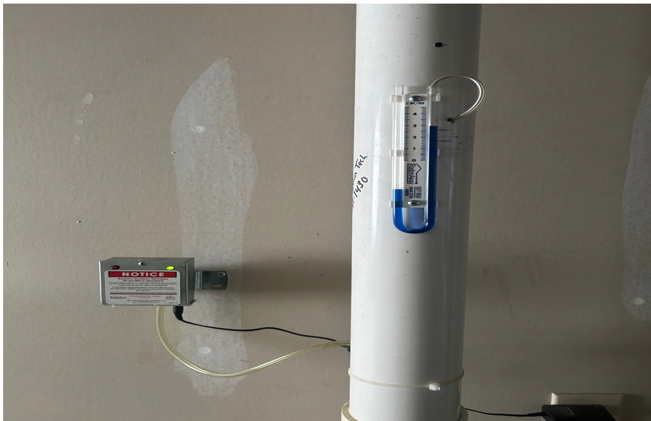
SSDS Alarm and Manometer
