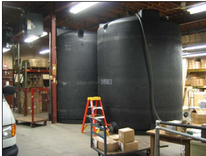
PHOTO 6 View of recovery Tanks 1 and 2 in the Building B Annex. The flexible discharge line is visible running up the side of Tank 1.
