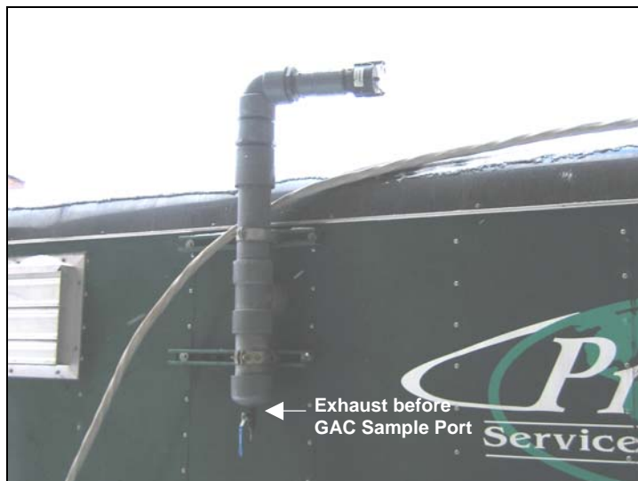
PHOTO 3 View of MPVE trailer exhaust point. Exhaust air was piped from this point to GAC treatment drums.
