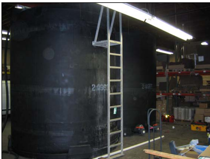
PHOTO 7 View of recovery tanks in Building B Annex. White 2" PVC header pipe is being set up along the edge of the tank.
