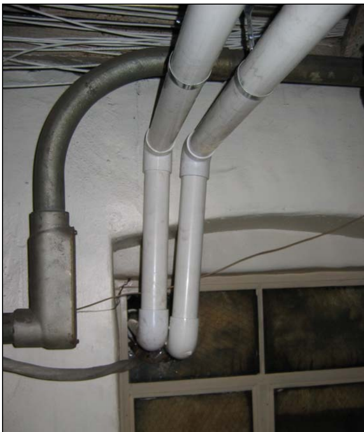
PHOTO 10 Header pipe and discharge pipe passing through a window along the north wall of Building B.
