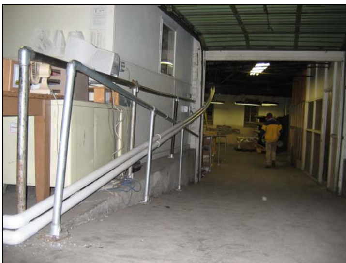
PHOTO 8 View of header pipe and discharge pipe from Building B Annex down ramp to Building B.
