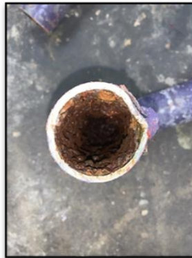
Interior of old water line pipe (July 1, 2020)
