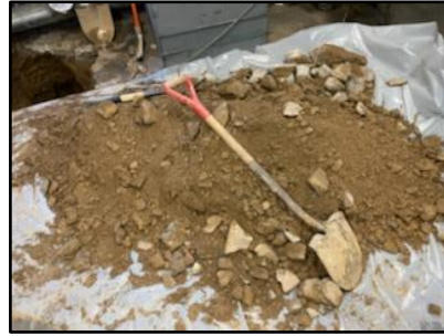
Staged excavated material inside the building on polyethylene sheeting (July 1, 2020)
