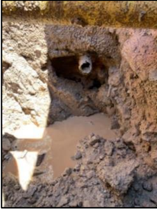
Water line pipe outside the building encased in concrete (July 1, 2020)
