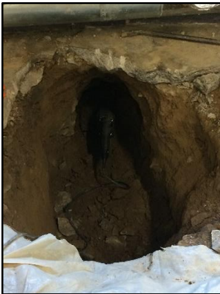
Excavated area inside building (July 2, 2020)
