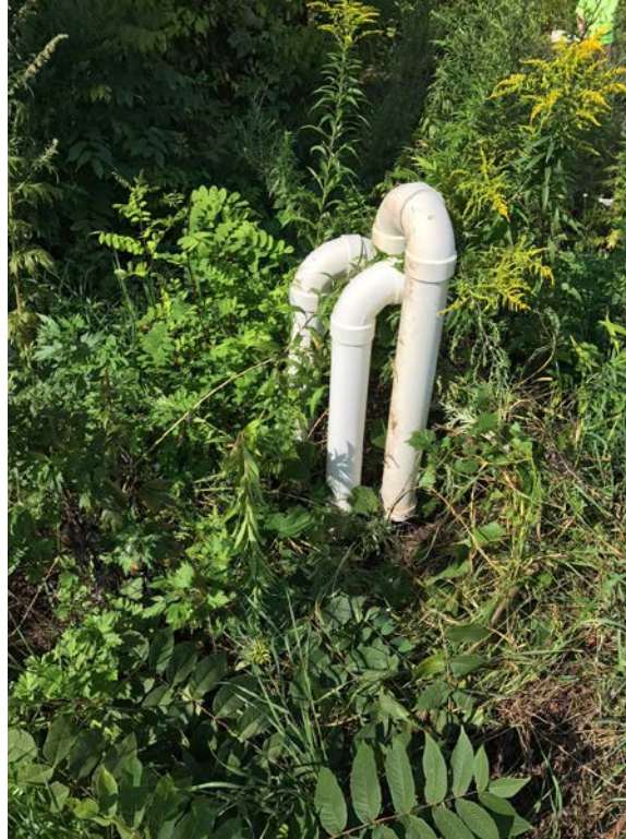
In-situ bioremediation system air influent vent piping, with one being unattached (8-16-2017)
