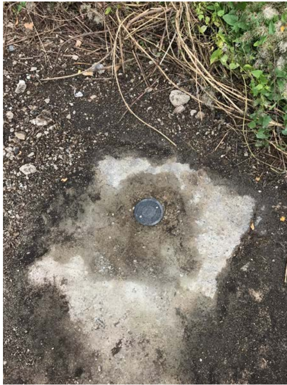
Monitoring well MW-6 with repaired curb box (8-31-2017)
