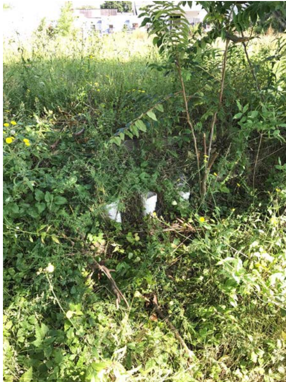
In-situ bioremediation system air effluent piping missing PVC stick-ups and wind turbines (8-16-2017)
