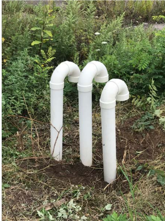
Re-attached in-situ bioremediation system air influent vent piping (8-31-2017)
