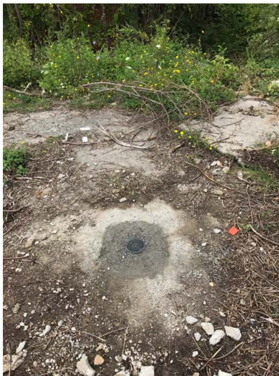
Monitoring well MW-13 with repaired curb box (8-31-2017)
