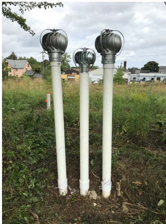
Repaired in-situ bioremediation system air effluent PVC piping and wind turbines (8-31-2017)
