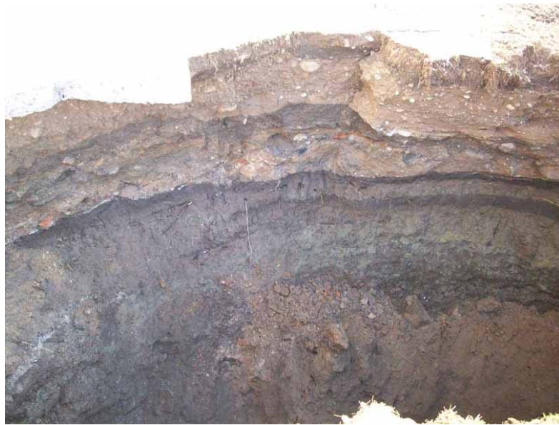
View of north wall – excavation of Cell 1C showing soil sloughing from Cell 3B (4-16-08)
