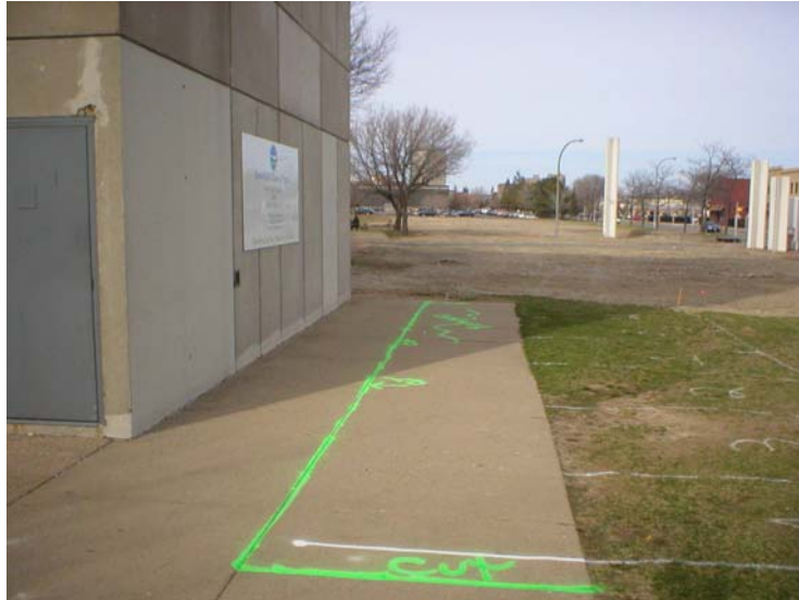
View looking northeast – Pre-excavation mark-out of excavation limits
