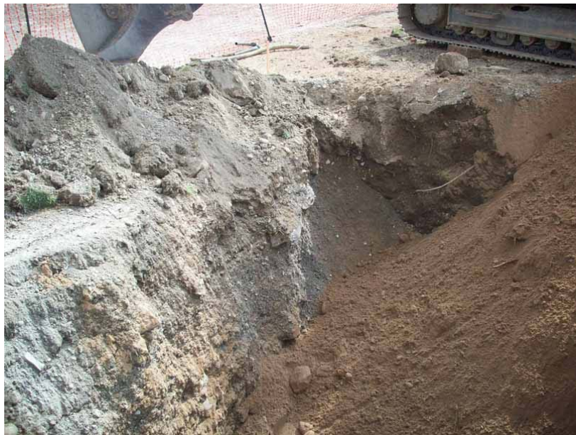
Backfilling Cell 2A with bank run (04-16-08)
