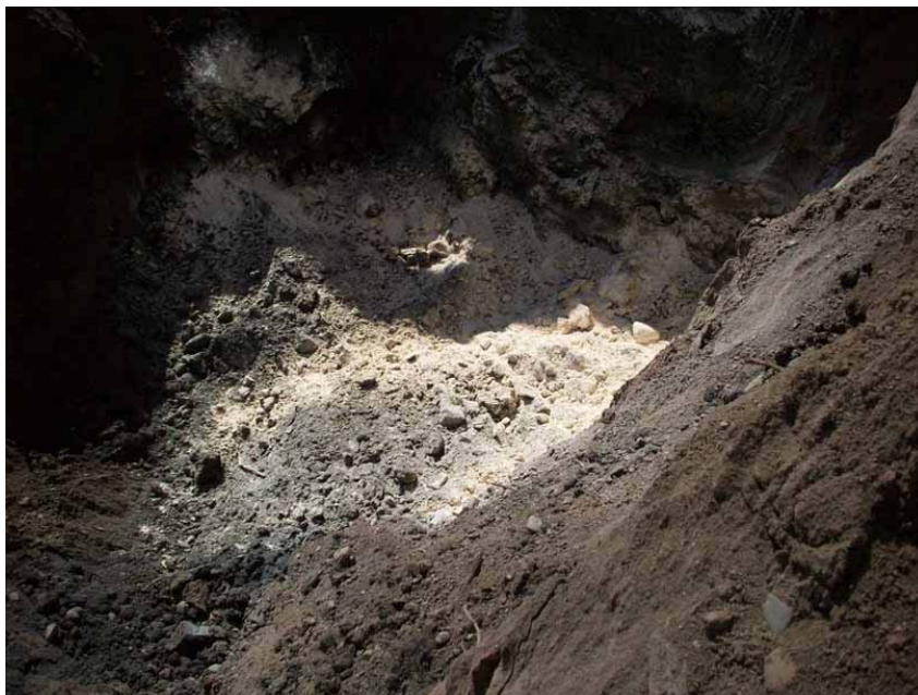
ORC-Advanced applied to bottom of Cell 4C prior to backfilling (4-17-08)
