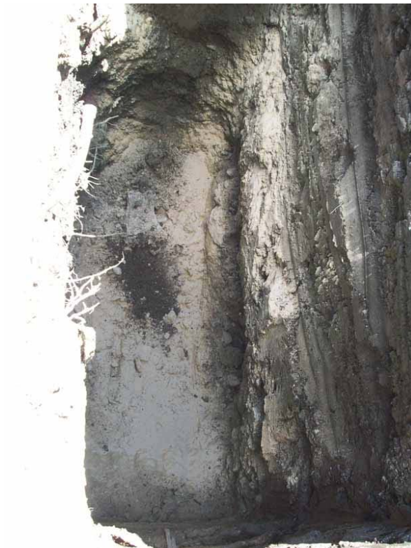
ORC- Advanced applied to bottom of Cell 1B prior to backfilling (04-15-08)
