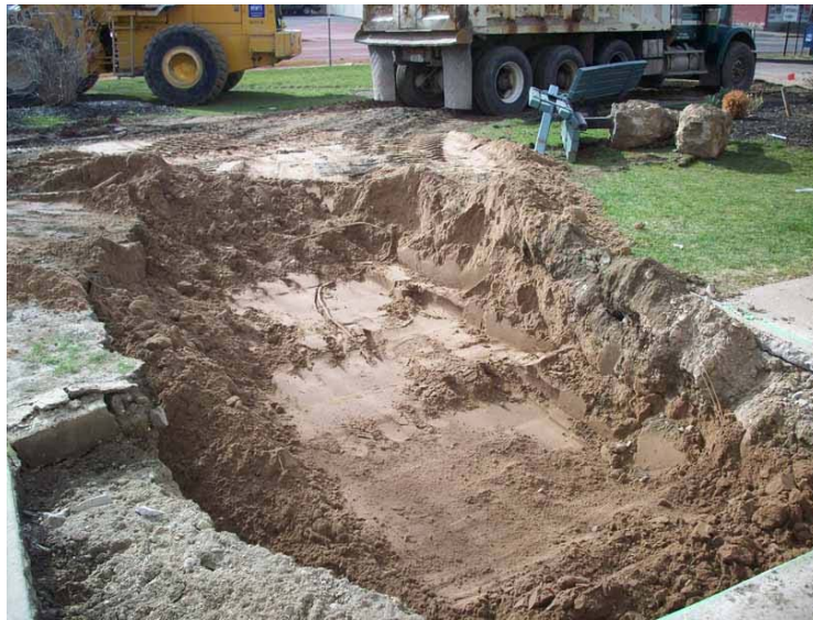
Backfill of excavation Cell 1C using bank run sourced off site (04-16-08)
