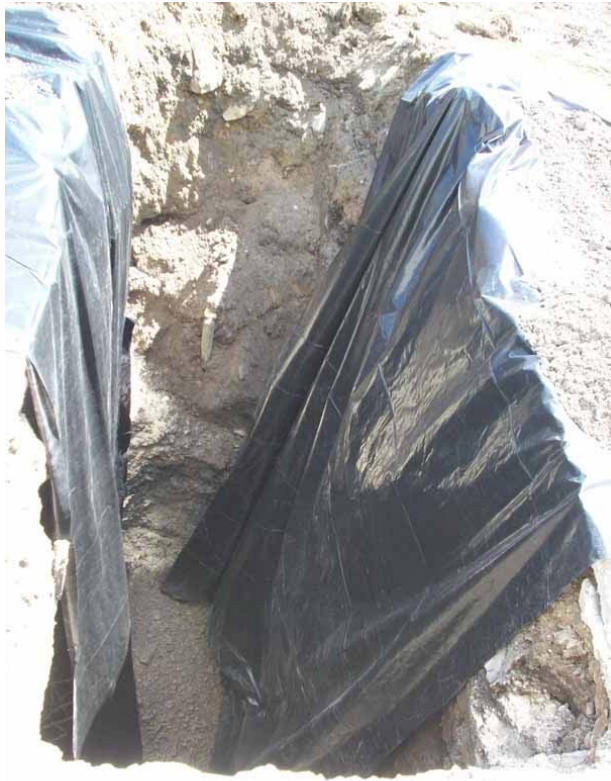
Installation of plastic sheeting during backfilling to separate contaminated soil and clean backfill between adjoining cells (04-15-08)
