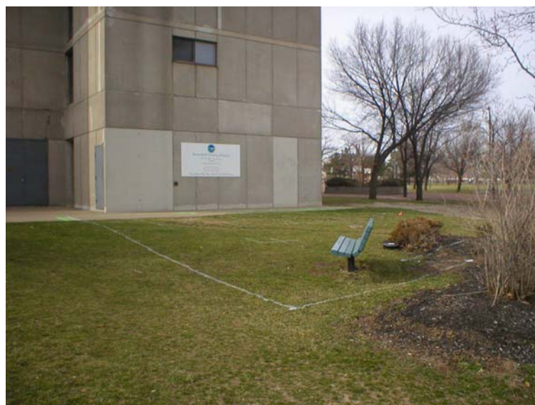
View northwest – Pre-excavation mark out of excavation limits
