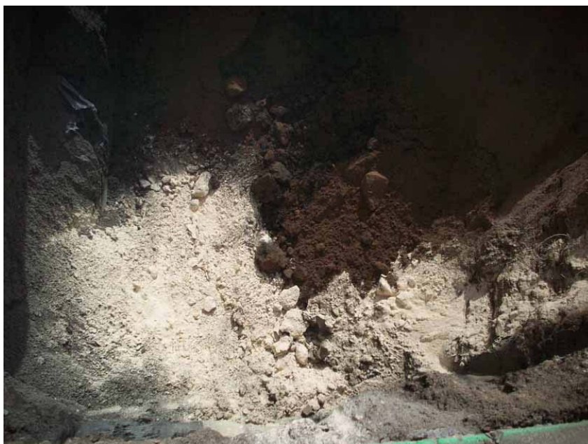
ORC-Advanced applied in the bottom of excavation Cells 2B and 3B (04-16-08)
