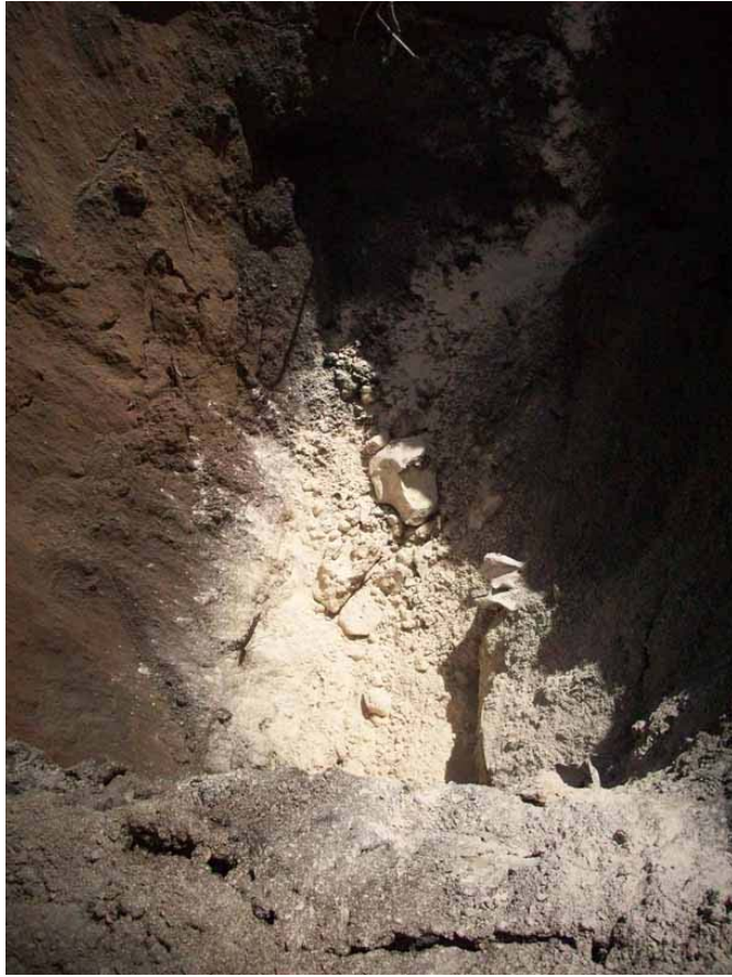
ORC-Advanced applied to the bottom of Cell 3A prior to backfilling (04-16-08)
