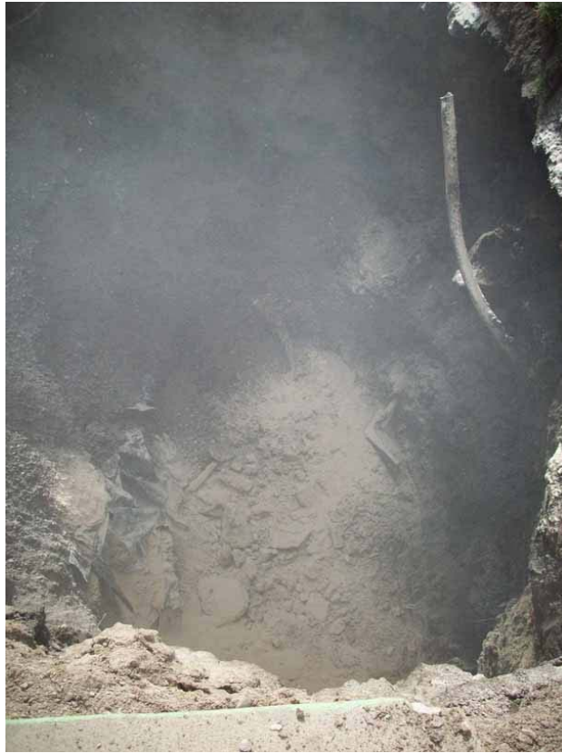
ORC- Advanced applied to the bottom of Cell 2A prior to backfilling (04/16/08)
