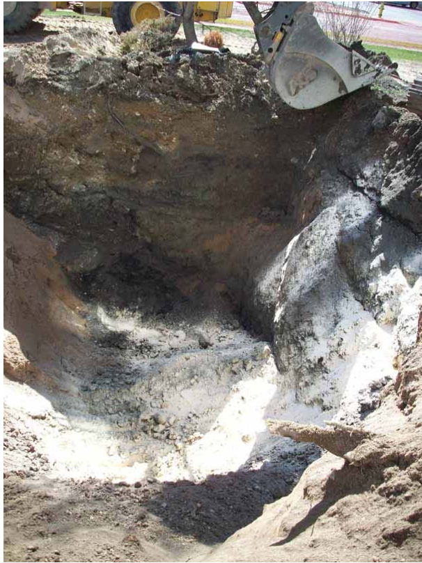
ORC-Advanced applied to bottom of Cell 4B prior to backfilling (04-17-08)
