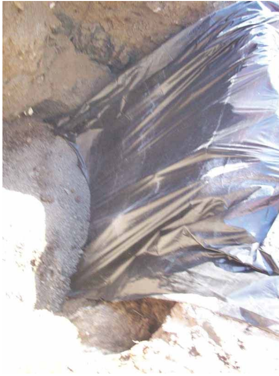
Installation of plastic sheeting during backfilling to separate contaminated soil and clean backfill between adjoining cells (04-15-08)
