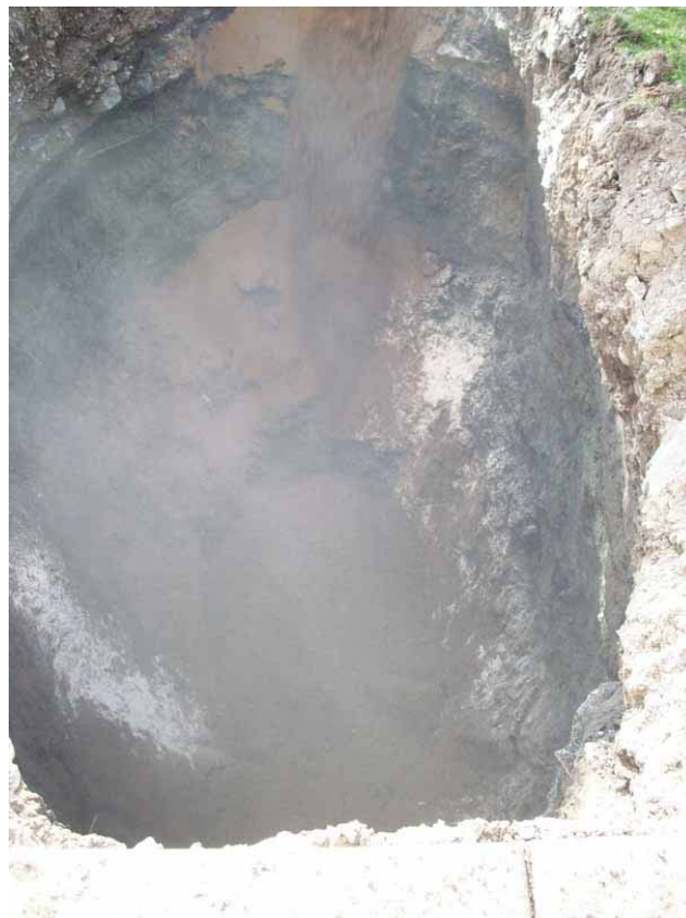
ORC- Advanced applied to bottom of Cell 1C prior to backfilling (04-16-08)
