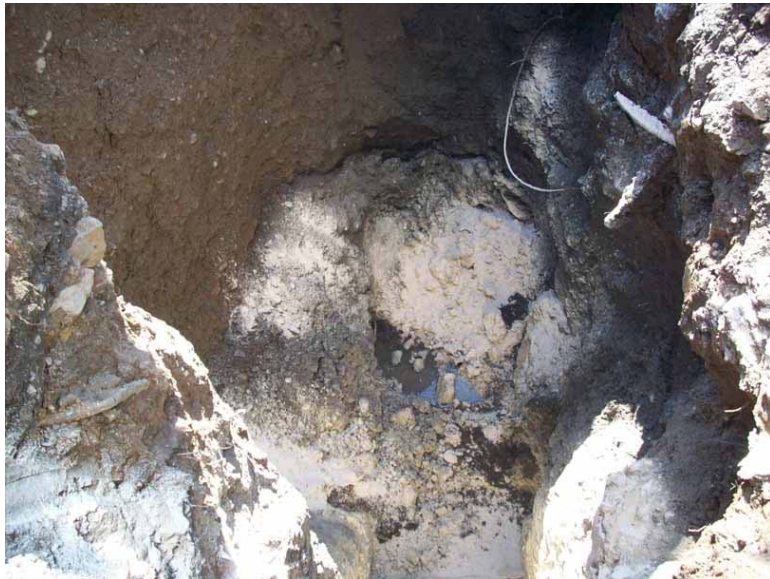
ORC-Advanced applied to the bottom of Cell 1A before backfilling (04-15-08)
