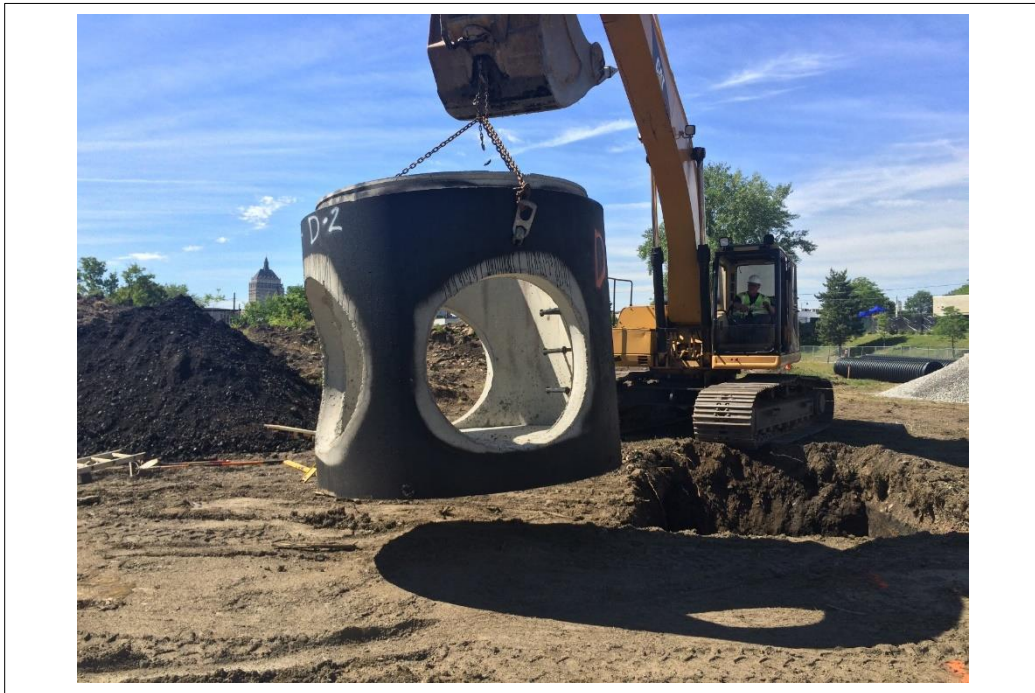
Stormwater retention system installation on subject property
