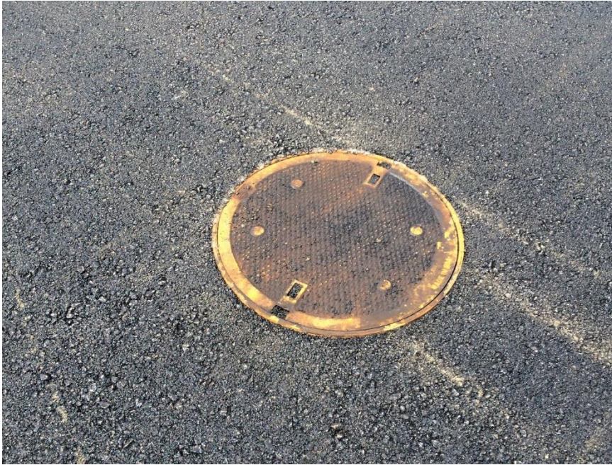
Stormwater collection manhole in cover system
