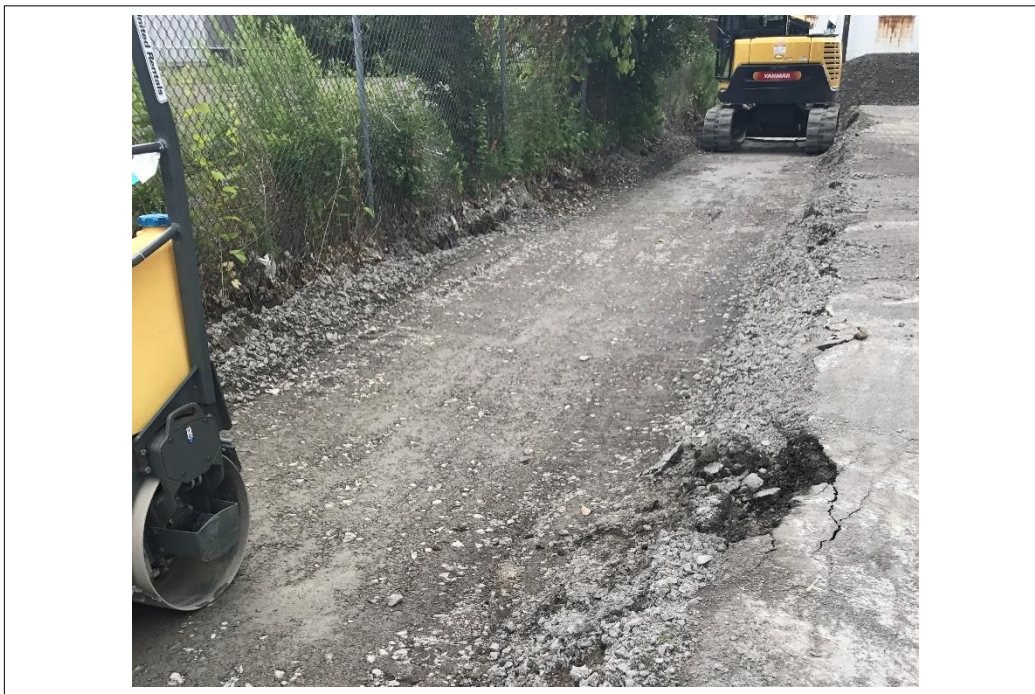
Gravel laid over on east side of ROW
