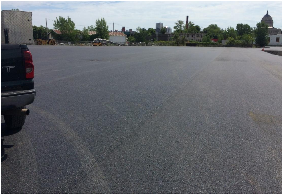
Capping of back lot with asphalt paving
