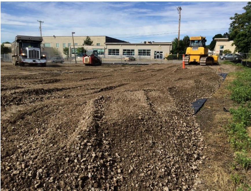
Mixed crush concrete spread out with subject property
