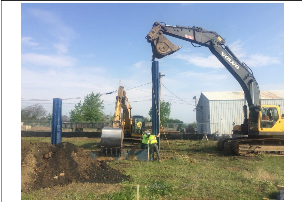
Hot Spot excavation, installation of shoring
