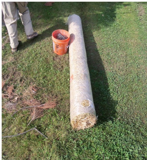
Straw erosion mat used on west side of Haidt Place
