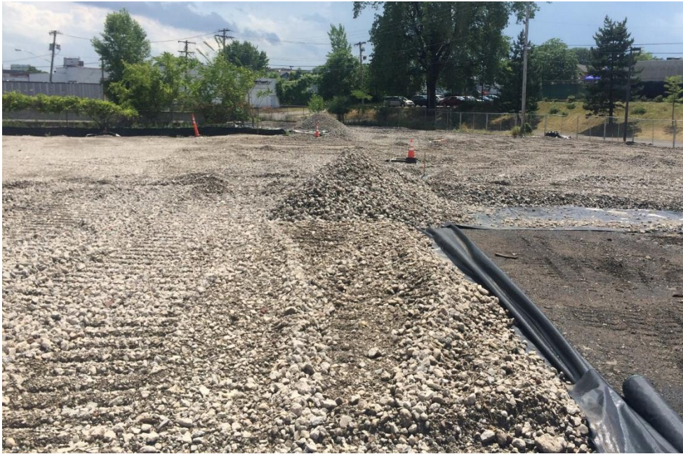
Mixed crush concrete spread out with subject property
