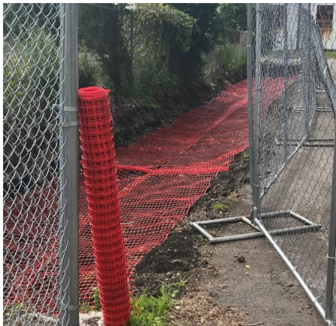
Orange plastic barrier laid on the east side of the ROW
