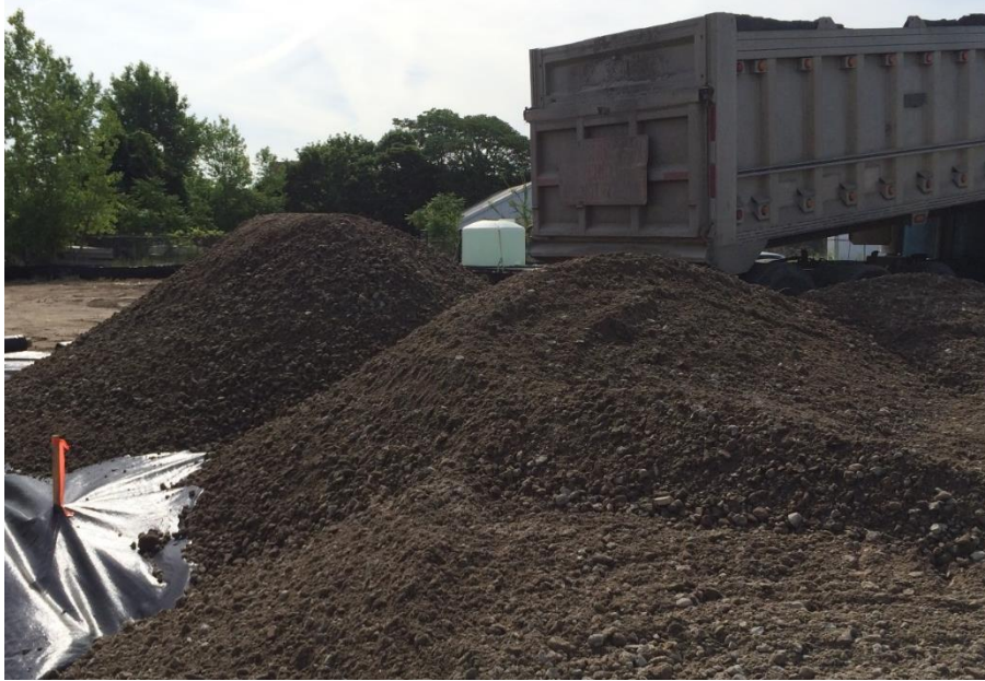
Delivery of mixed crush concrete spread out with subject property
