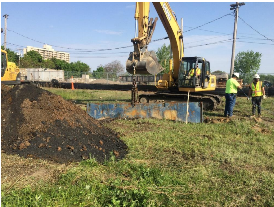
Hot Spot excavation, installation of shoring
