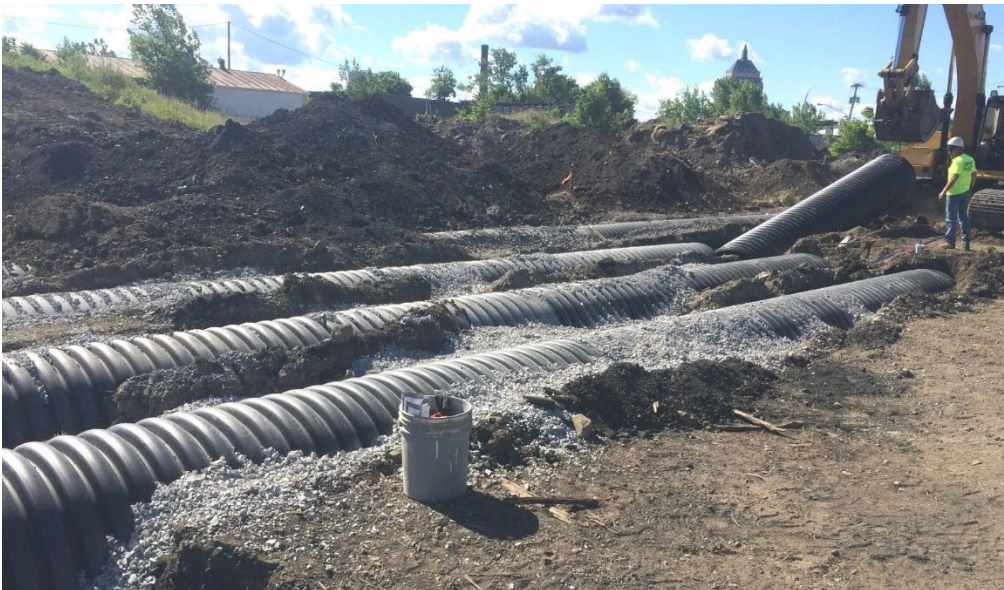
Stormwater retention system installation on subject property
