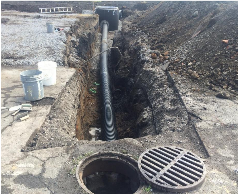
Dewatering system and sewer line installation on subject property
