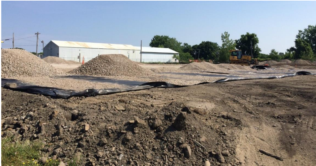
Mixed crush concrete spread out with subject property
