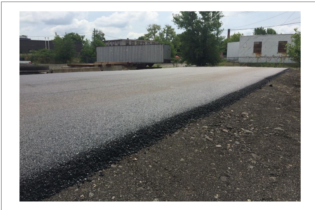
Capping of back lot with asphalt paving
