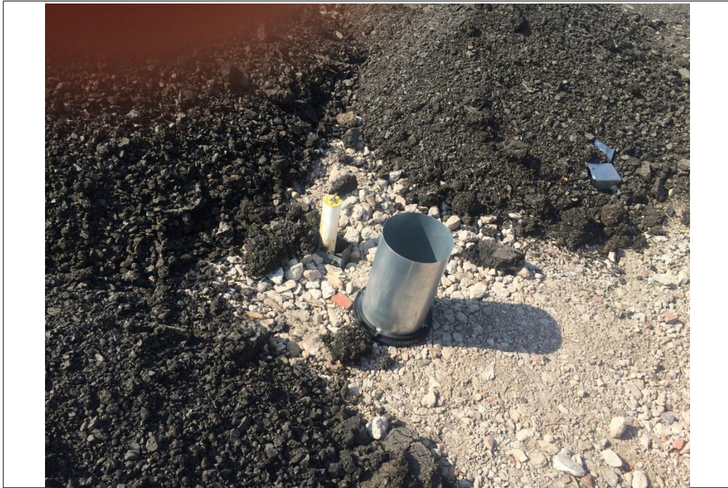
Retro fit monitoring well surface completion
