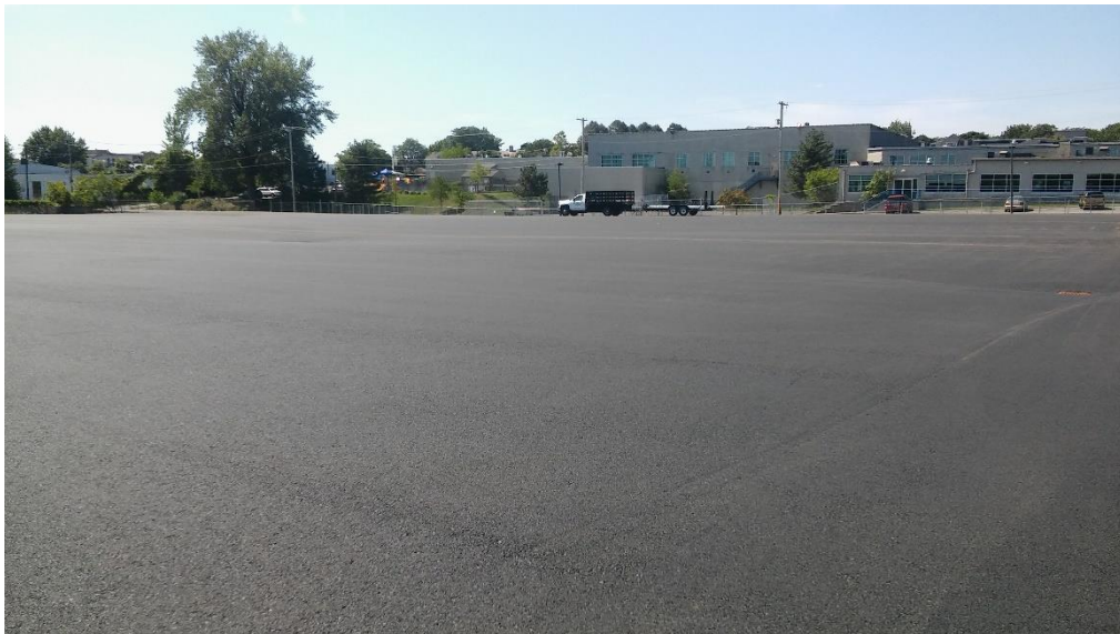
Capping of back lot with asphalt paving
