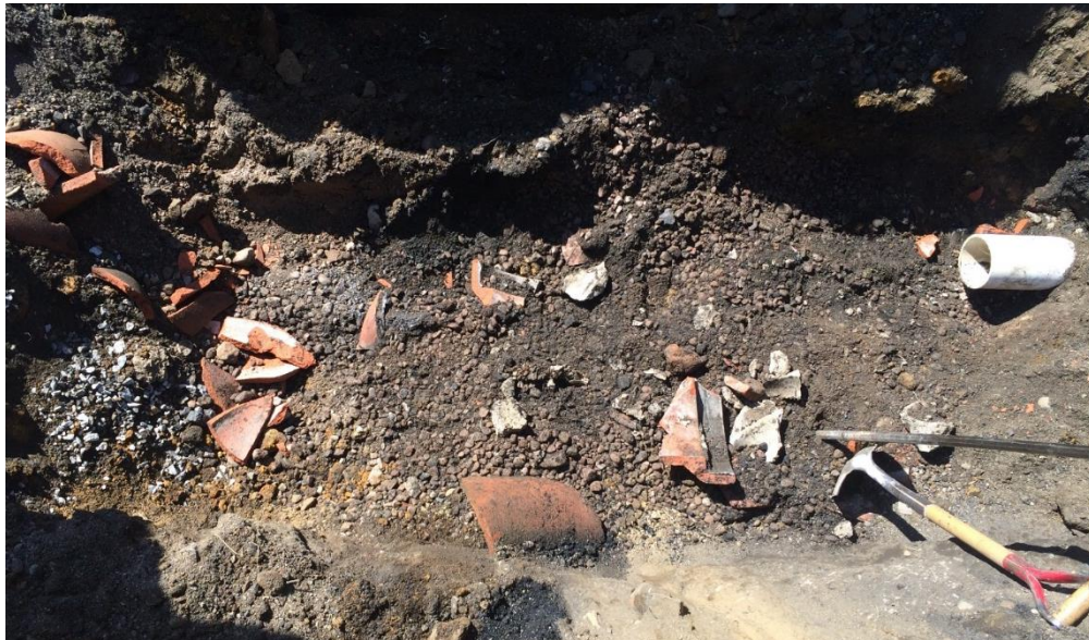
Discovered 6" pipe within 10" pip leading to sewer line
