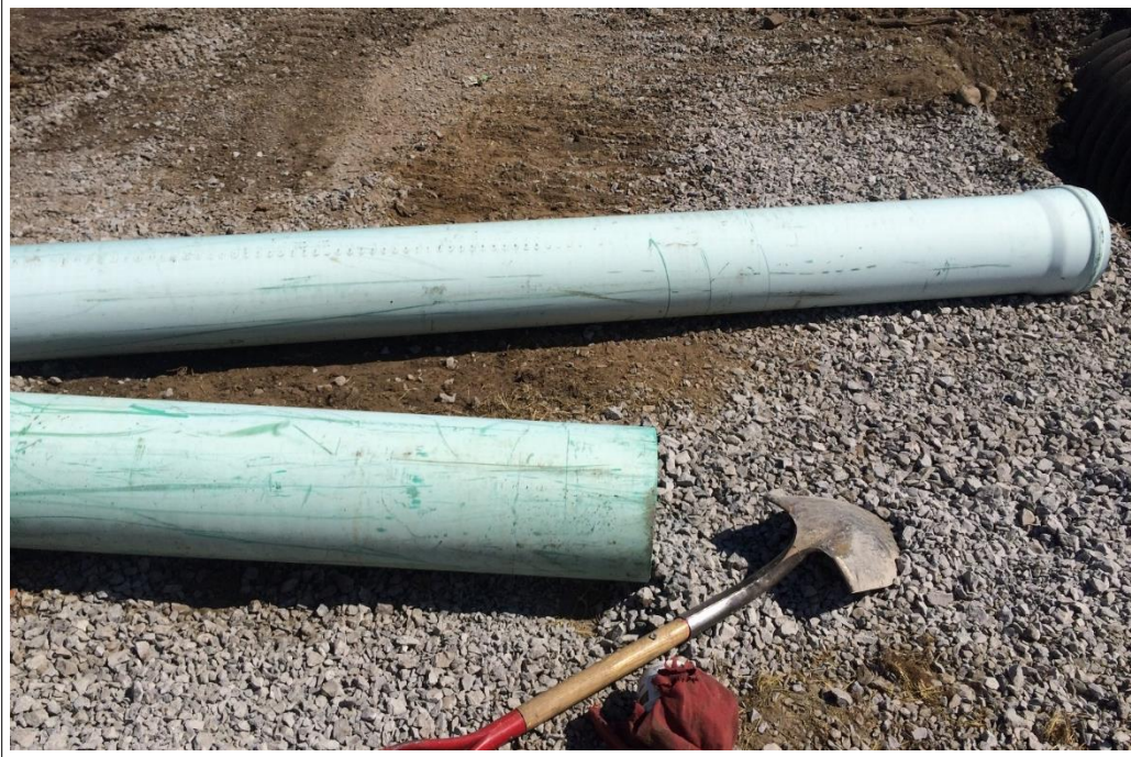
Sewer line installation
