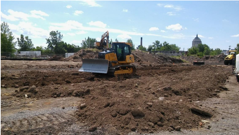
Excavation and installation of stormwater retention system on subject property.
