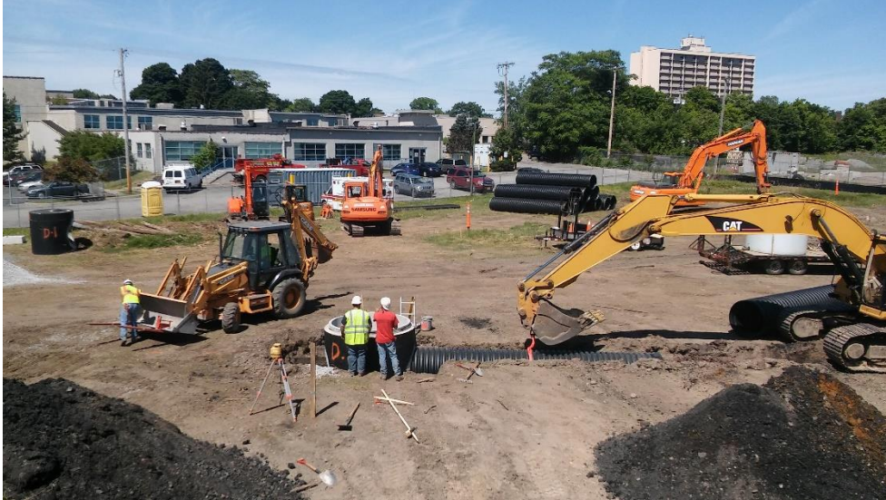
Stormwater retention system installation on subject property
