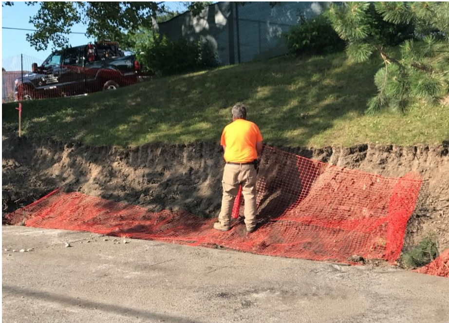
Orange plastic barrier laid on the west side of the ROW
