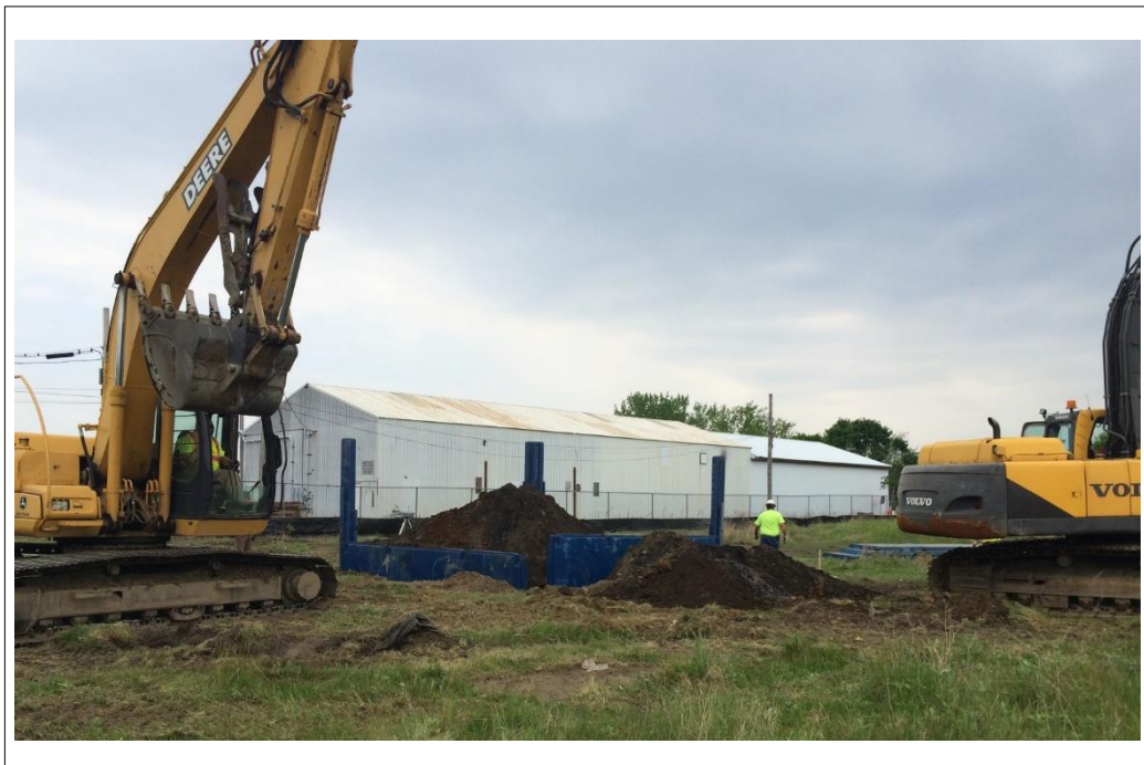
Hot Spot excavation, installation of shoring
