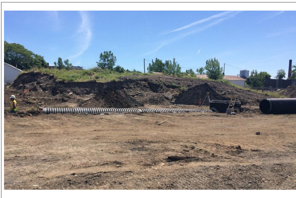
Stormwater retention system installation on subject property
