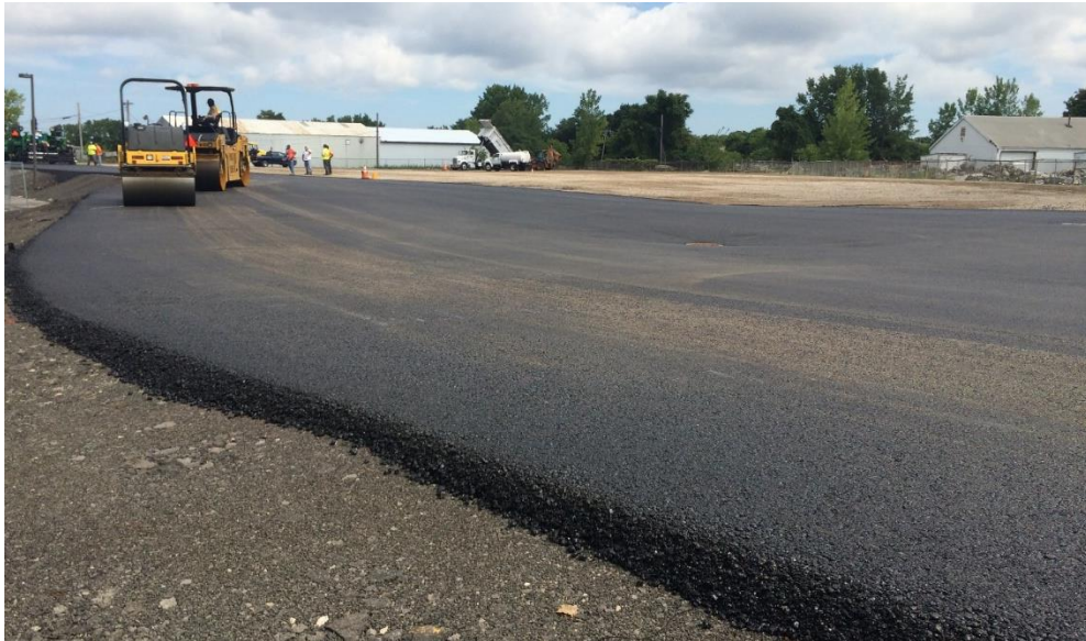
Capping of back lot with asphalt paving
