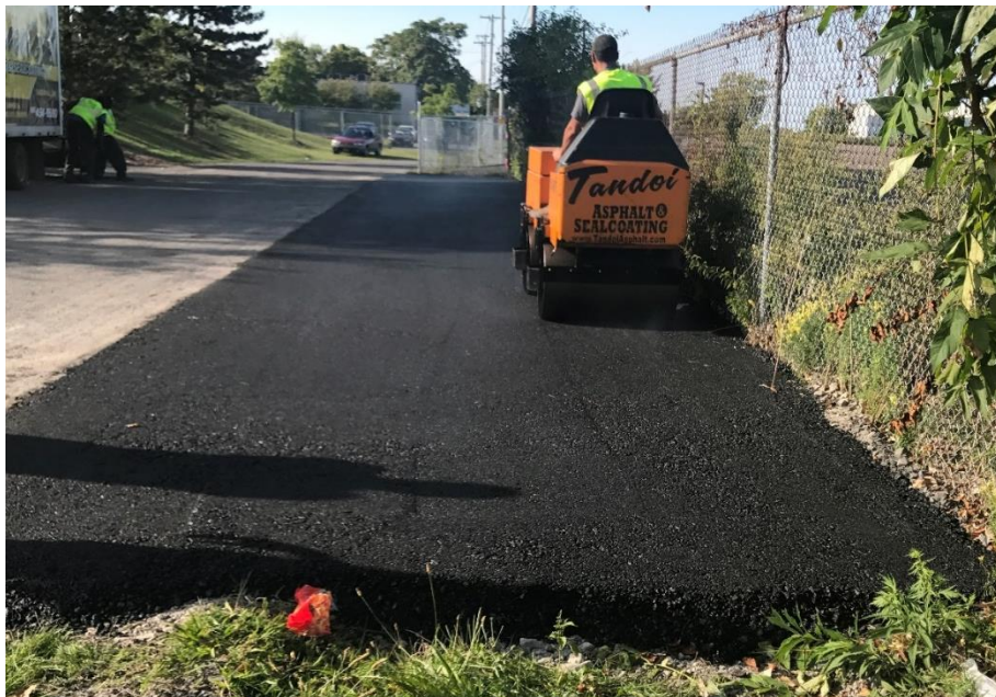
Asphalt laying on east side of Haidt Place
