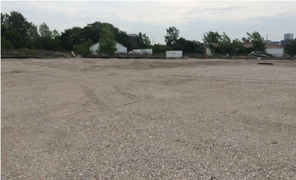
Mixed crush concrete spread out with subject property
