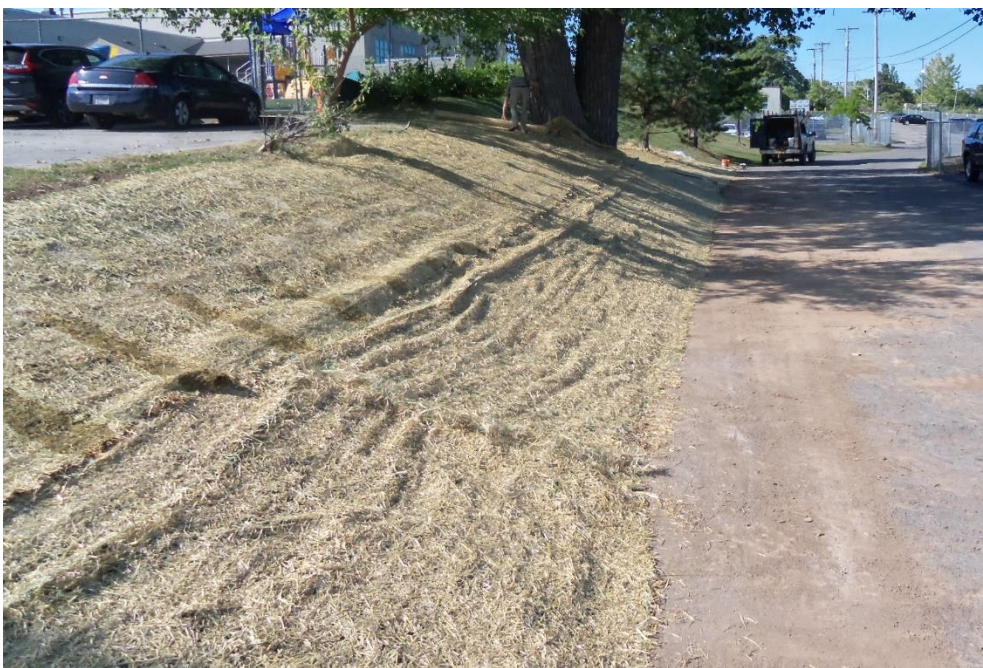
Straw erosion map used on west side of Haidt Place
