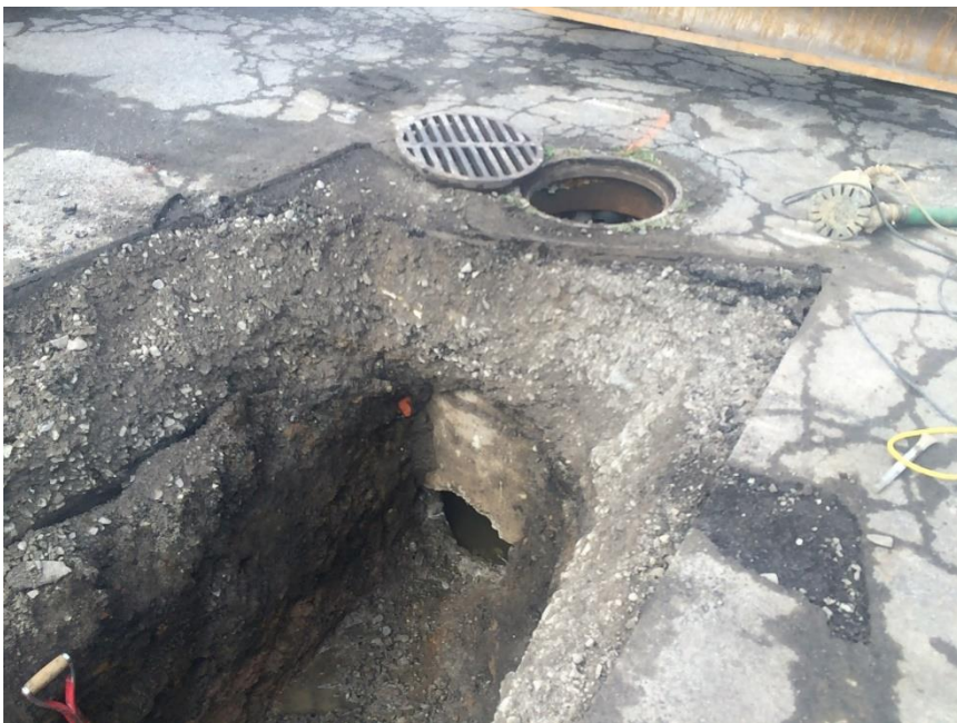
Dewatering system and sewer line installation on subject property
