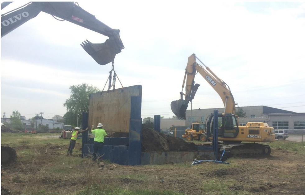
Hot Spot excavation, installation of shoring
