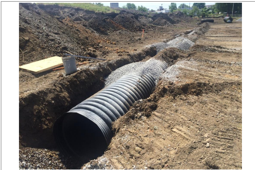
Stormwater retention system installation on subject property
