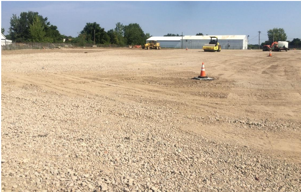
Spreading and compaction of fill material on subject property
