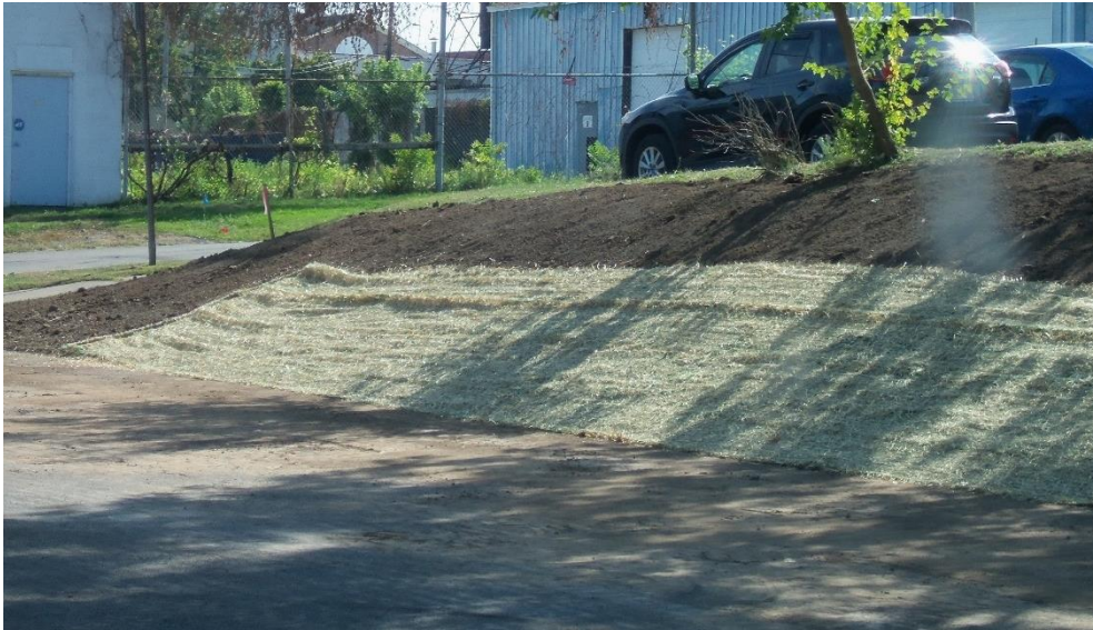
Straw erosion map used on west side of Haidt Place
