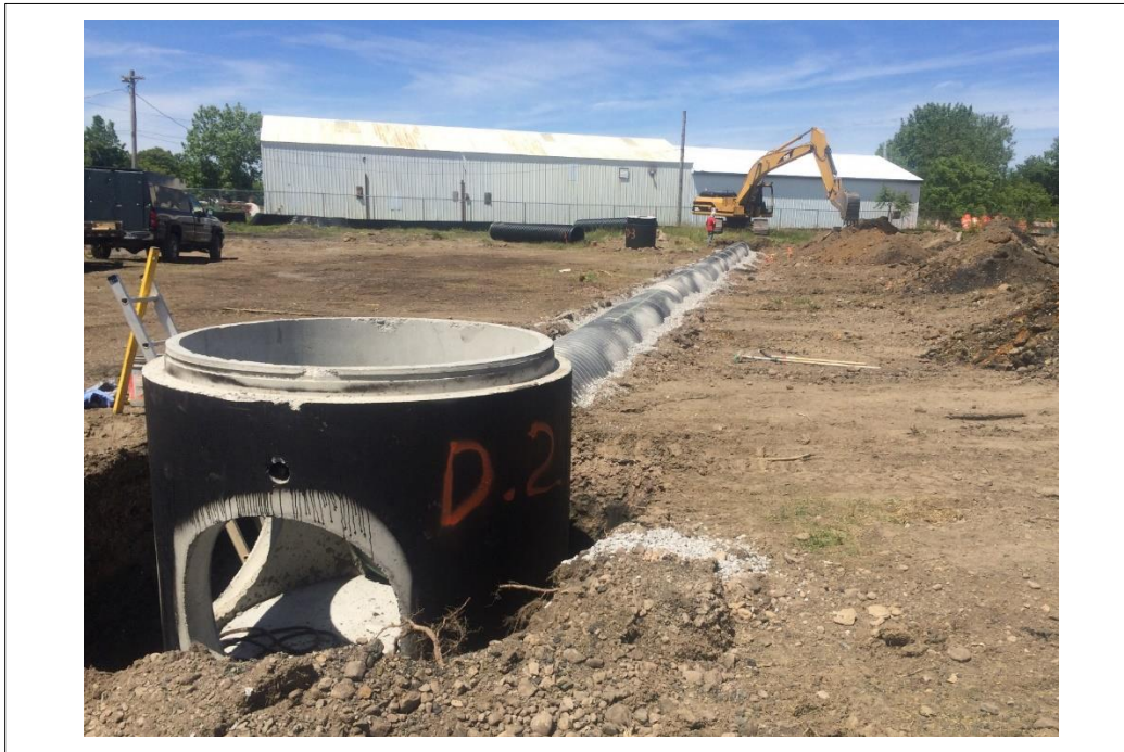
Stormwater retention system installation on subject property
