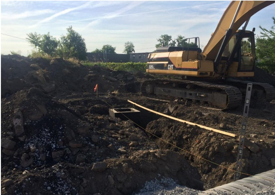
Stormwater retention and sewer line installation on subject property
