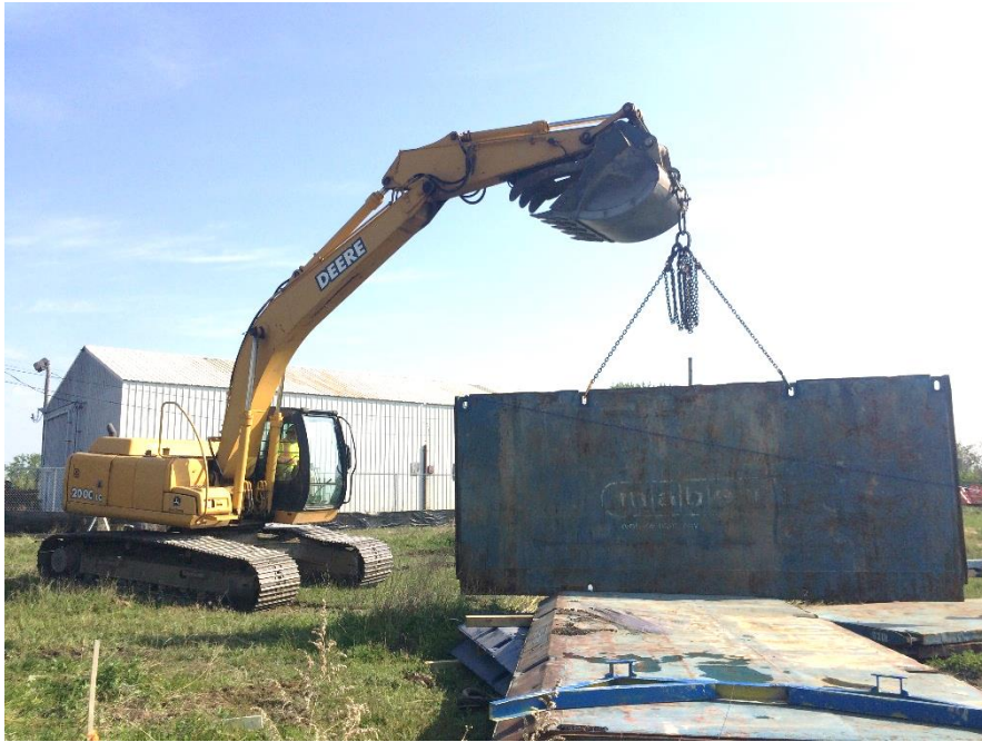
Hot Spot excavation, installation of shoring
