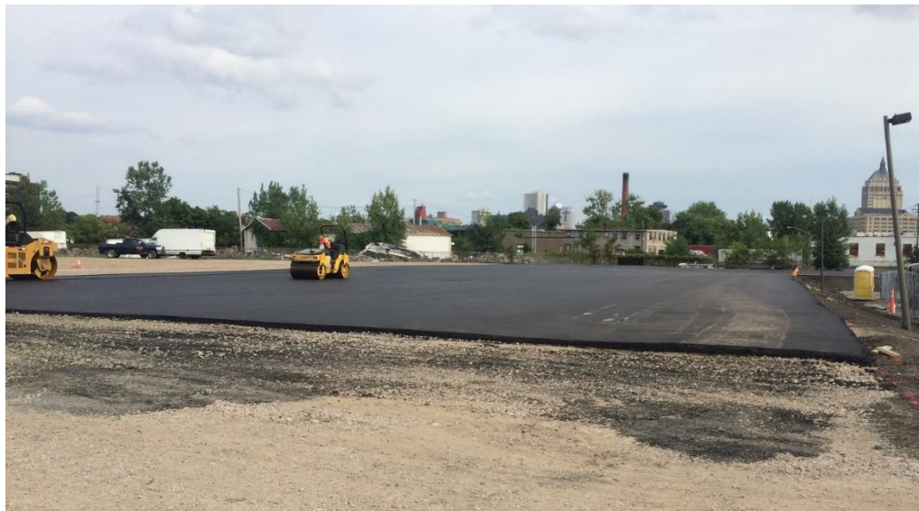
Capping of back lot with asphalt paving
