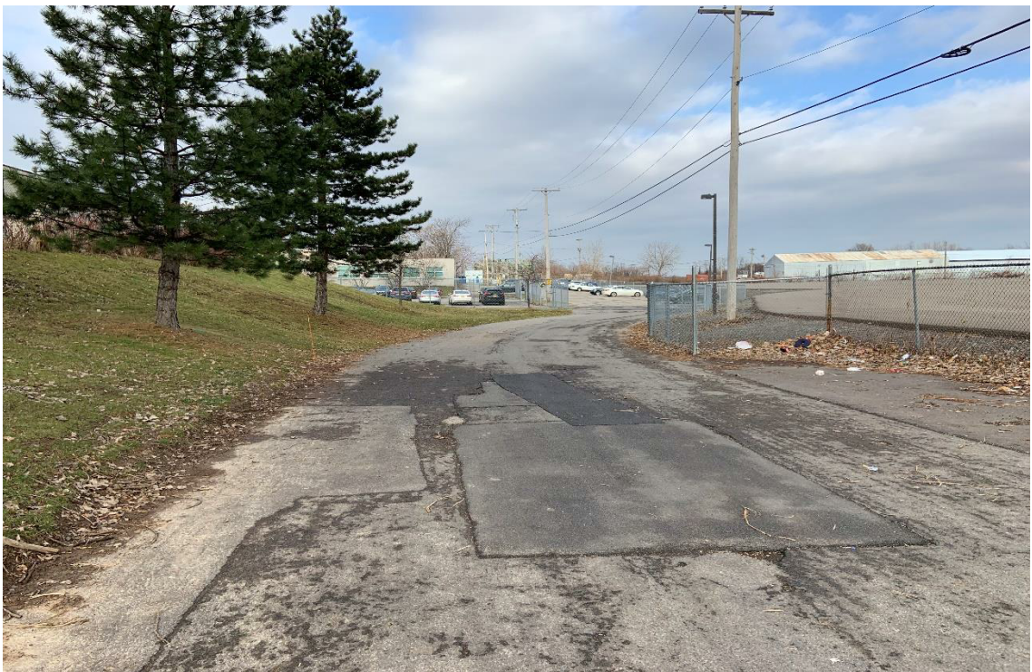
View looking north Cover Type 2, pavement patches installed in 2018 and 2019 .
