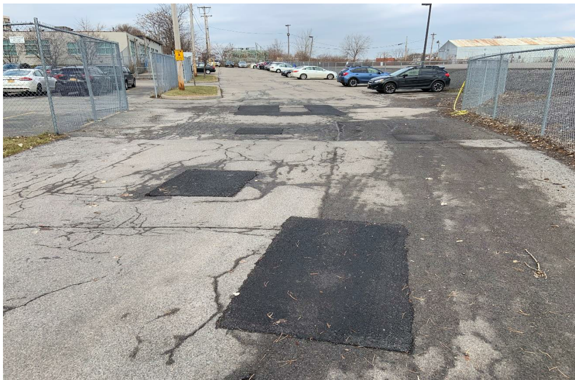
Cover Type 2, pavement patches installed in 2019.
