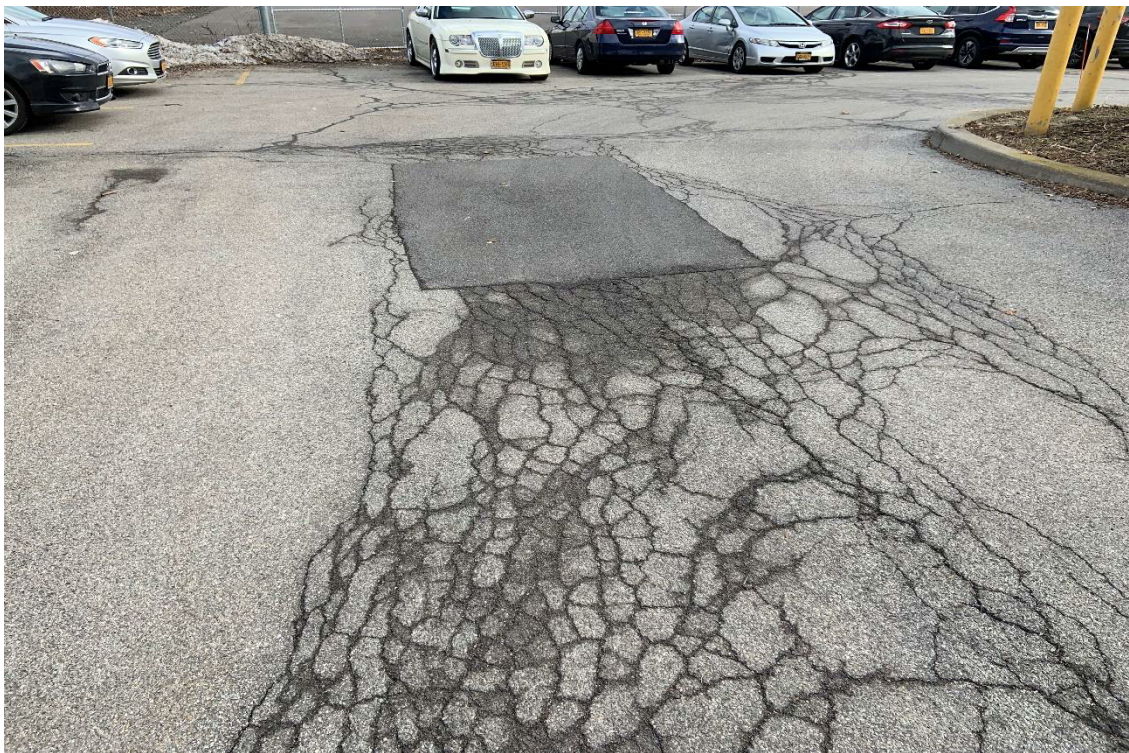
Cracked area of Cover Type 2 that requires sealer in 2020.
