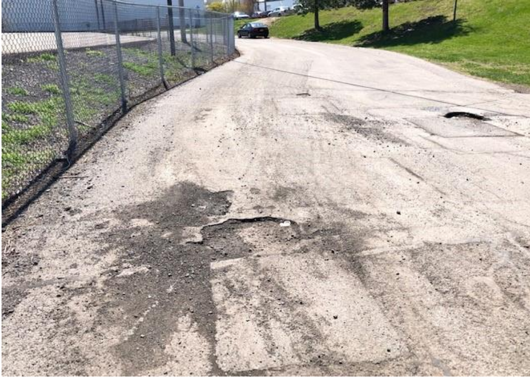
Cover Type 2, view looking south at pothole areas and patches from 2019.
