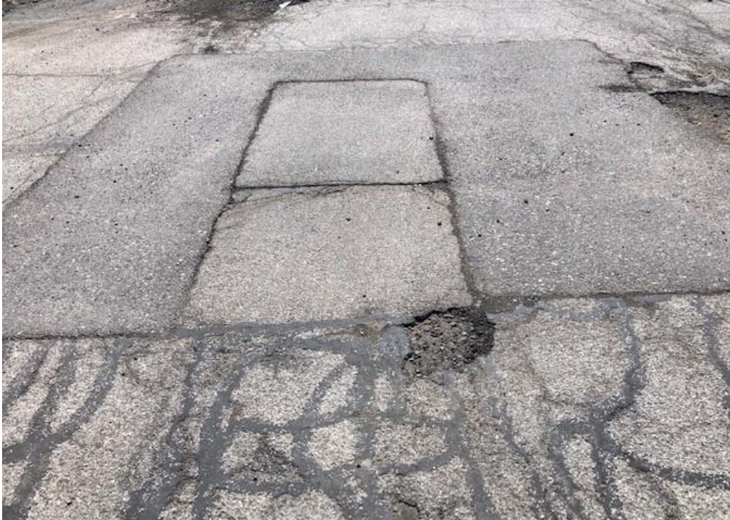
Cover Type 2, view looking south at pothole area/cracks and patched spots.
