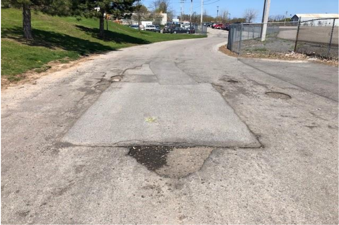
Type 2 Cover potholes and patched area from 2019.
