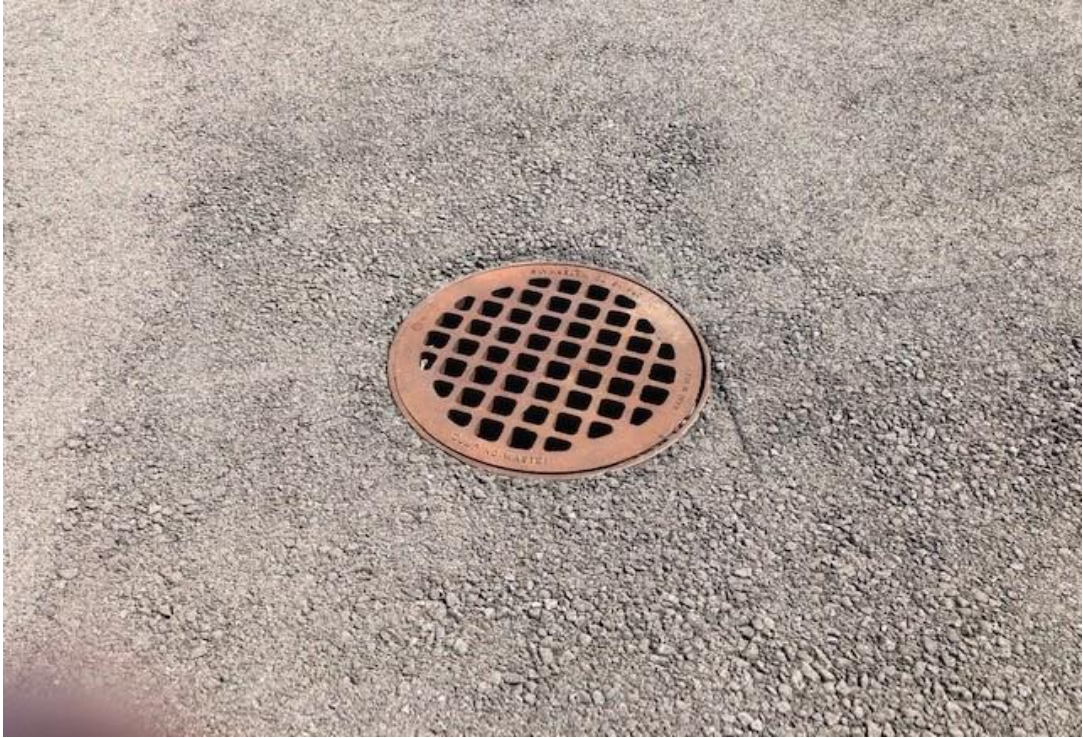
Storm manhole in Cover Type 1.
