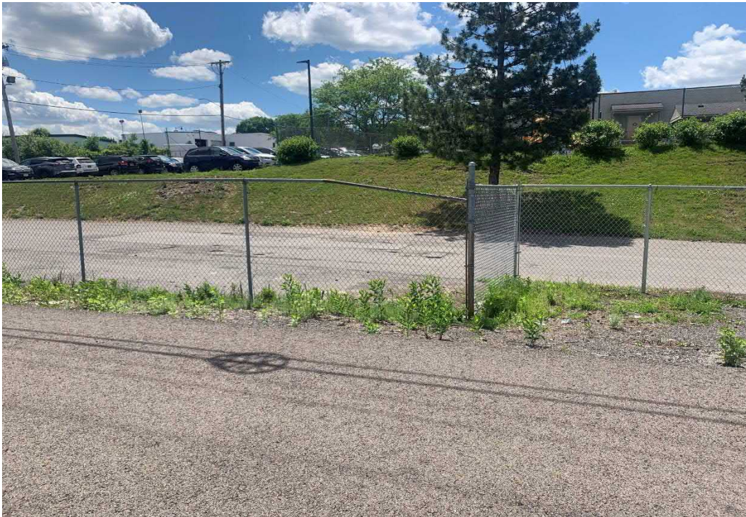
Fencing around Cover Type 1. Vegetation to be removed.
