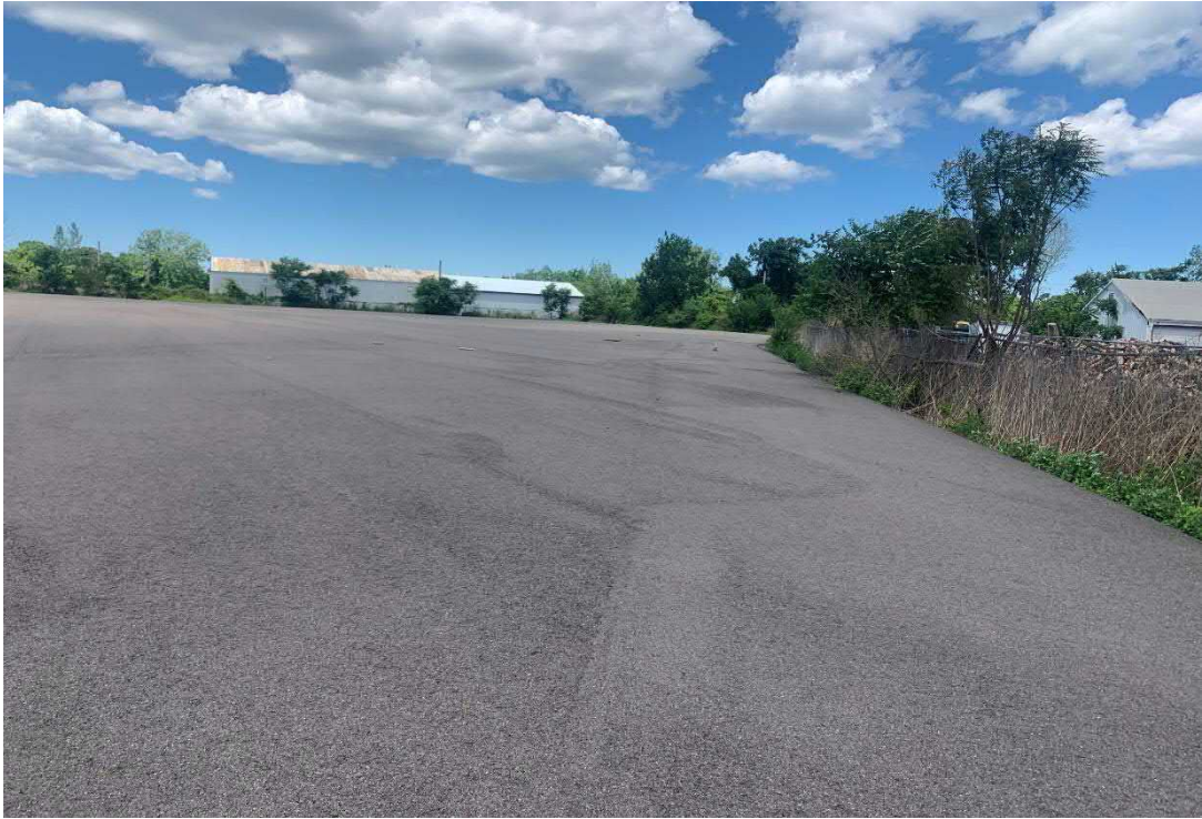
Cover Type 1, view looking north.
