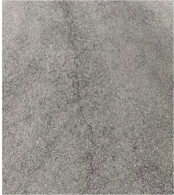
Cracks in Cover Type 1 within fenced area.
