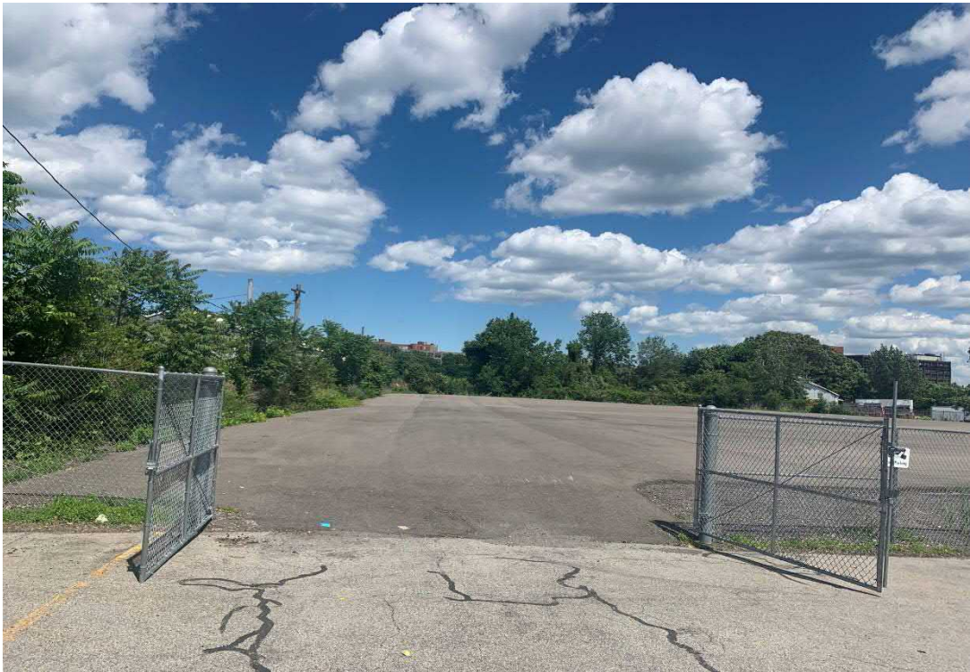
Cover Type 1, view looking east and gate.
