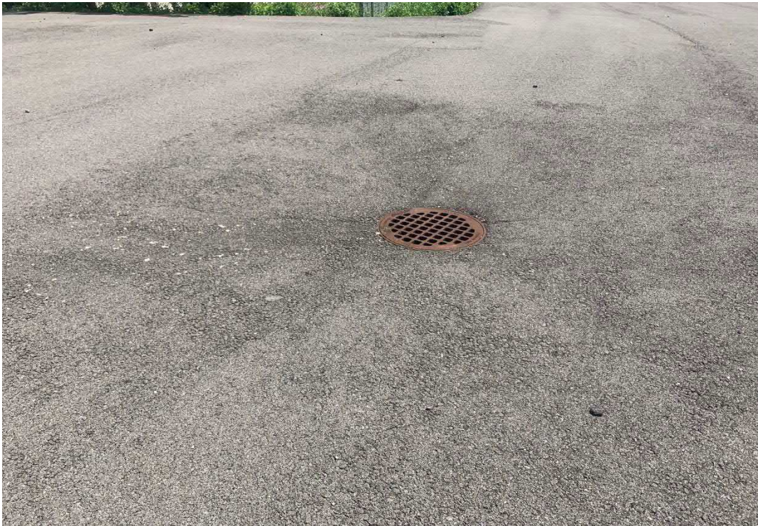
Catch basin in Cover Type 1.
