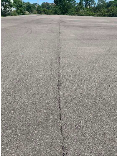
Cracks in Cover Type 1 within fenced area.
