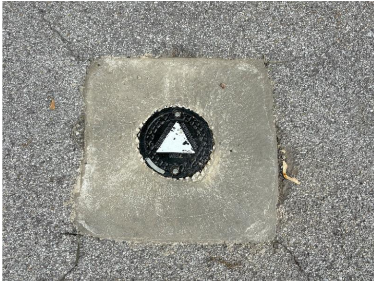
Photo 1: MW-102 has been fixed with new concrete and a new lid.
