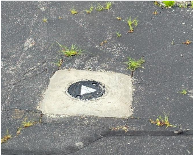
Photo 3: MW-101 has been fixed with new concrete and a new lid.
