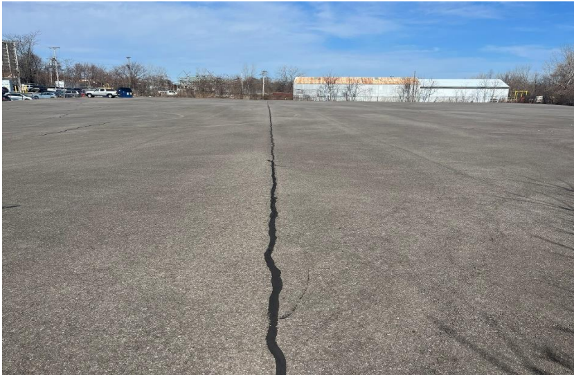
Photo 21- South side of Back Lot. Long crack has been previously sealed but has begun to come apart again.
