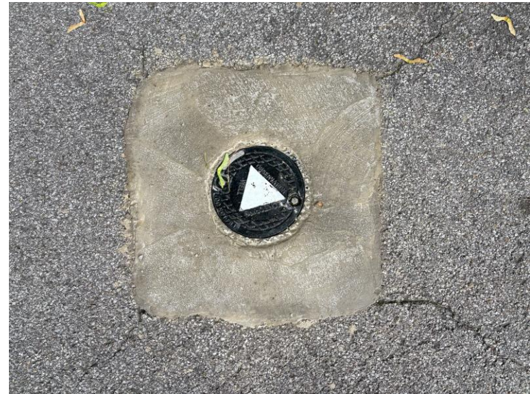
Photo 2: MWR-102 has been fixed with new concrete and a new lid.
