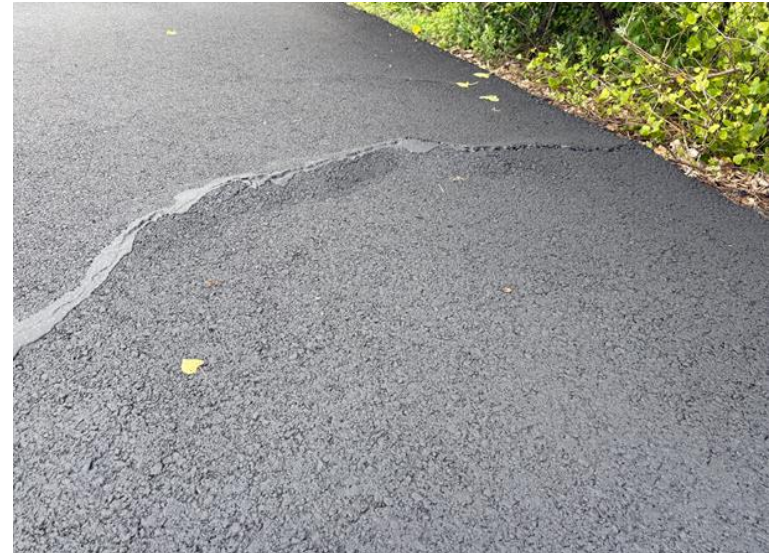
Photo 8: Close up of the crack shown in Photo 6.
