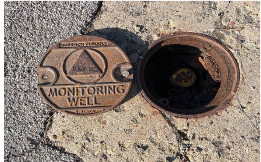
Photo 14: MWR-102: Concrete well box has some small cracks.
