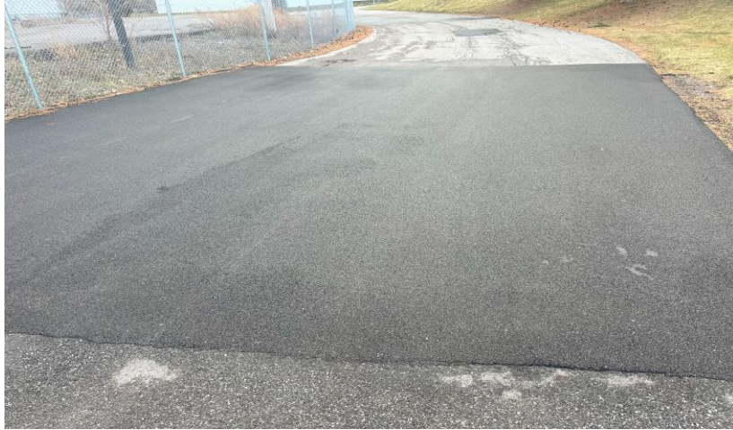
Photo 5: Type 2 Cover on Haidt Place with new pavement cover to the west side of the Site.
