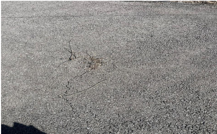
Photo 19: East side of Back Lot. Small cracks in pavement.
