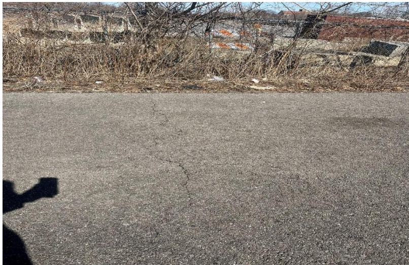
Photo 7: East side of Back Lot. Asphalt has a shallow and long crack visible.
