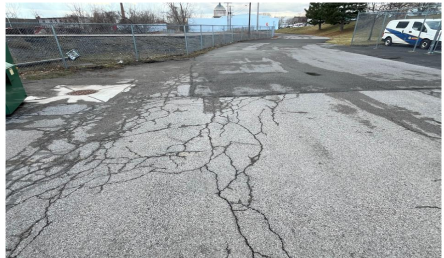
Photo 8: West side of site facing south, Refurbished drain, Haidt Place pavement covers visible. Some cracks in pavement.
