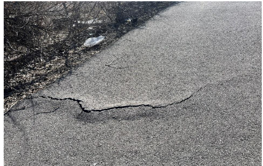
Photo 20- Northeast side of Back Lot. Tree root growing under pavement has cause a large crack to form in the asphalt.
