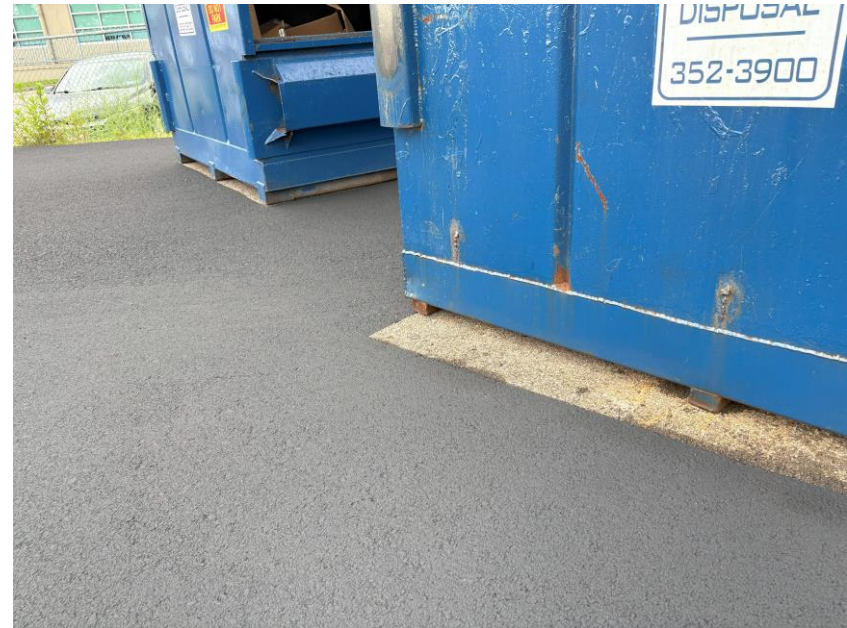
Photo 26: Asphalt under the two dumpsters near the northwest corner in the back lot was not repaved.
