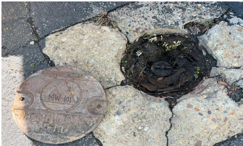
Photo 11: MW-101: Concrete well box is damaged with several large cracks. The seal has been compromised, allowing soil and vegetation into the well.
