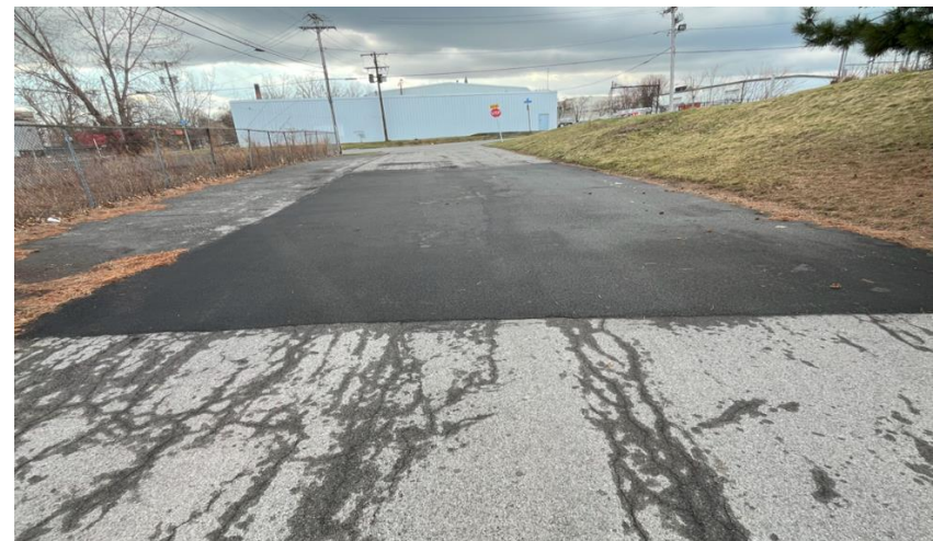
Photo 4: Type 2 Cover fully patched on west side of the Site. Facing south.
