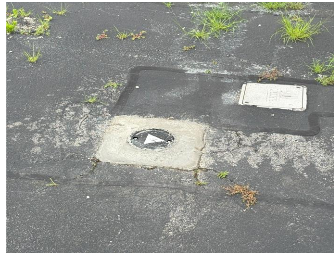
Photo 4: has been fixed with new concrete and a new lid.
