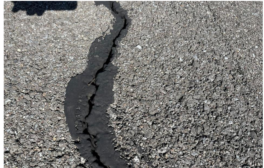
Photo 22 – Back Lot. Previously sealed pavement has started to crack again and will require to be sealed again.
