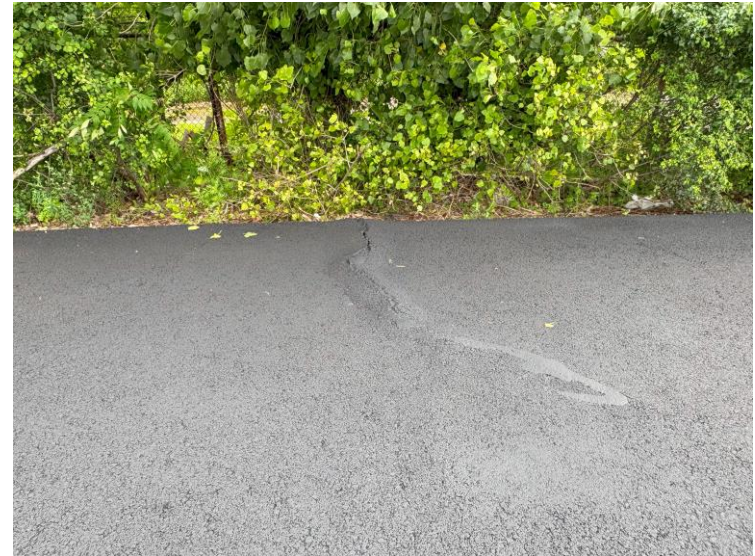
Photo 6: Crack in the pavement, likely caused by a tree root, near the northeast corner of the back lot.
