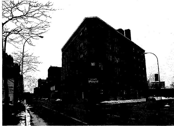
Looking west at subject Kirstein Building
