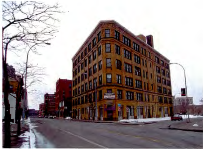
Looking west at subject Kirstein Building
