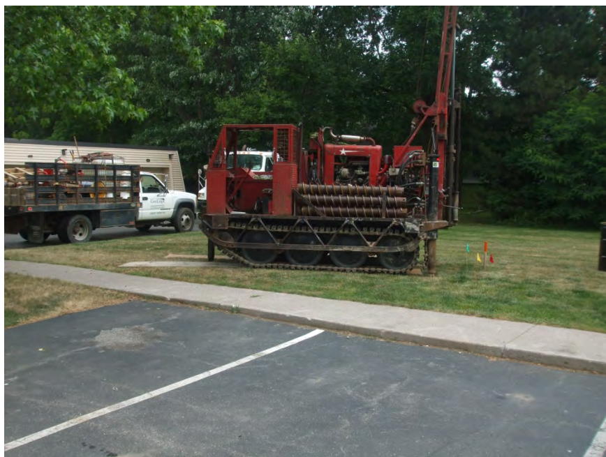
Installing monitoring well MW-11.
