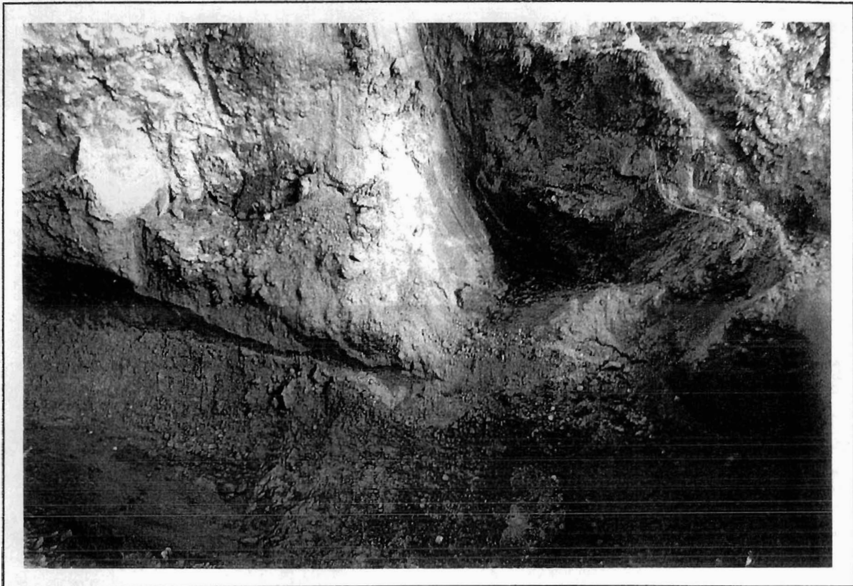
Photograph 13: Central east wall at 5-8 foot depth of eastern tank pit
