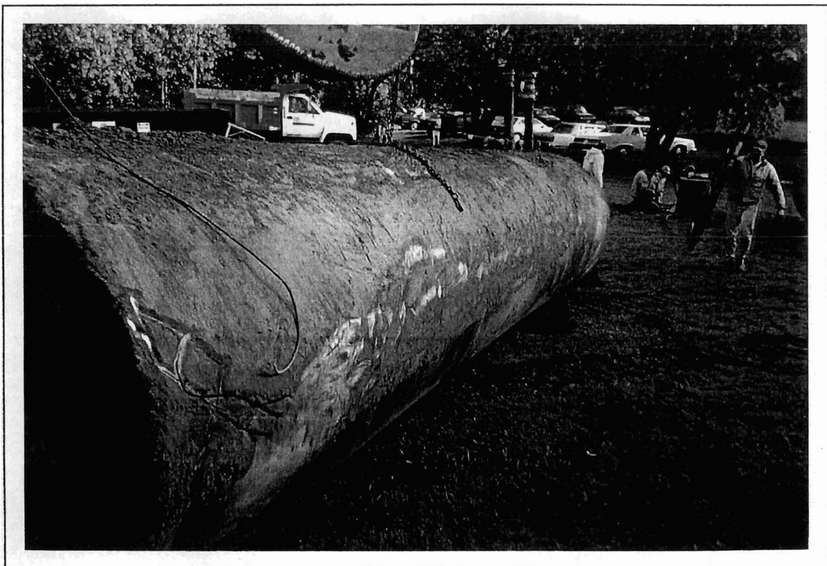
Photograph 4: Western-most 6,000-gallon UST removed from west side of station
