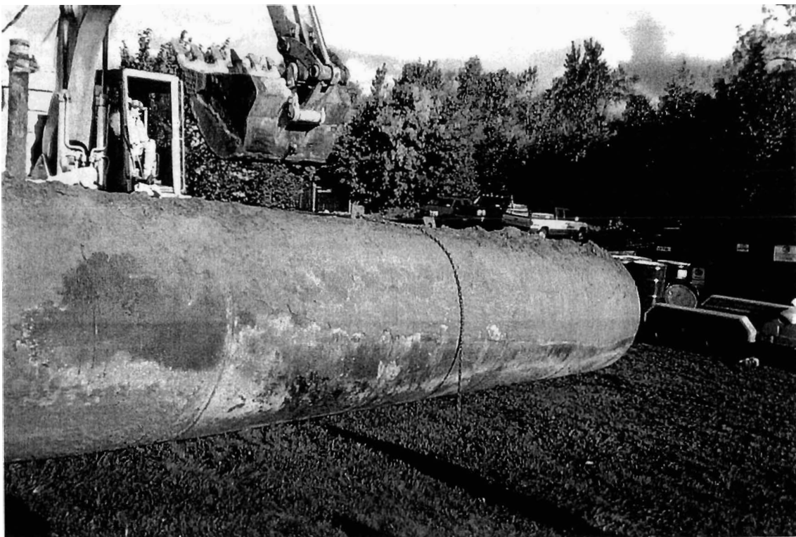
Photograph 6: Eastern-most 6,000-gallon UST removed from the west side of the station
