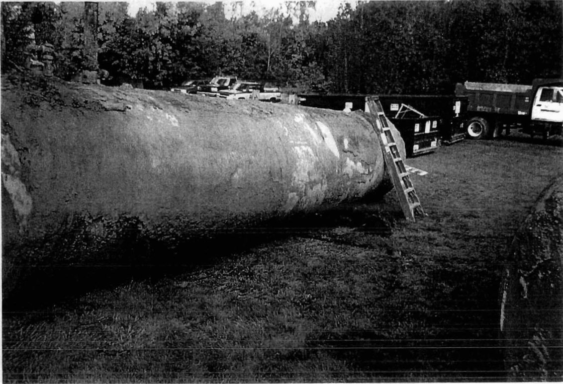
Photograph 5: Central 6,000-gallon UST removed from the west side of the station
