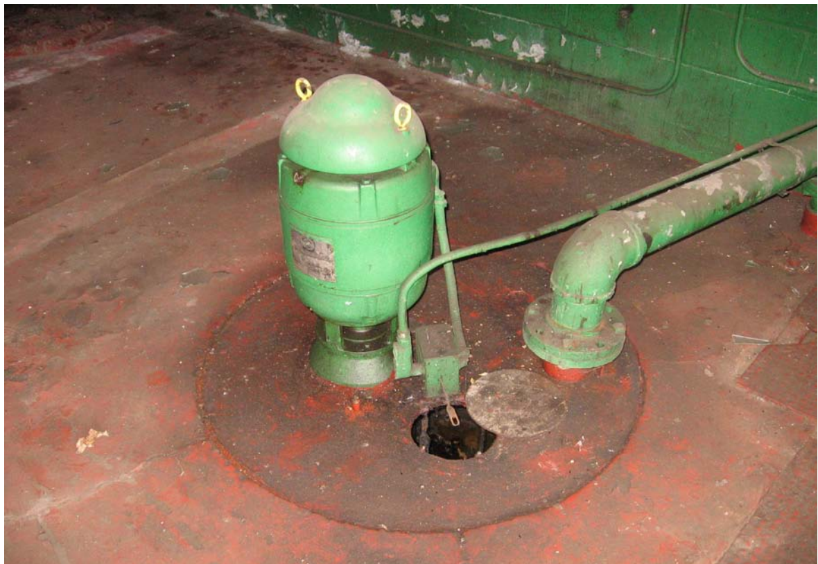
Top: Concrete sediment/oil water separator in central portion of water treatment room.
