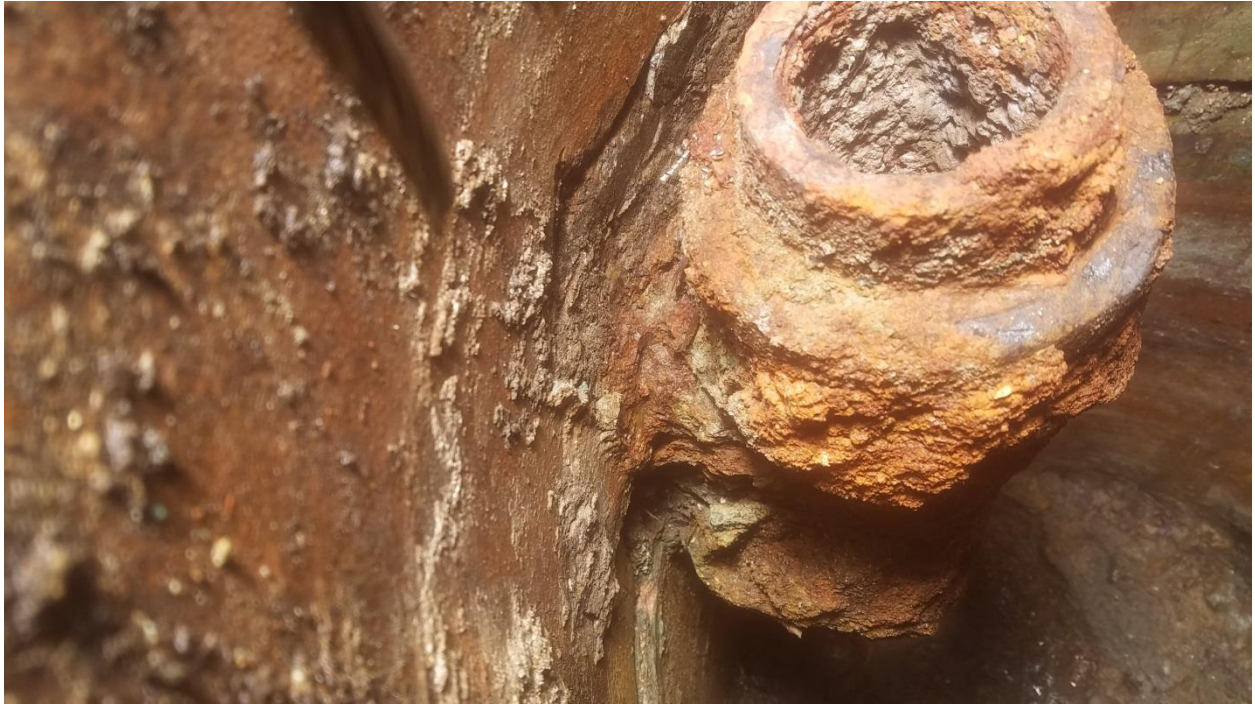
Side view of feature at northwest perimeter
