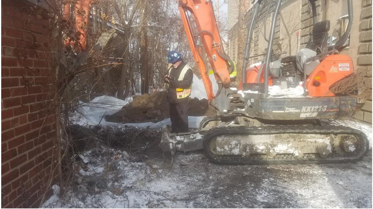
Excavation of recovery well pit
