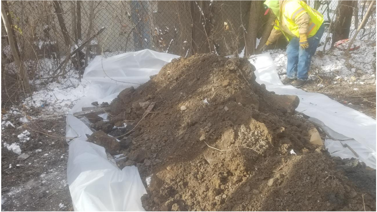
Staging of excavated soils
