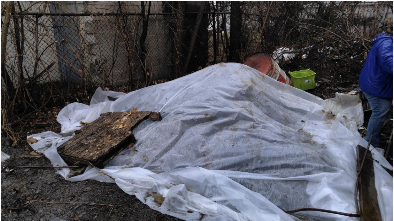
Covered excavation soils
