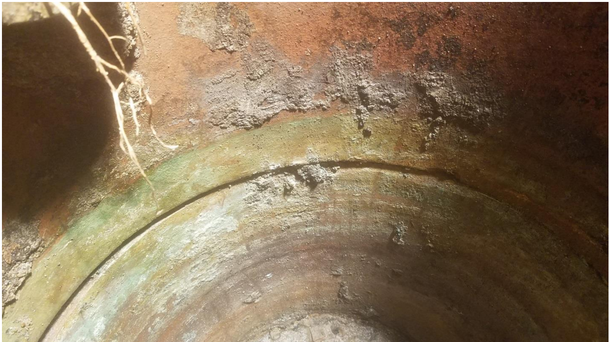
Closeup of grouted seam between two stacked concrete columns
