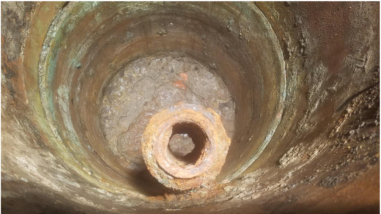
Birds eye view of feature at northwest perimeter of sump
