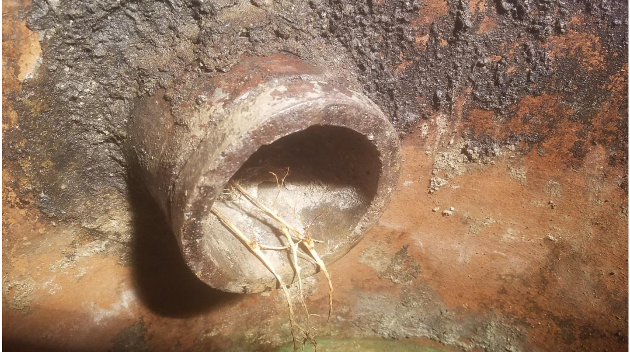
Close up of pipe at southeast perimeter of sump
