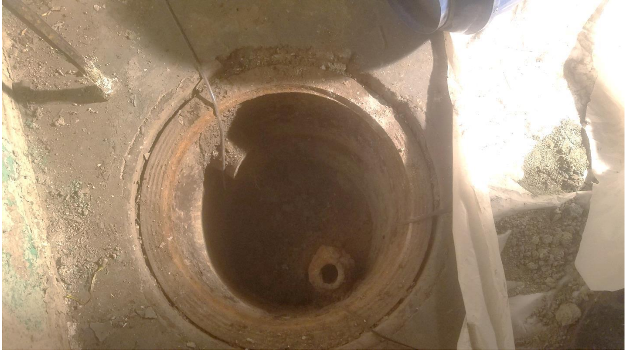
Sump prior to sediment removal
