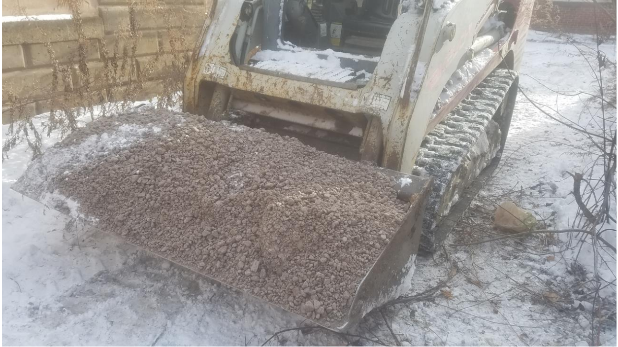
1A gravel used as recovery well backfill
