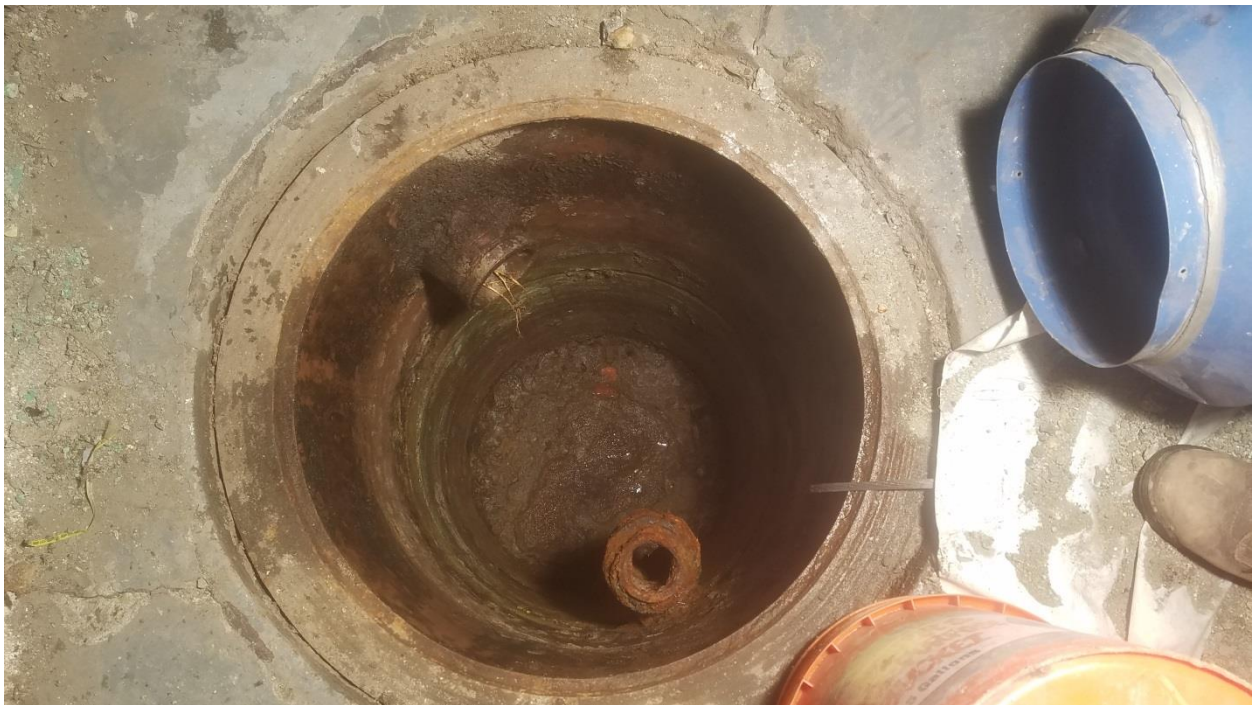
Sump after sediment removal
