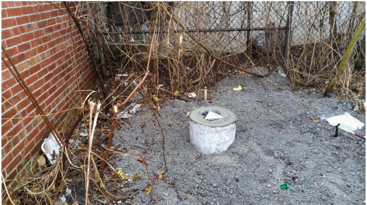
The finished recovery well
