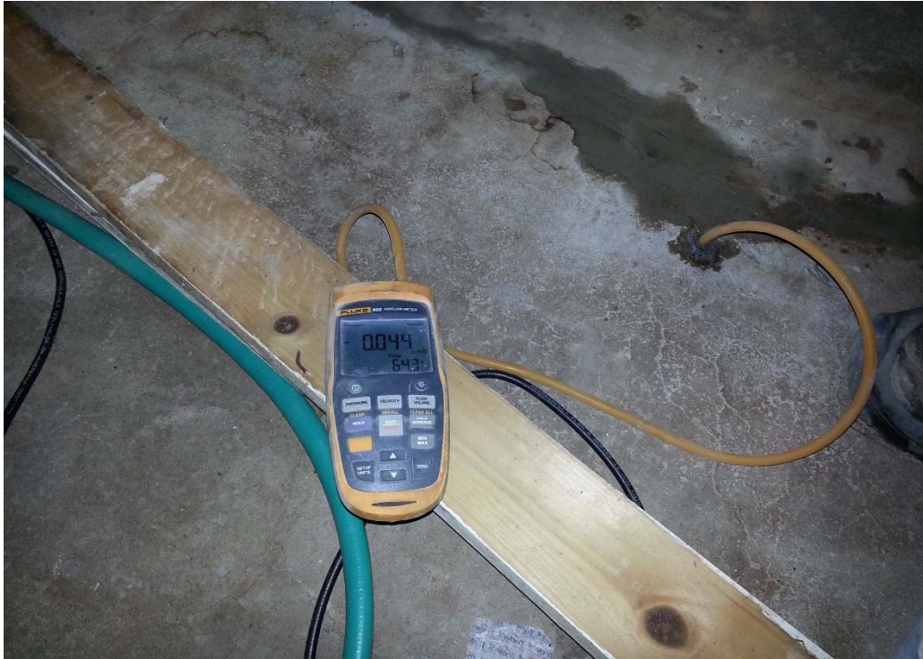
Digital micromanometer test point pressure differential measurement
