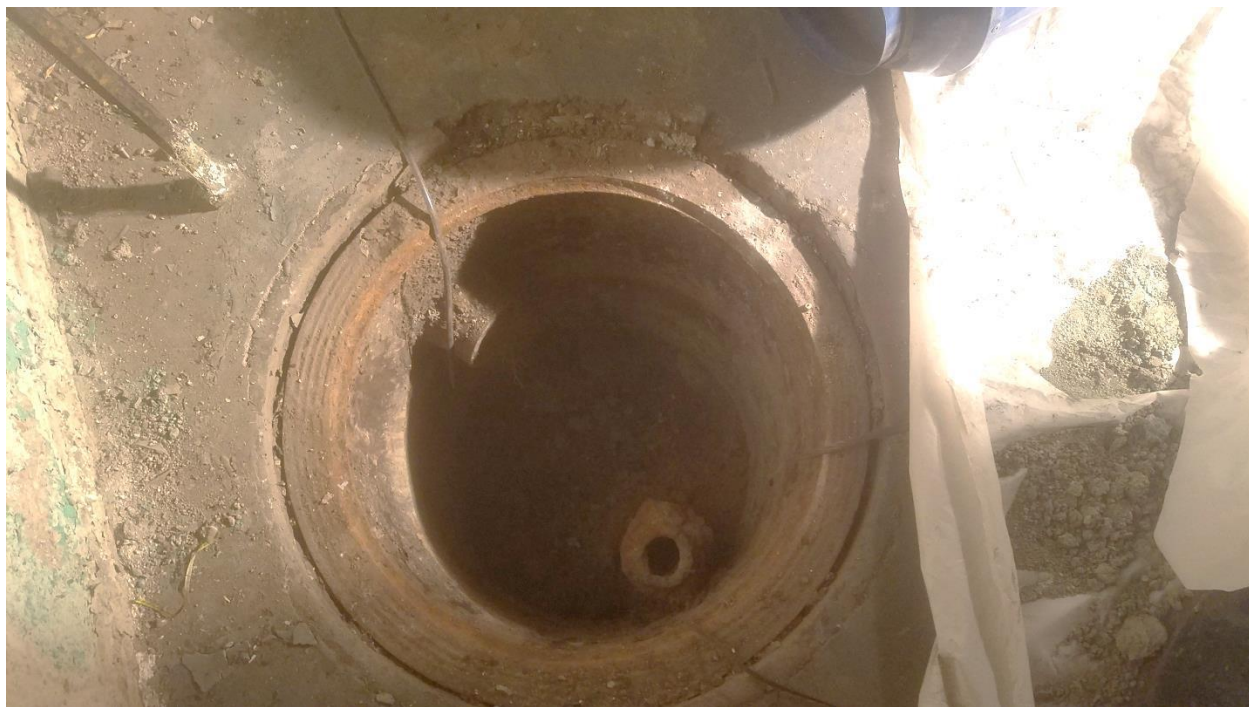
Sump prior to sediment removal
