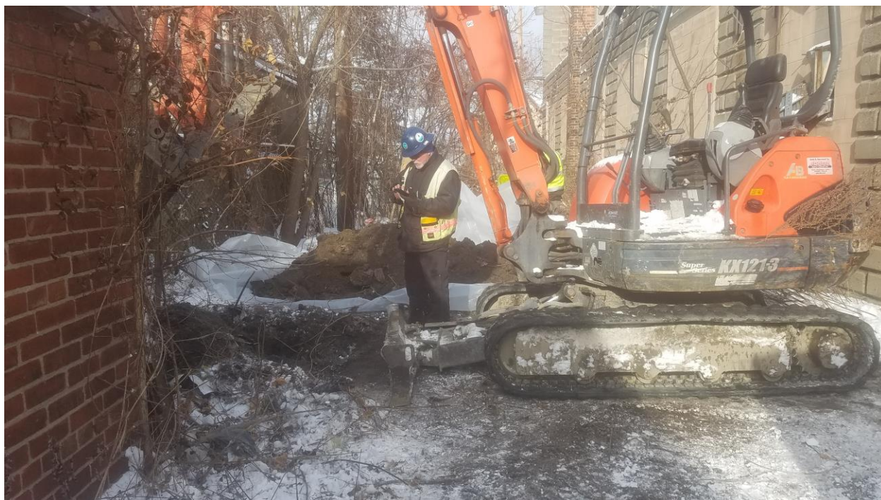
Excavation of recovery well pit
