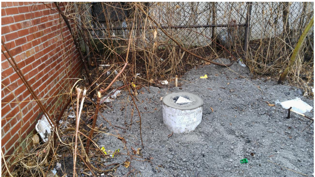
The finished recovery well
