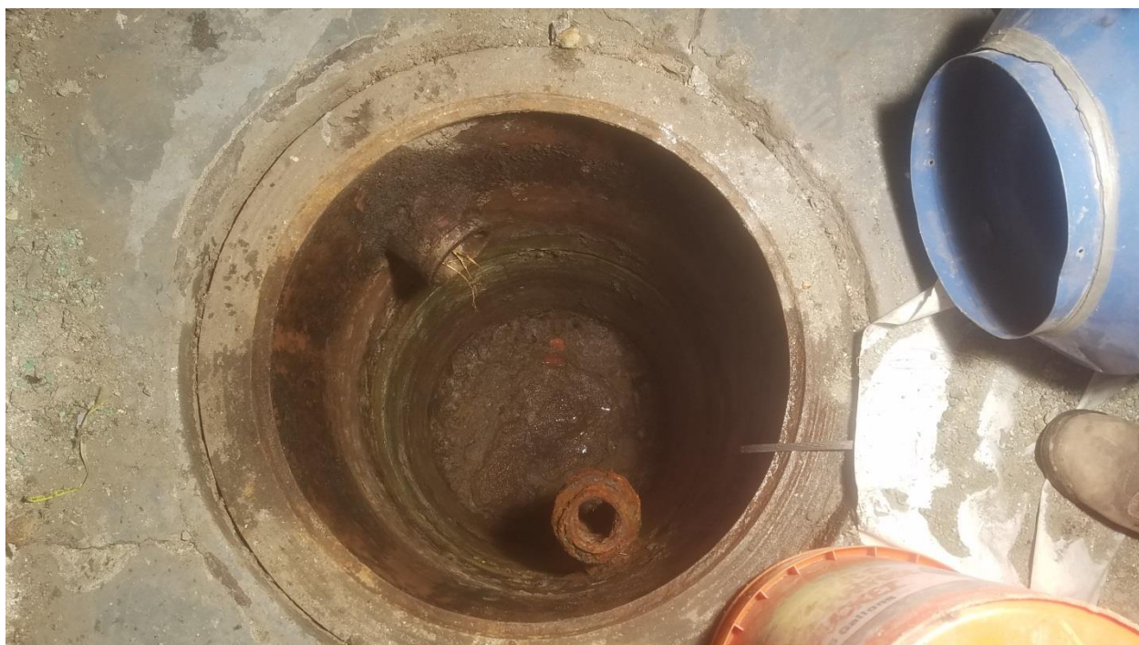
Sump after sediment removal
