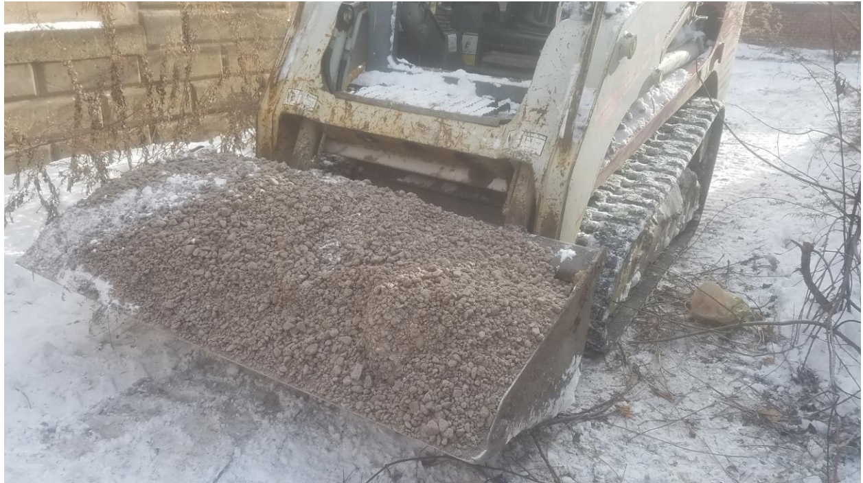
1A gravel used as recovery well backfill
