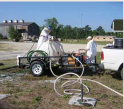
3-D Microemulsion is typically applied through permanent wells or by using direct-push injection.
