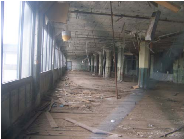
Typical view of the interior of the vacant portion of one of the buildings at the Site.
