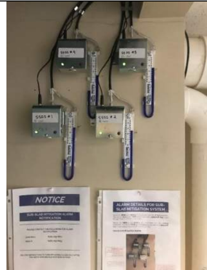
Audible alarms and manometers for SSDS
