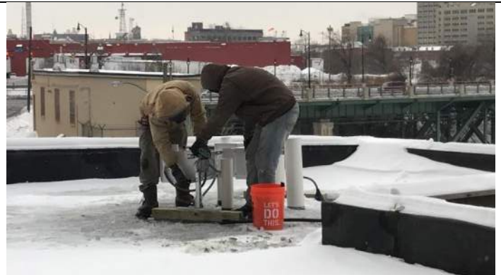
Fan installation for SSDS
