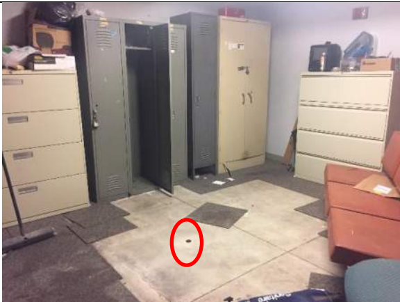
Pressure field extension monitoring point
